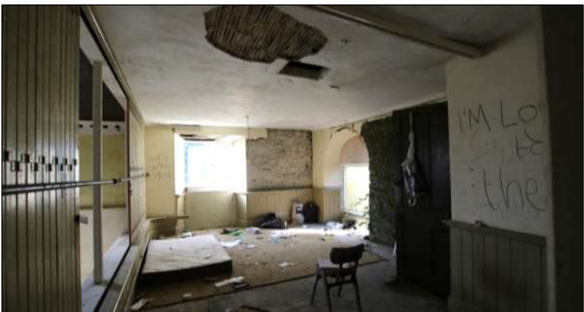
FIGURE 16: THE FIRST-FLOOR SPACE IN THE CHAPEL WITH PLANK BOARDED SLIDING SCREEN AND DADO PANNELLING; VIEWED FROM THE NNE.
