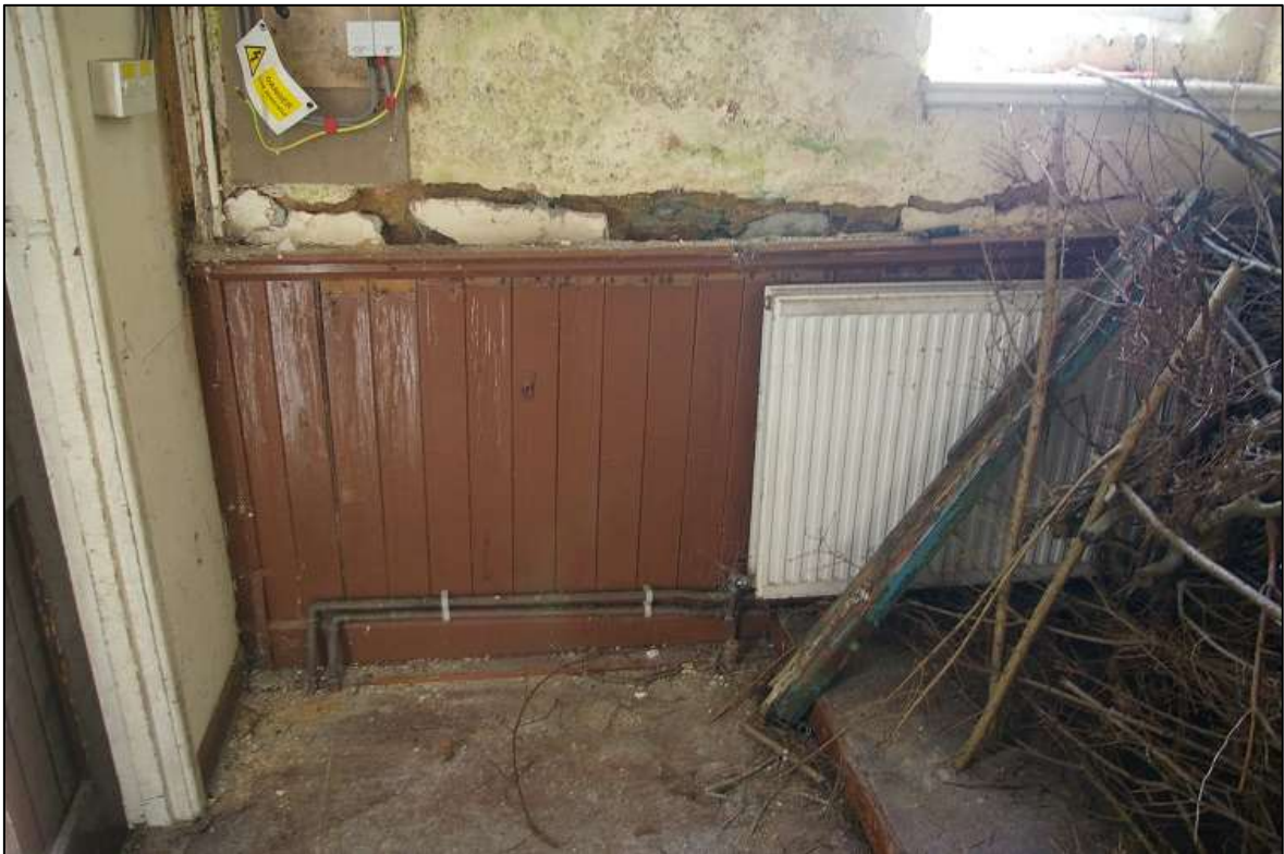
FIGURE 25: FRAGMENTARY PLANK BOARDED PANELLING ON THE EAST WALL OF THE MAIN CHAPEL HALL; VIEWED FROM THE WEST.
