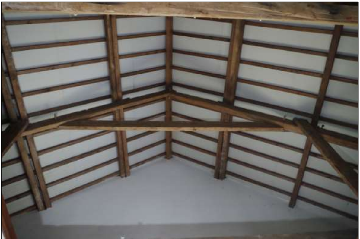
FIGURE 16: RUSTIC A-FRAMES PEGGED AND SPIKED REPRESENT GOOD INDUSTRIAL FORM AND CHARACTER. TAKEN FROM BELOW IN TO NORTH END OF R3.
