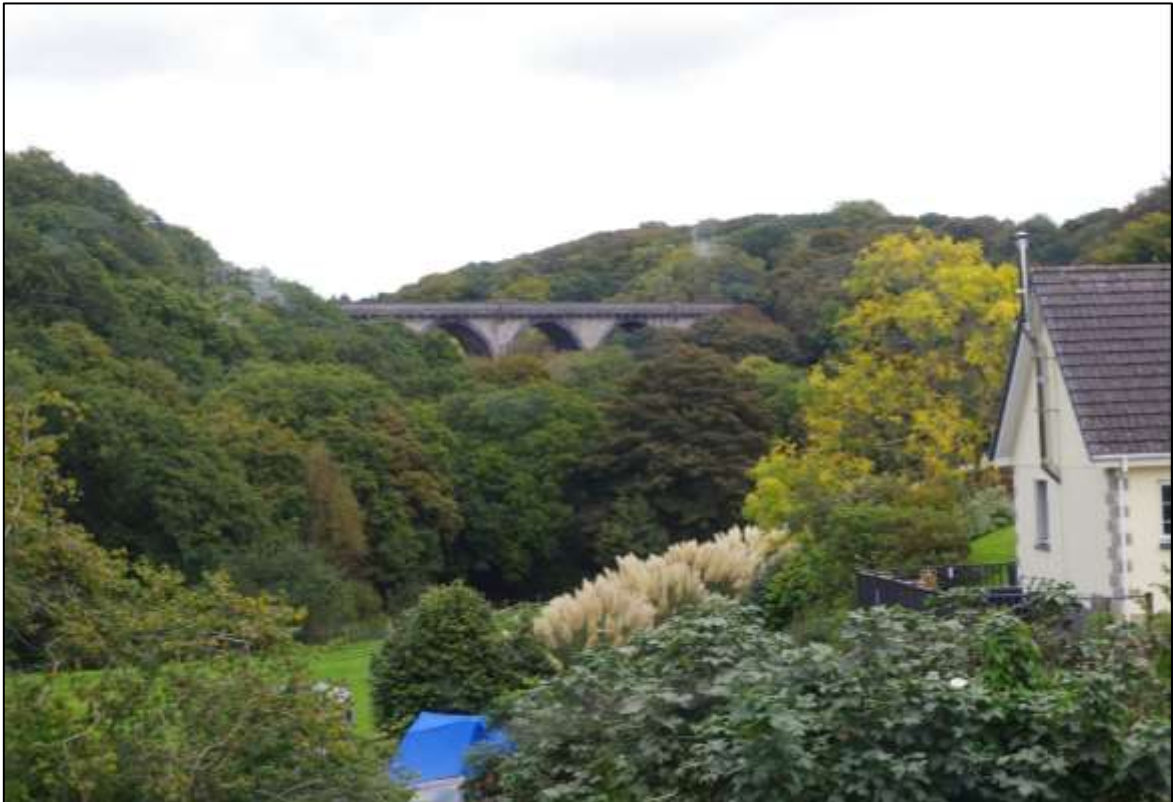
FIGURE 9: VIEWS ACROSS TO THE 19 TH CENTURY VIADUCT, TAKEN FROM THE FIRST FLOOR, FROM THE WEST.
