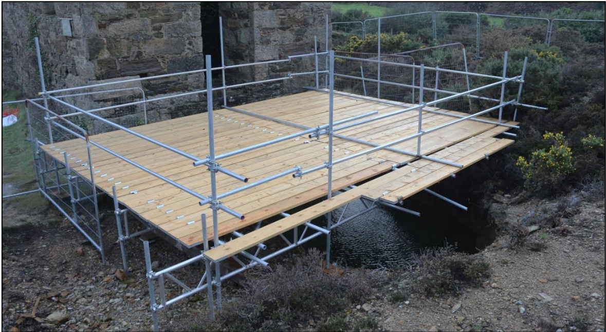
FIGURE 11: THE UNCAPPED SHAFT IN FRONT OF THE BOB WALL, WITH SCAFFOLDING COVERING IT; VIEWED FROM THE WEST (NO SCALE). THE HIGH WATER TABLE IN THE WINTER IS EVIDENT.
