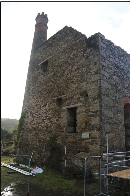
FIGURE 8: THE ENGINE HOUSE AND ITS IMMEDIATE SETTING; VIEWED FROM THE NORTH.
