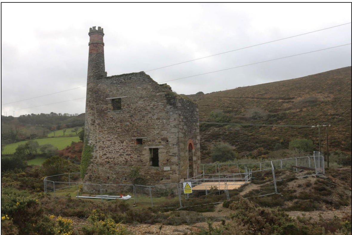
FIGURE 5: THE NORTH-EAST ELEVATION; FROM THE EAST-NORTH-EAST (NO SCALE).
