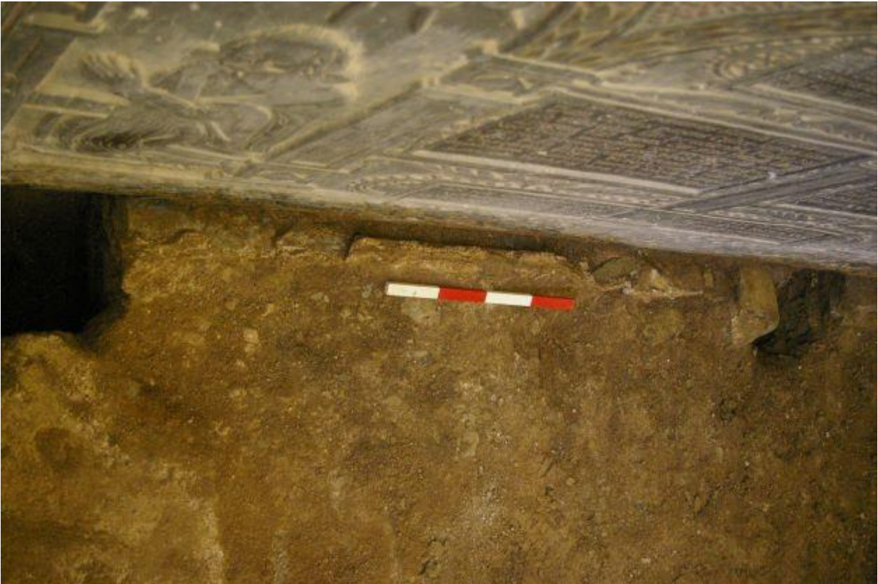
19. LIME PLASTER LIP UP AGAINST THE VERMAN MEMORIAL; VIEWED FROM THE NORTH (0.4M SCALE).
