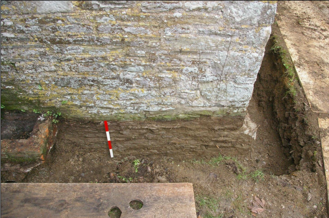
5. THE FOOTINGS OF THE WEST WALL OF THE SOUTH TRANSEPT; VIEWED FROM THE WEST (0.4M SCALE).
