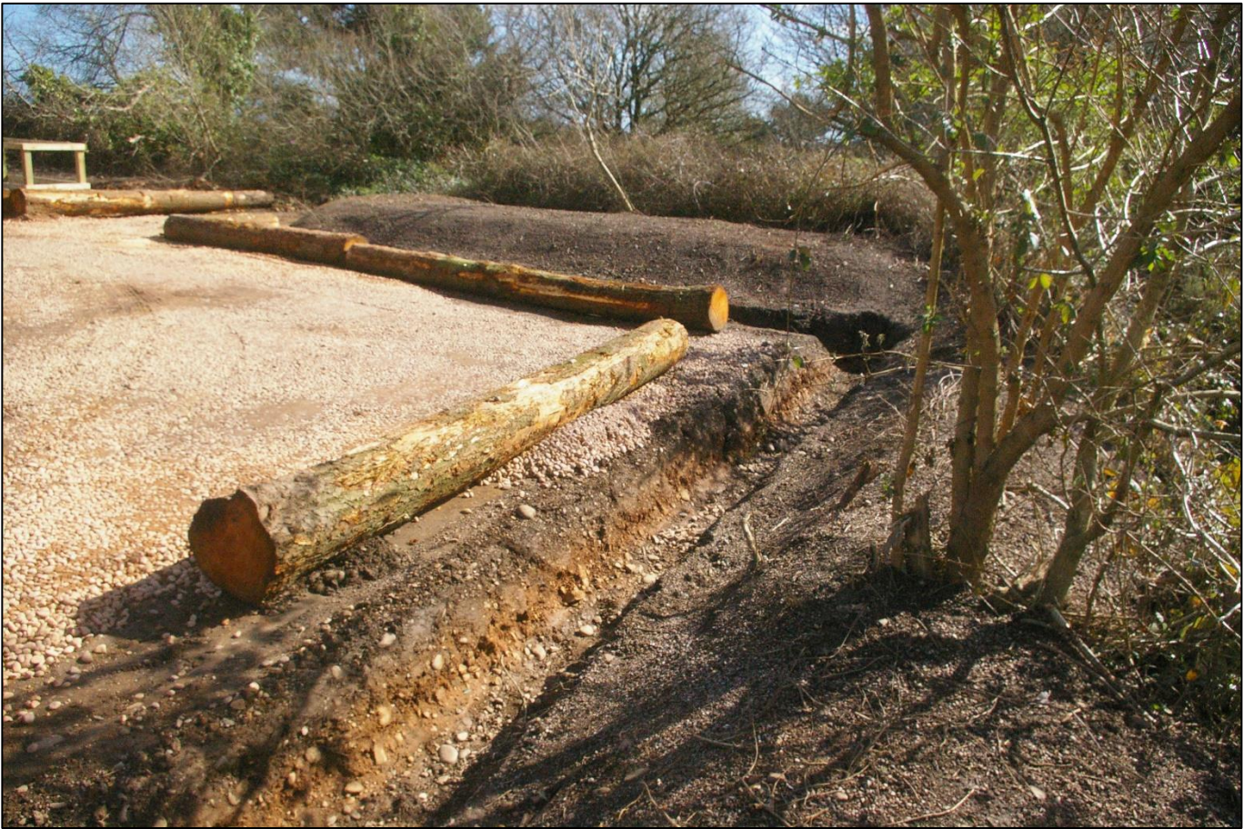
FIGURE 2: TYPICAL SAMPLE SECTION, SHOWING THE TOPSOIL, BELOW NEW CARPARK SURFACE EXPOSED WITHIN DRAINAGE DITCHES, VIEWED FROM THE NORTH-WEST. (NO SCALE).
