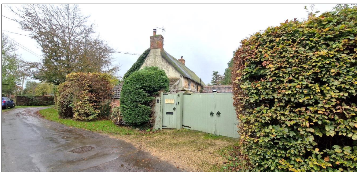
FIGURE 29: THATCHWELL ('OLD LEGGS FARM'); VIEWED FROM THE NORTH, LOOKING SOUTH.
