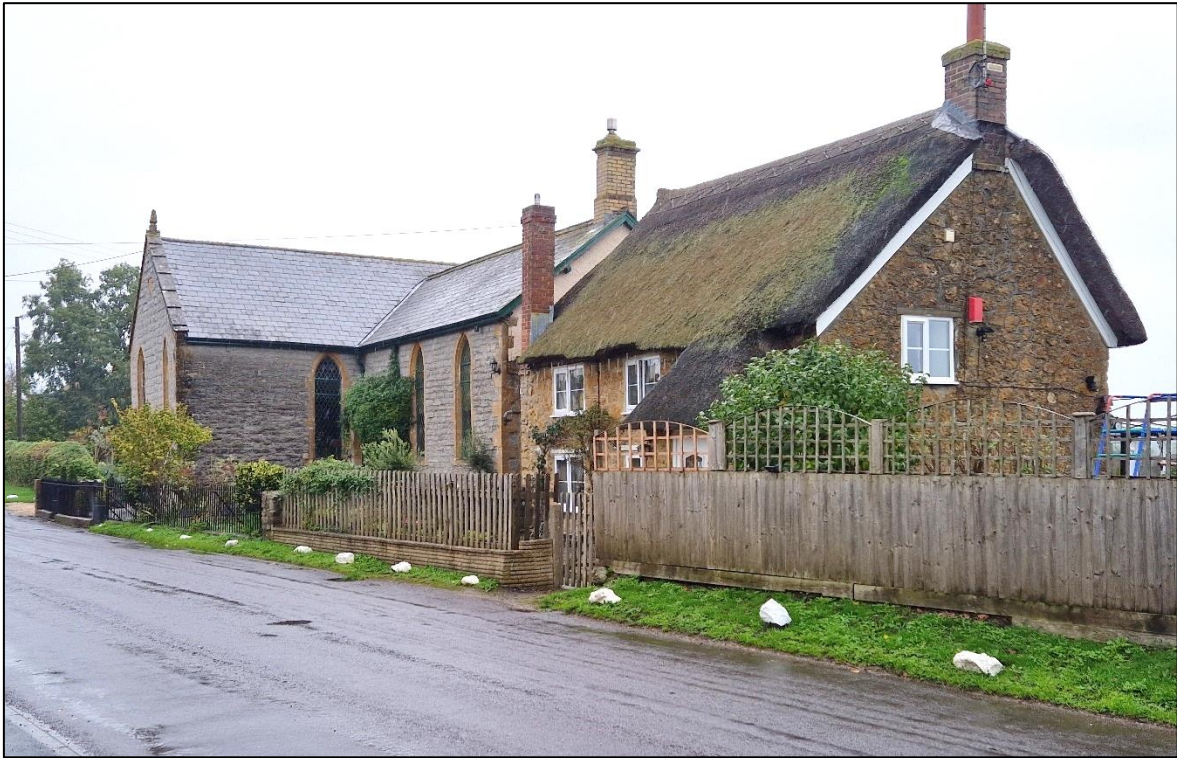
FIGURE 21: THE FORMER CHAPEL AND ADJOINING COTTAGE; VIEWED FROM THE SOUTH-WEST, LOOKING NORTH-EAST.
