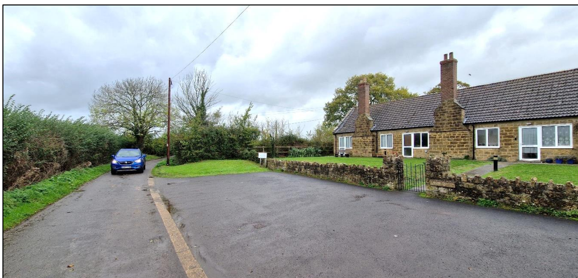
FIGURE 25: THE WADHAM ALMSHOUSES; VIEWED FROM THE SOUTH-EAST, LOOKING NORTH-WEST.
