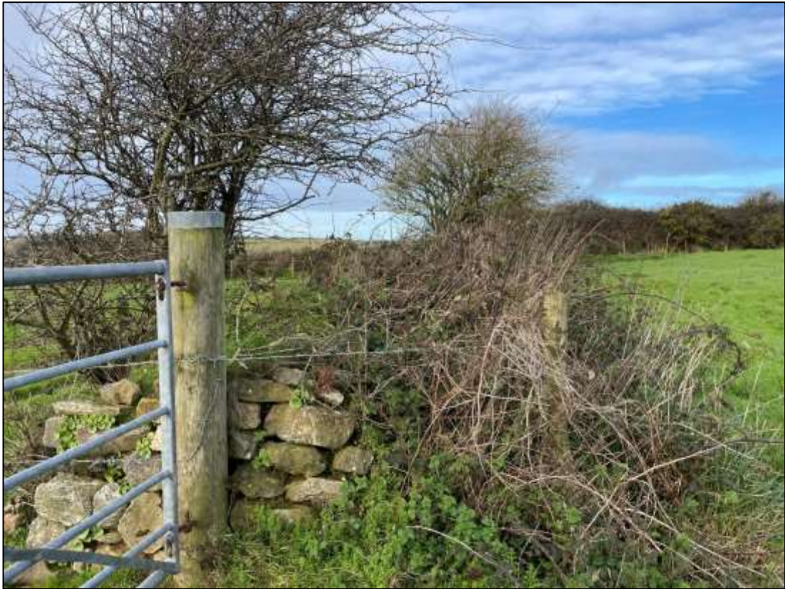
11. F2, DETAIL OF THE STONE FACED HEDGEBANK BOUNDARY BETWEEN FIELDS F1 AND F2; VIEWED FROM THE SOUTH-EAST (NO SCALE).
