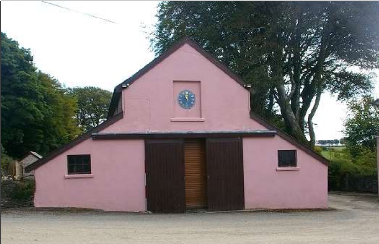
28. THE WEST ELEVATION OF THE GREAT BARN AT HONEYMEAD.
