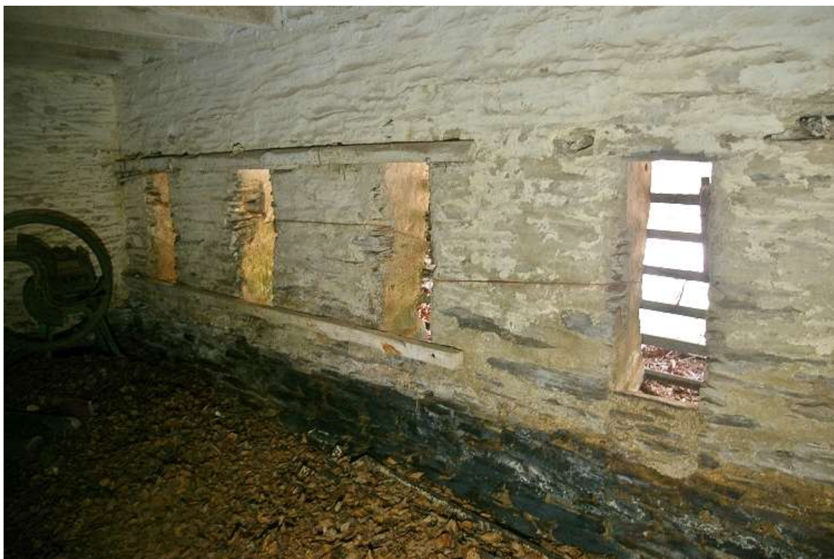
FIGURE 19: THE FEED SLOTS BETWEEN THE MAIN RANGE AND THE AISLES, WITHIN ROOM A; FROM THE SOUTH-EAST.
