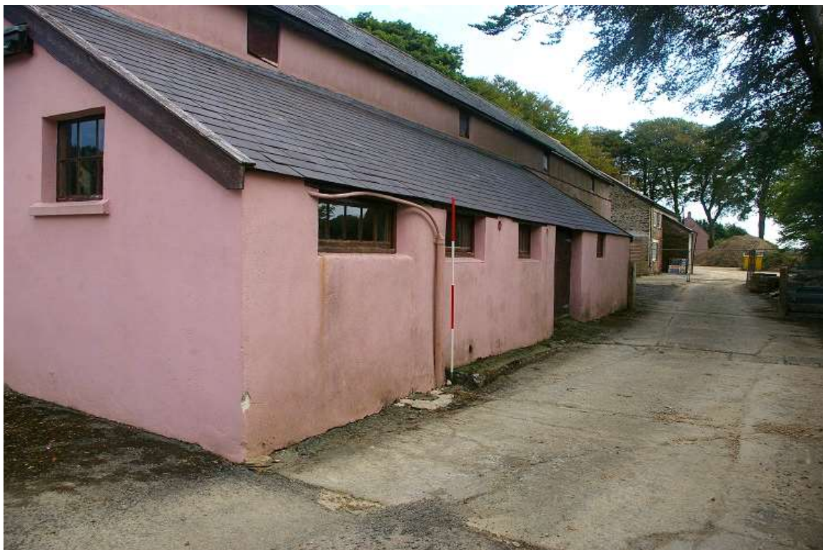
FIGURE 18: THE SOUTH ELEVATION SIDE OF THE GREAT BARN, THE SURVIVING STONE PILLAR INCORPORATED INTO THE CURRENT WALL BY THE SCALE (2M SCALE); VIEWED FROM THE SOUTH-WEST.
