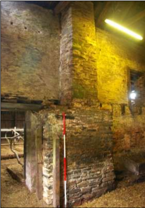
12. THE STACK WITH BLOCKED FIREPLACE AT THE SOUTH END OF THE GREAT BARN AT CORNHAM (2M SCALE); VIEWED FROM THE SOUTH-EAST.
