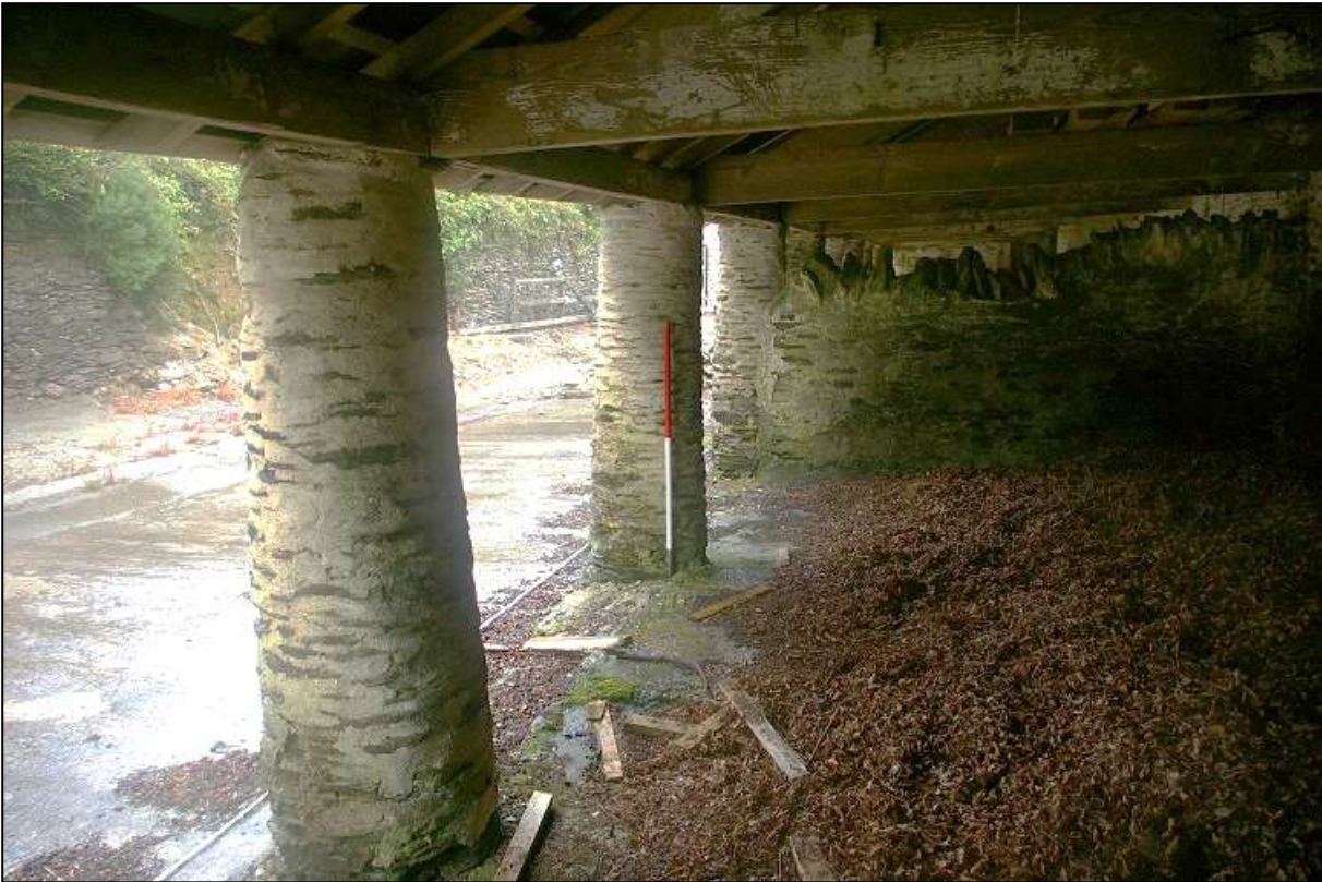
30. THE INTERIOR OF THE NORTH AISLE (2M SCALE); VIEWED FROM THE WEST.
