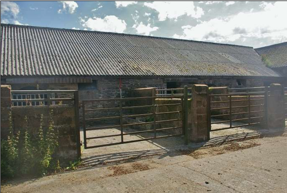
14. THE WEST ELEVATION (2M SCALE); VIEWED FROM THE NORTH-WEST.
