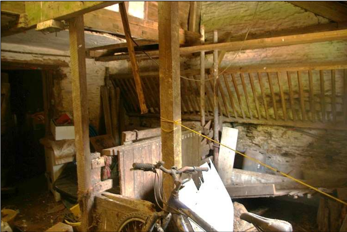
26. ROOM G, WITH HAYRACKS AND PLANK PARTITIONS, SHOWING A RETURN TO AGRICULTURAL FUNCTION AFTER A SHORT PERIOD OF DOMESTIC ACCOMMODATION CONVERSION; VIEWED FROM THE NORTH-WEST.
