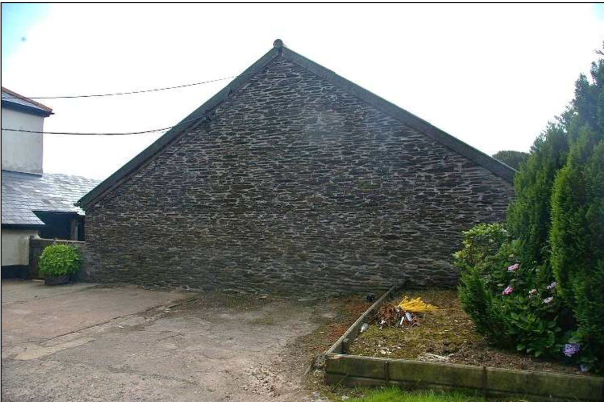
13. THE BLIND NORTH GABLE OF THE BUILDING; VIEWED FROM THE NORTH-WEST.
