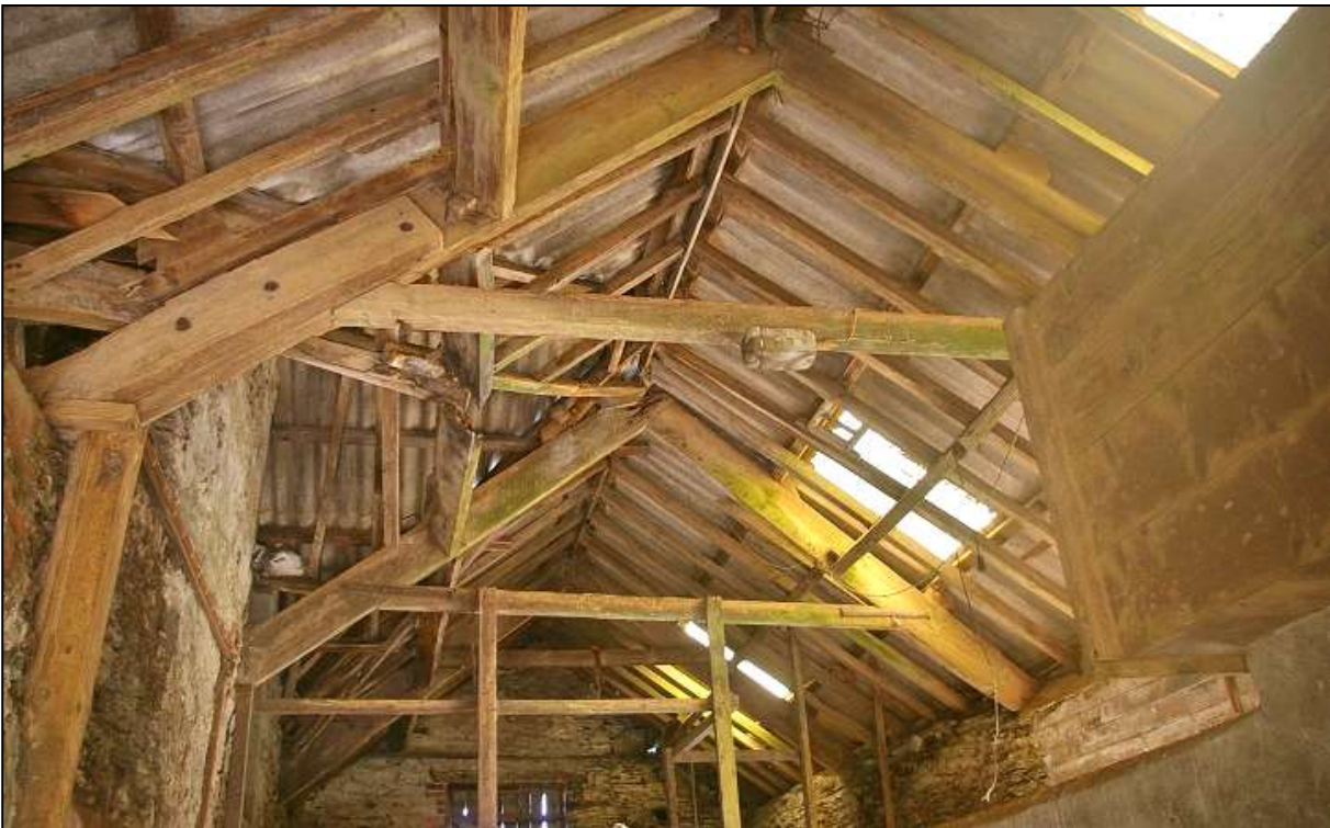
19. THE ROOF OVER ROOM A; VIEWED FROM THE WEST-NORTH-WEST.
