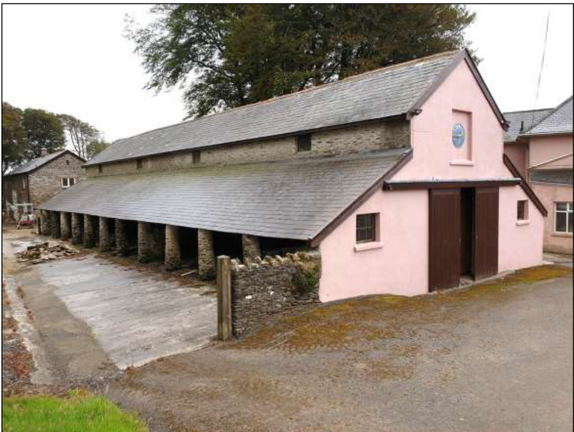
FIGURE 16: THE GREAT BARN AT HONEYMEAD (2M SCALE); THE WEST ELEVATION IS LARGELY OF RENDERED AND PAINTED CONCRETE BLOCK. VIEWED FROM THE NORTH-WEST.
