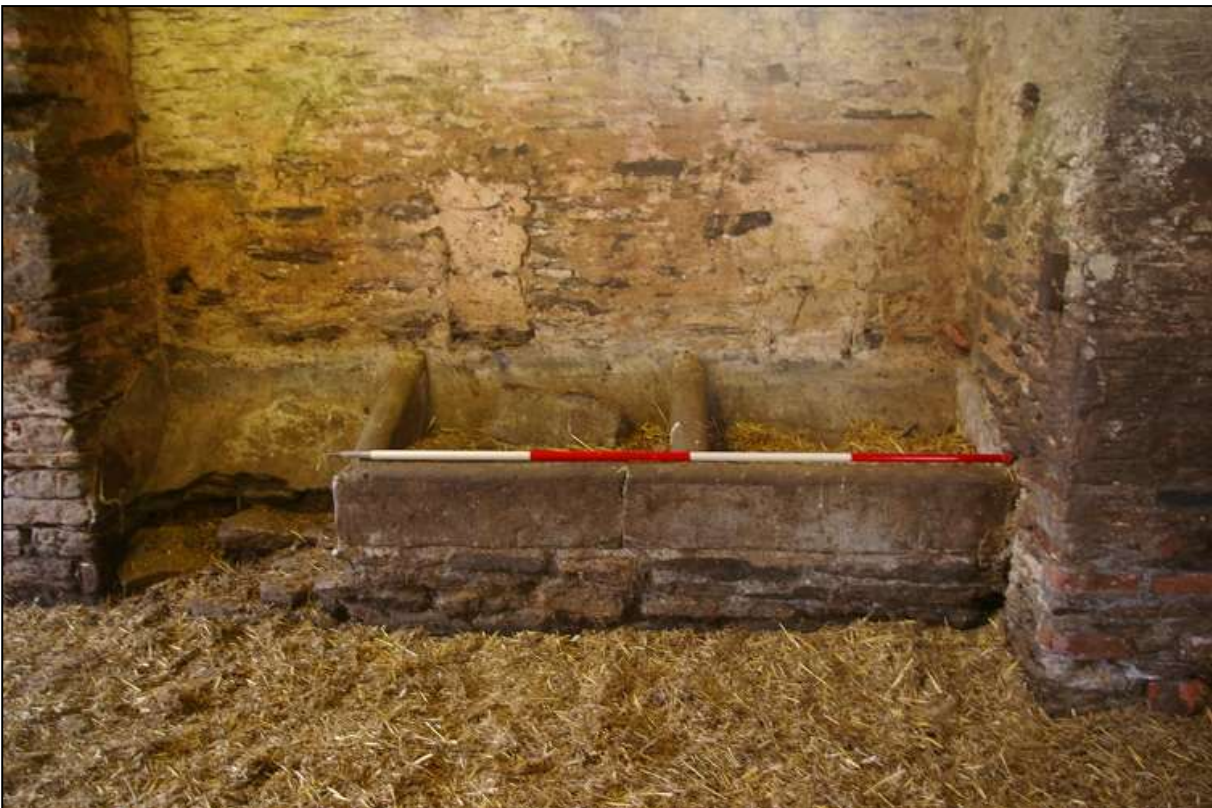
11. ONE OF THE INSERTED RUBBLE AND CONCRETE TROUGHS (2M SCALE); VIEWED FROM THE EAST.
