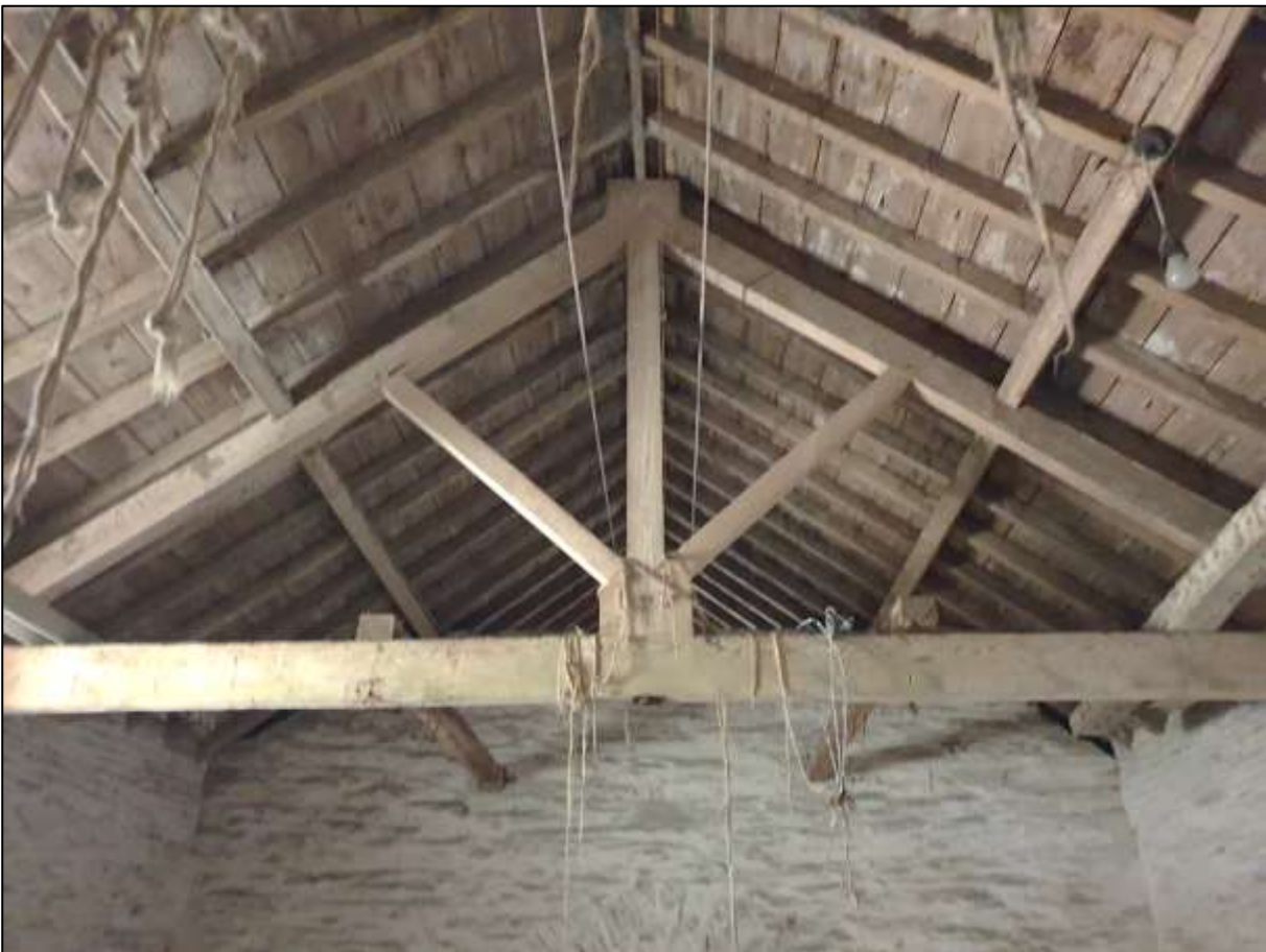
38. DETAIL OF THE KINGPOST ROOF STRUCTURE; VIEWED FROM THE WEST-NORTH-WEST.
