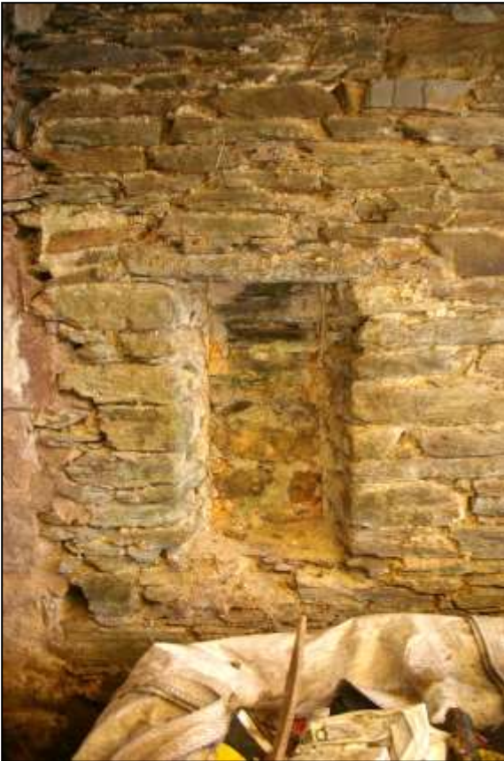
7. LEFT: ONE OF THE BLOCKED SLIT VENTS IN THE GREAT BARN AT CORNHAM, WEST WALL; VIEWED FROM THE WEST.
