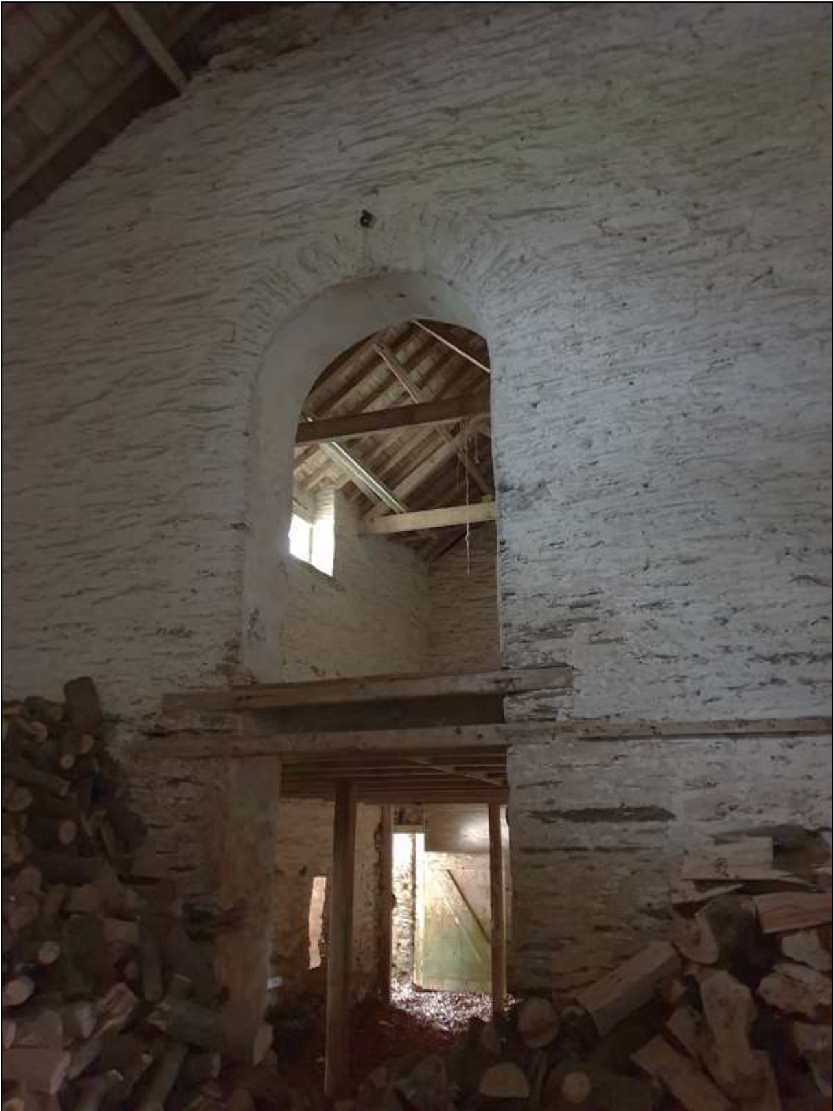
36. THE INTERNAL WALL OF ROOMS A AND B AT HONEYMEAD, SHOWING THE FULL-HEIGHT OPENING; VIEWED FROM THE WEST.
