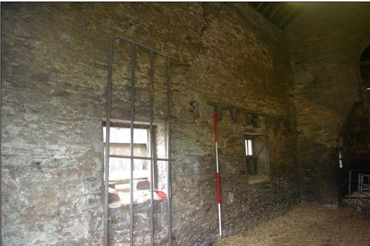
9. THE EAST WALL OF THE GREAT BARN AT CORNHAM, AT THE NORTH END SHOWING THE ABSENCE OF JOISTS SOCKETS AT THE NORTH END, DEFINING AN OPEN AREA FOR UNLOADING (2M SCALE); VIEWED FROM THE NORTH-WEST.
