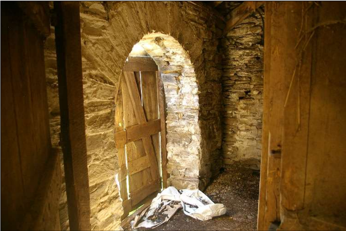
20. THE INTERNAL FACE OF THE SOUTHERN ROUND-HEADED ARCHWAY IN THE EAST ELEVATION, ROOM B; VIEWED FROM THE NORTH.
