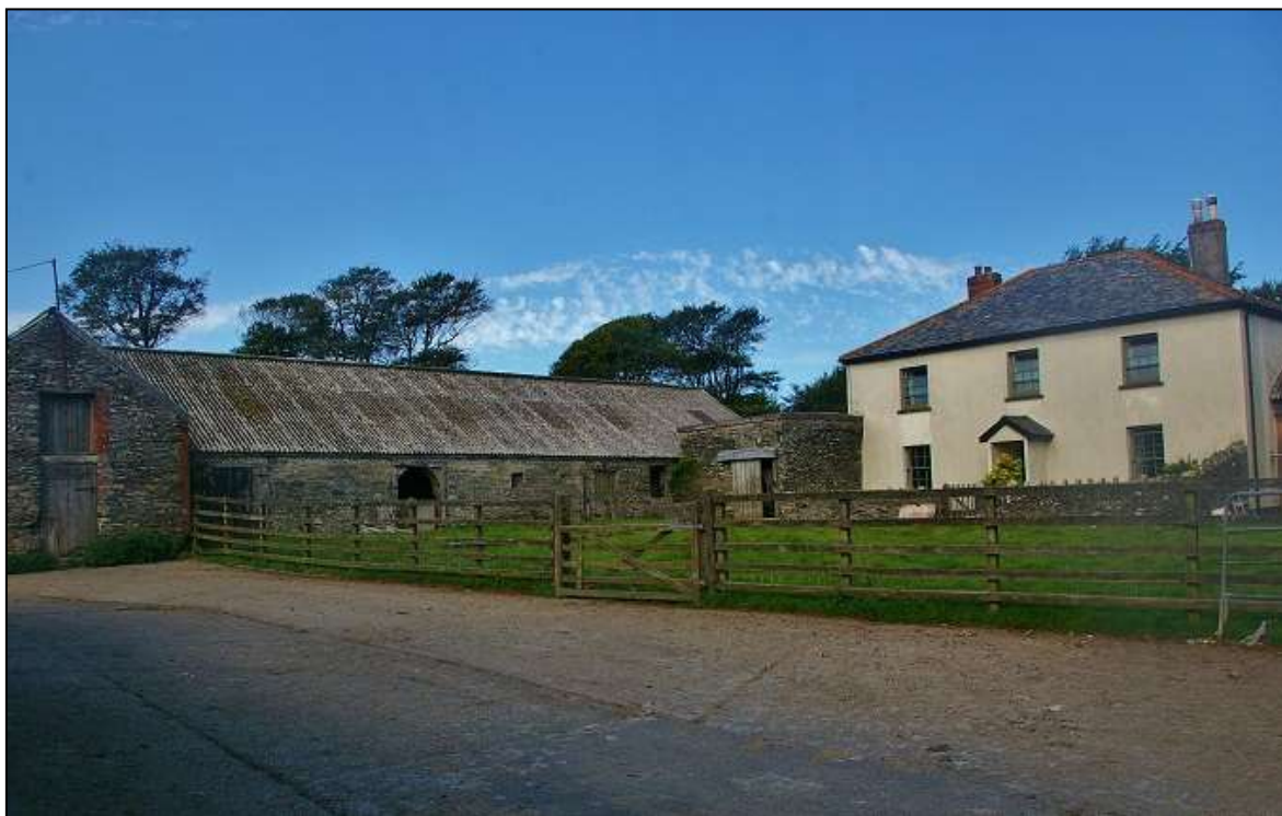
FIGURE 4: CORNHAM FARM, THE FARMYARD, FARMHOUSE, STABLES AND BARN (LEFT); VIEWED FROM THE SOUTH-EAST.
