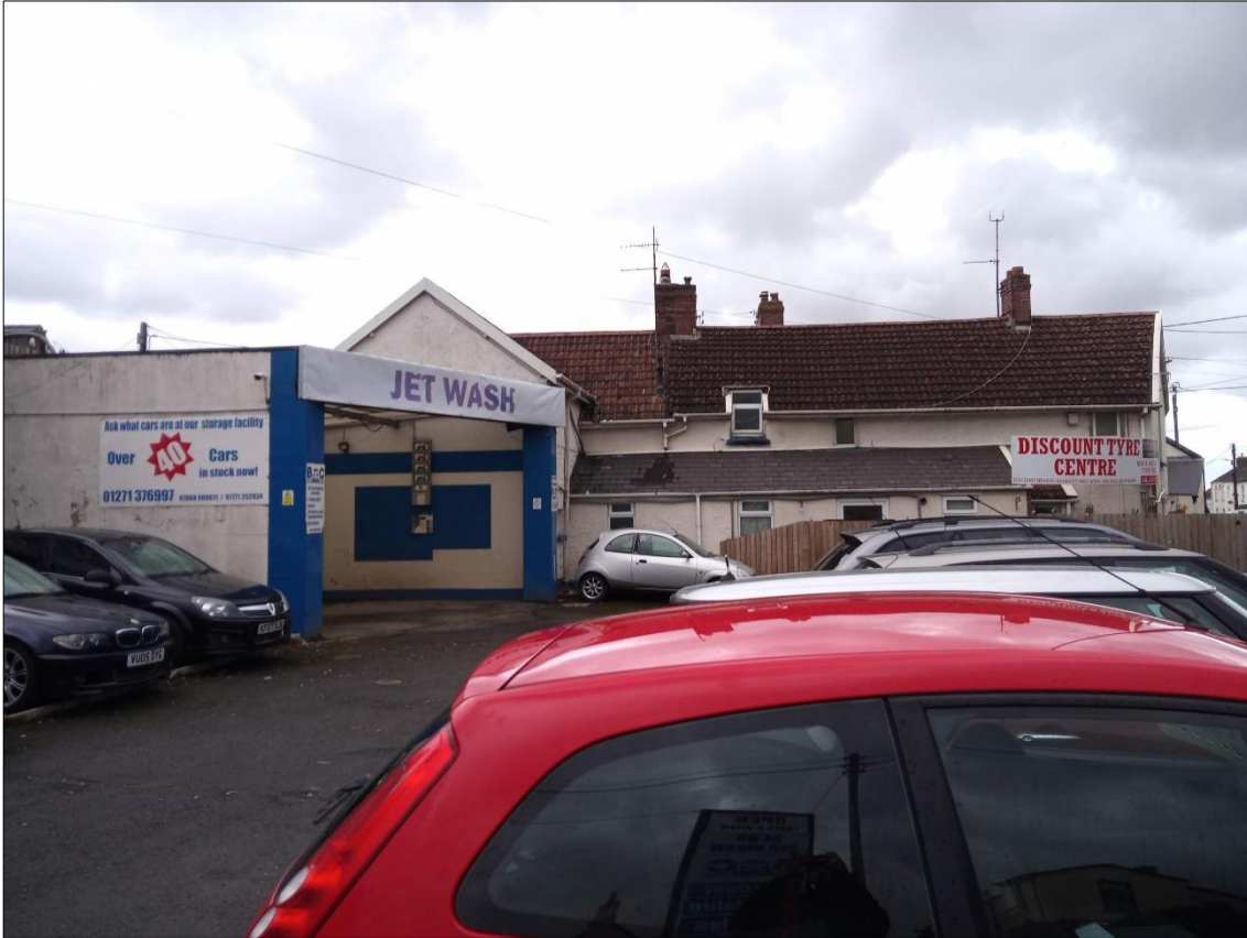
1. VIEW OF HOUSE TO THE WEST AND CAR WASH; VIEWED FROM THE EAST (NO SCALE).
