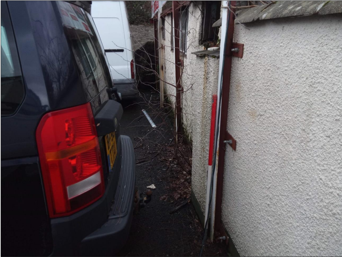
5. EDGE OF THE SITE TO THE EAST, WITH SHED BELONGING TO (DDV16743) ON THE RIGHT; VIEWED FROM THE SOUTH (1M SCALE).
