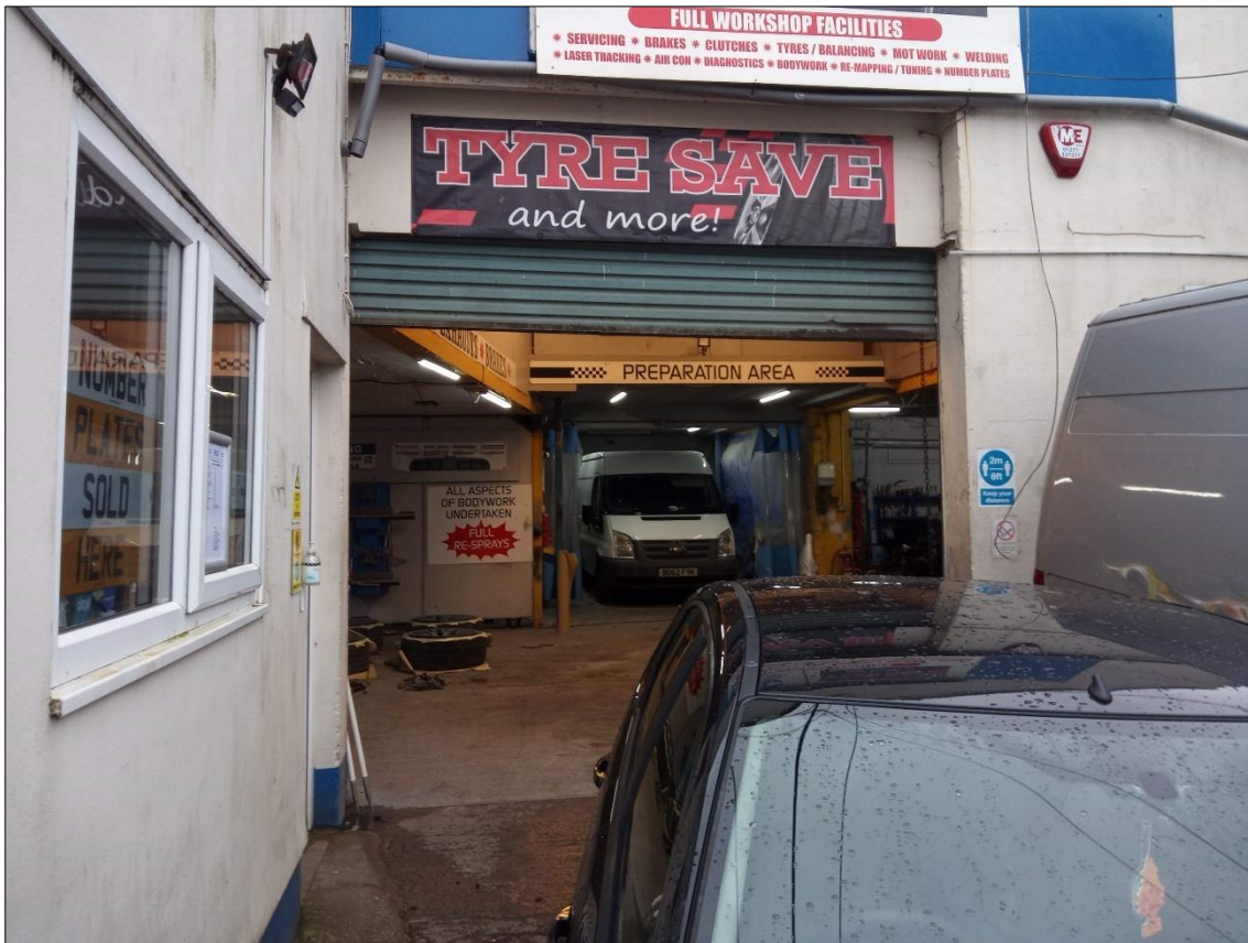
7. ENTRANCE TO WAREHOUSE GARAGE; VIEWED FROM THE NORTH (NO SCALE).
