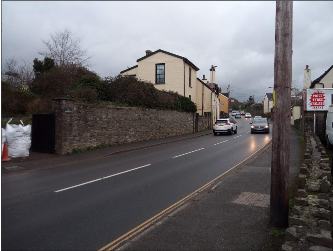
15. VIEW OF LISTED BUILDING (DDV4990), WITH GARDEN WALL ON THE LEFT; VIEWED FROM THE WEST (NO SCALE).
