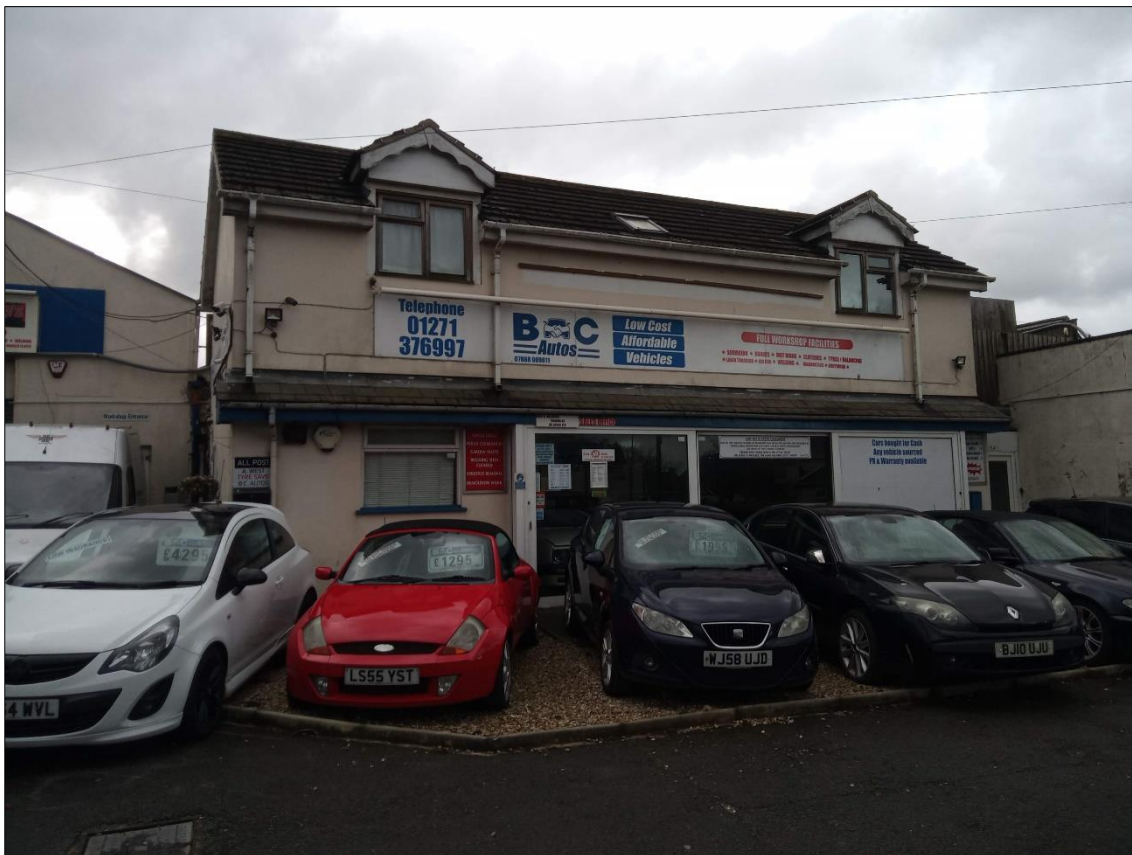
2. CAR SALES OFFICE; VIEWED FROM THE NORTH (NO SCALE).
