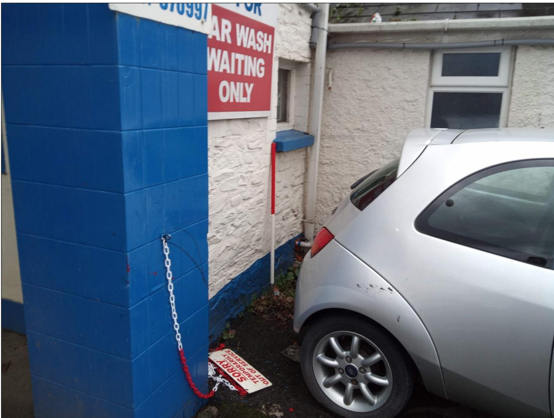
6. CAR WASH BUILDING JOINING HOUSE TO THE WEST; VIEWED FROM THE NORTH-EAST (1M SCALE).
