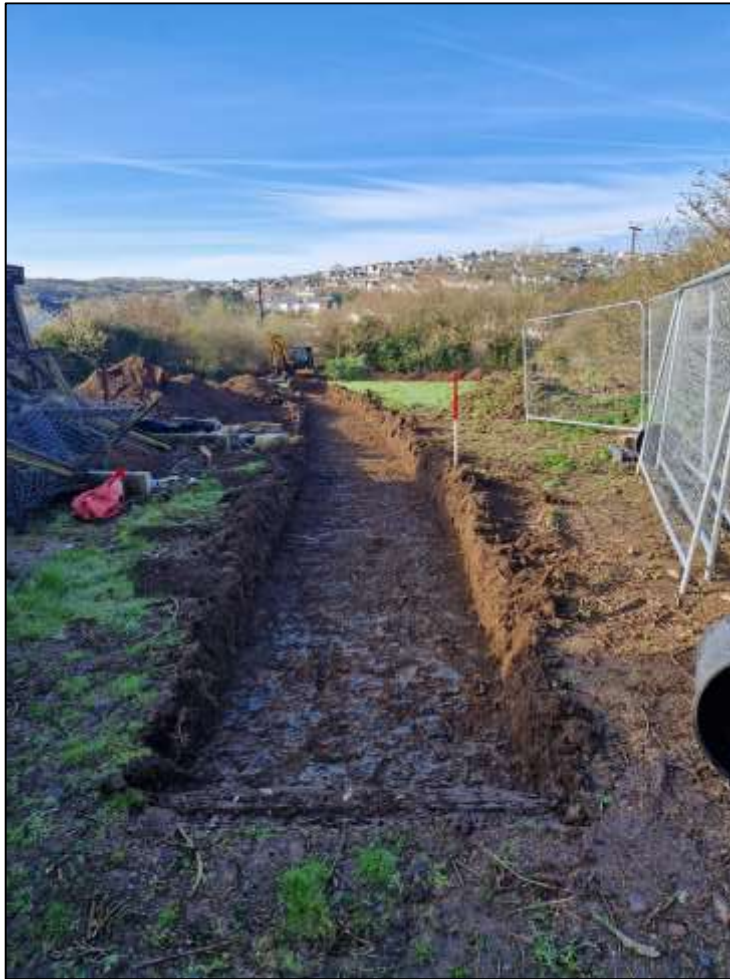
FIGURE 2: TRENCH 3, VIEWED FROM THE NORTH-EAST (1M SCALE).
