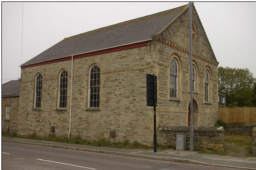
2. GOONHAVERN FORMER METHODIST CHAPEL AND SUNDAY SCHOOL; VIEWED FROM THE WEST.
