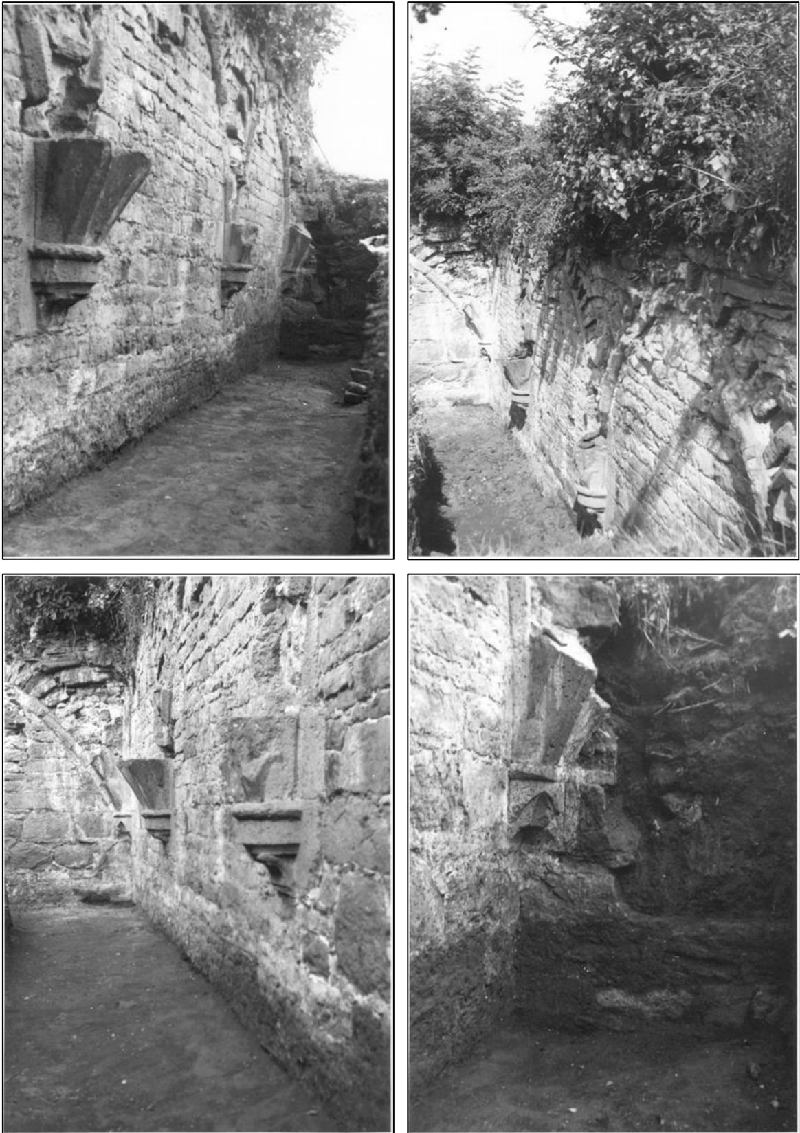
FIGURE 79: IMAGES OF THE EXCAVATED UNDERCROFT WALL AT BROADCLYST (NT COLLECTION). NOTE THAT THESE ALL APPEAR TO BE OF THE WEST ELEVATION OF THE WALL (I.E. WITHIN THE CHURCHYARD).
