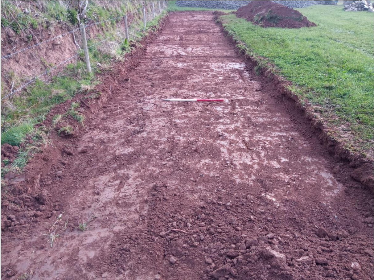
FIGURE 2: EXCAVATED AREA IN FIELD 1; FROM THE SOUTH-WEST (1M SCALE).
