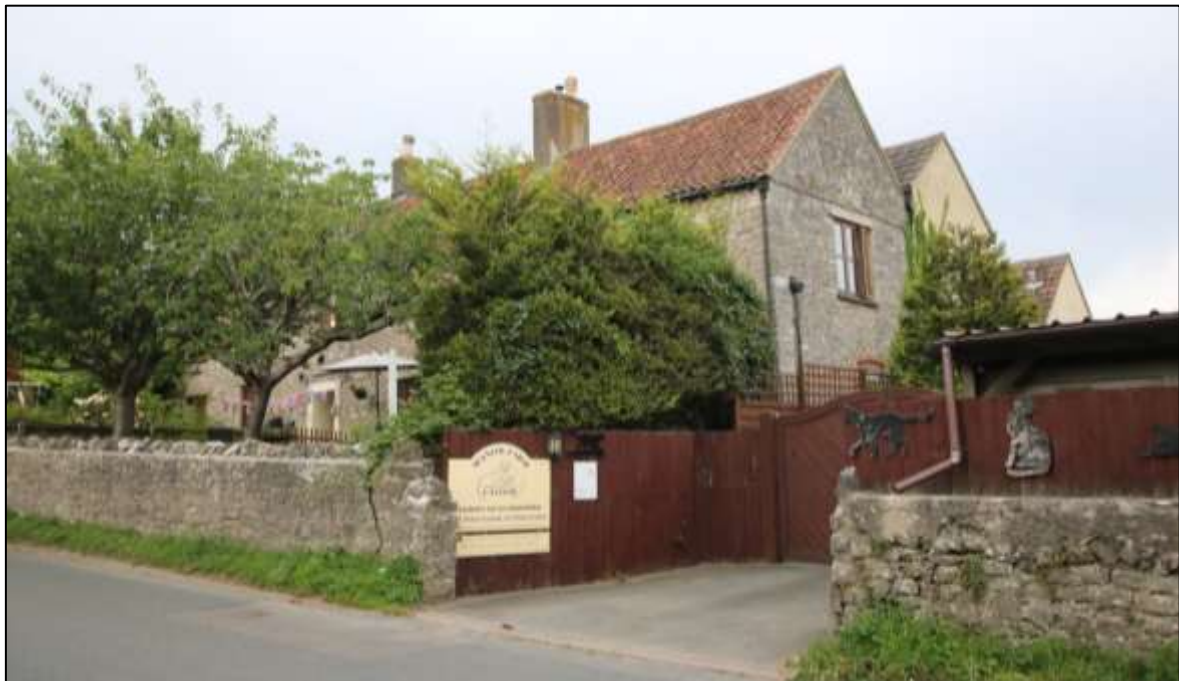
FIGURE 43: NORTON COURT FARMHOUSE; VIEWED FROM THE SSE, LOOKING NNW.
