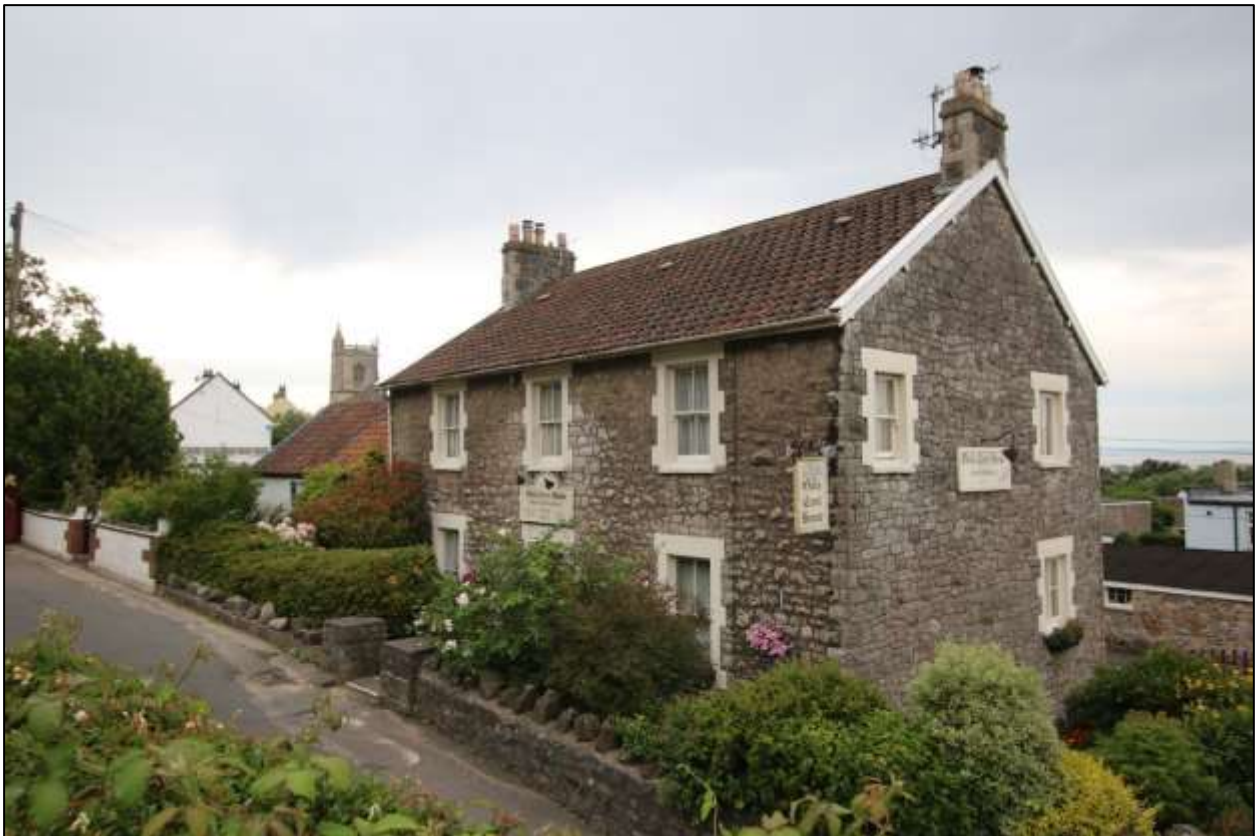
2. THE OWL'S COTTAGE CAFÉ AND ADJACENT OWL'S CREST HOUSE; VIEWED FROM THE EAST, LOOKING WEST.
