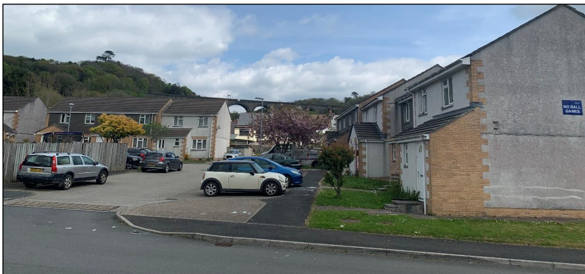
FIGURE 35: THE GOVER RAILWAY VIADUCT; VIEWED FROM THE SOUTH-WEST.
