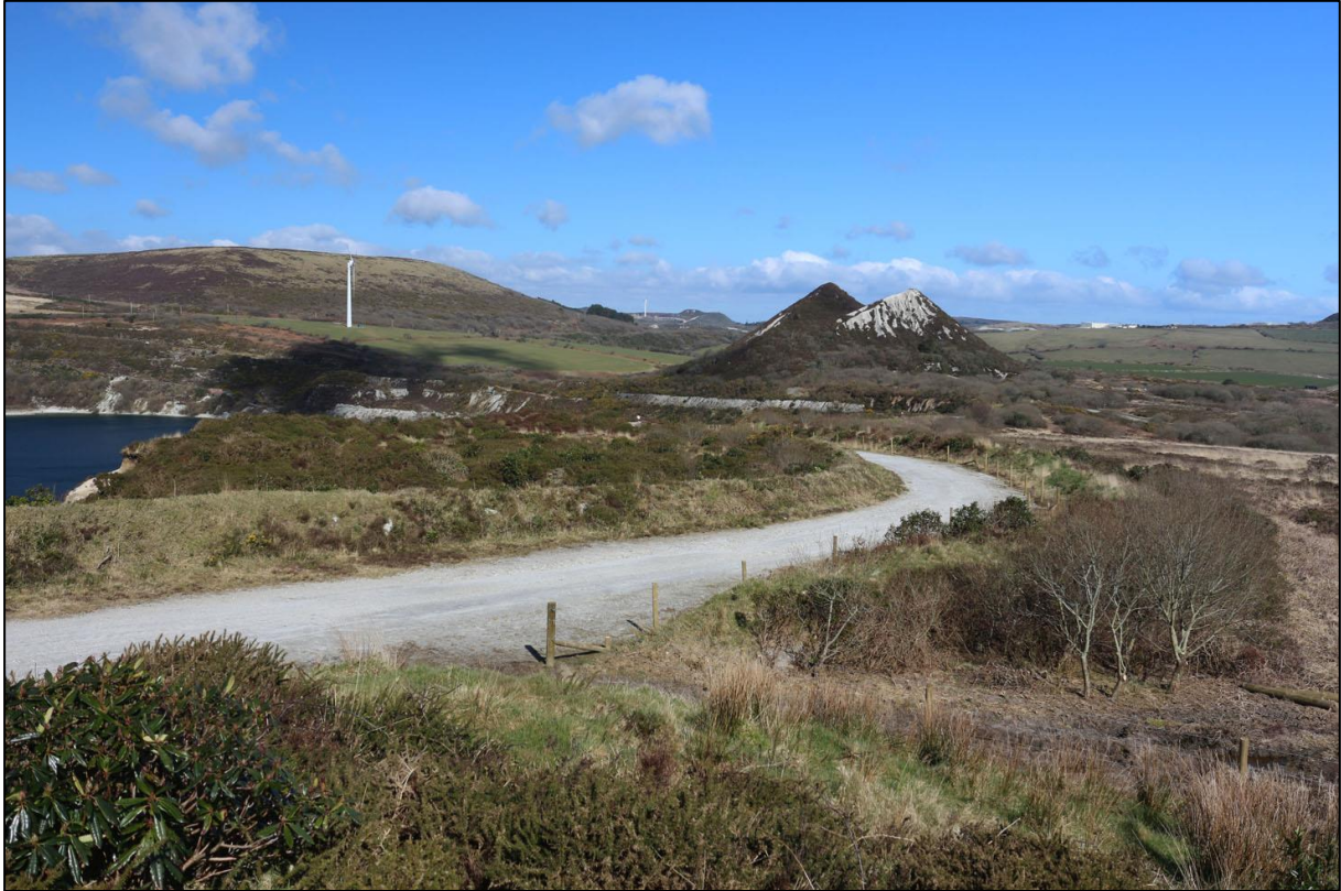
1. VIEW FROM THE NORTHERN TIP OF THE LINEAR SPOIL MOUND, LOOKING ALONG THE HAUL ROAD TO GOONAMARTH SKY TIP AND OPERATIONAL TURBINE; VIEWED FROM THE SOUTH-WEST.
