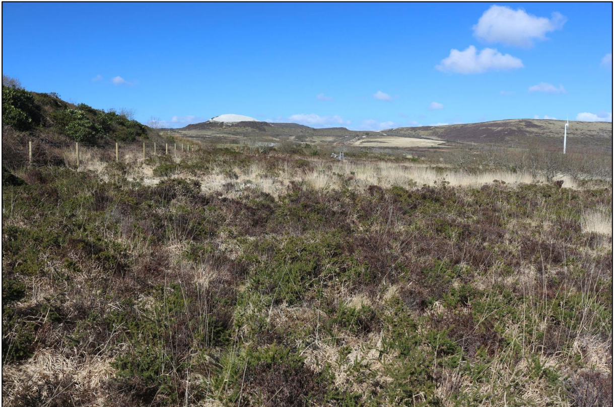
10. VIEW ALONG THE SIDE OF THE LINEAR SPOIL MOUND, LOOKING NORTH, WITH THE RELICT TRACKWAY IN THE FOREGROUND; VIEWED FROM THE SOUTH.
