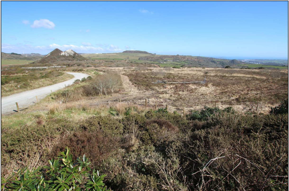
6. VIEW FROM THE NORTHERN TIP OF THE LINEAR SPOIL MOUND, LOOKING EAST ACROSS THE REMAINS OF BURNGULLOW COMMON; VIEWED FROM THE WEST.
