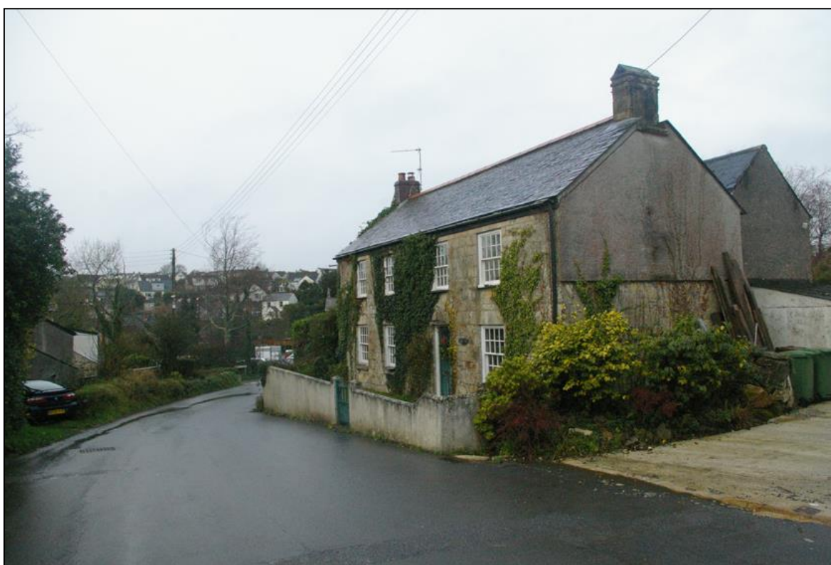
FIGURE 27: TRUDGEONS, IN STICKER; VIEWED FROM THE ESE [2015 PHOTOGRAPH].
