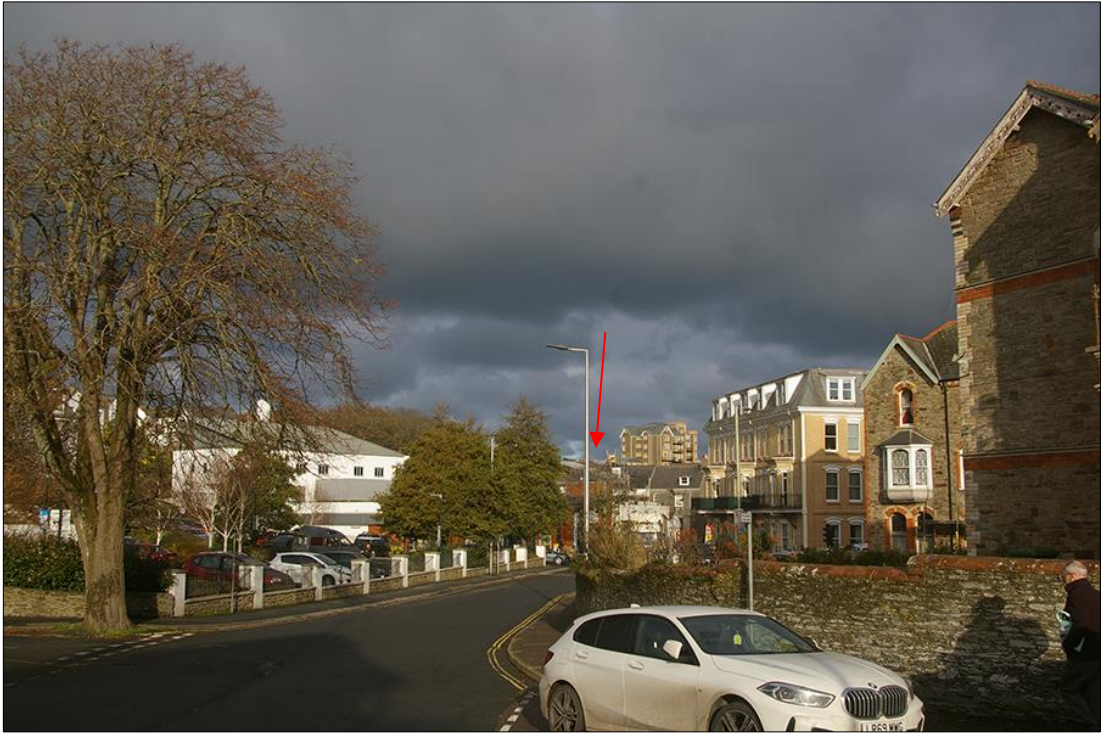
17. VIEW FROM WITHIN THE ILFRACOMBE CONSERVATION AREA (BROOKDALE LODGE) TOWARDS THE PROPOSAL SITE (INDICATED); VIEWED FROM THE SOUTH-SOUTH-WEST (NO SCALE).
