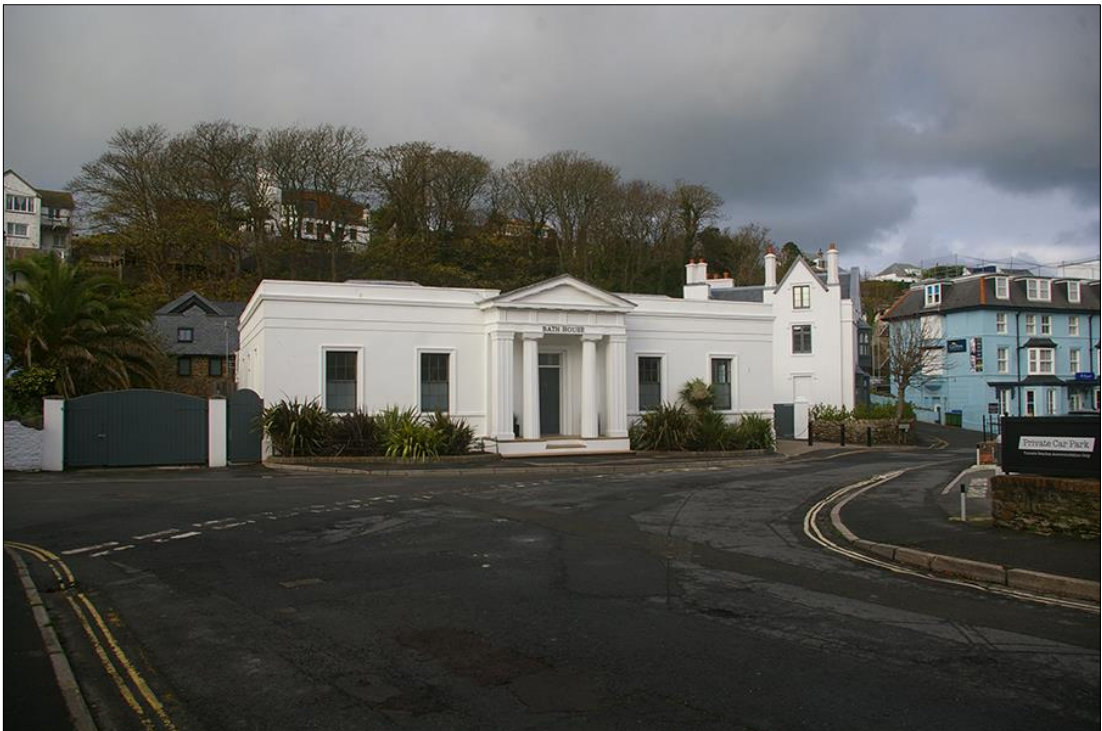
18. THE BATH HOUSE; VIEWED FROM THE SOUTH-SOUTH-EAST (NO SCALE).
