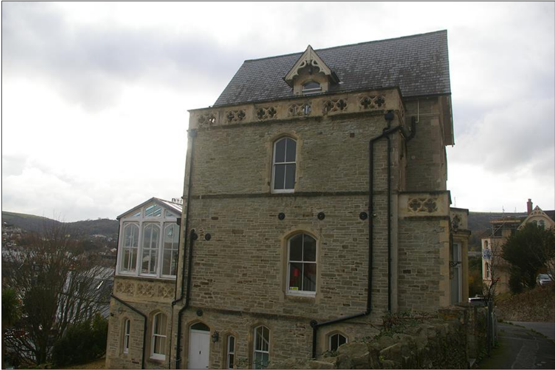
9. MERLIN COURT; VIEWED FROM THE NORTH-NORTH-EAST (NO SCALE).
