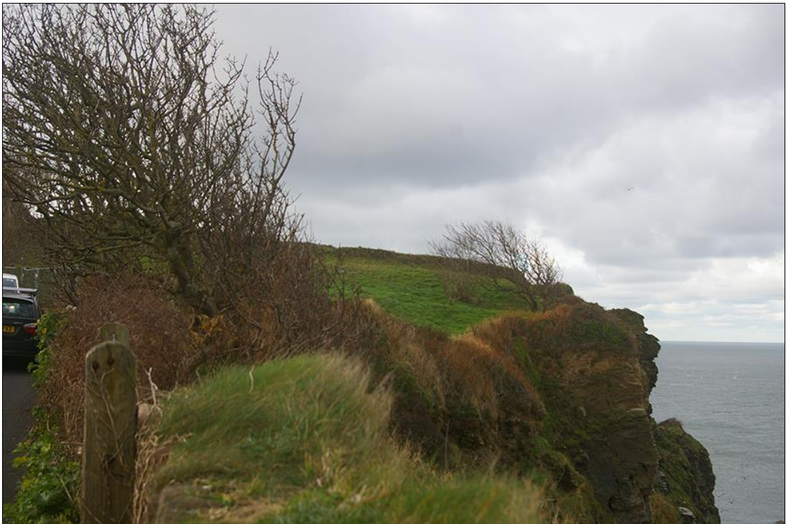
4. VIEW ACROSS THE SOUTH-EASTERN END OF THE PROPOSAL SITE; VIEWED FROM THE EAST-SOUTH-EAST (NO SCALE).
