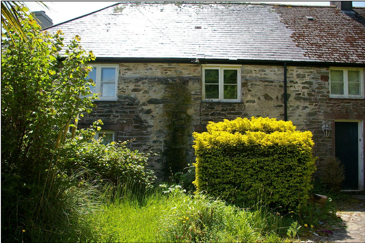
5. DETAILED VIEW OF THE THICKER LOWER SECTION OF WALLING WHICH DOMINATES THE NORTH FRONT OF THE FARMHOUSE, AT THE EAST END, THE REMAINS OF A RUINED EARLIER BUILDING; FROM THE NORTH.
