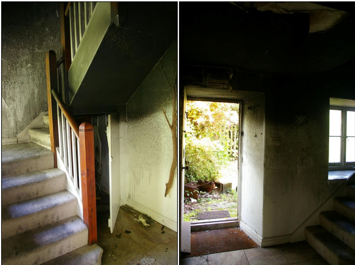
17. LEFT: VIEW OF THE LATE 20 TH CENTURY TIMBER STAIRCASE, HEAVILY SMOKE BLACKENED; FROM THE NORTH-WEST.
