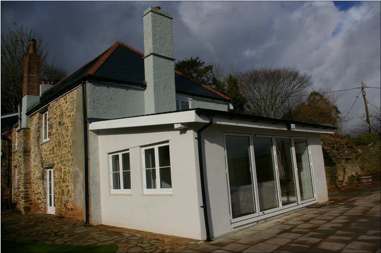
67. THE EAST GABLE OF THE FARMHOUSE AND NEW EXTENSION.
