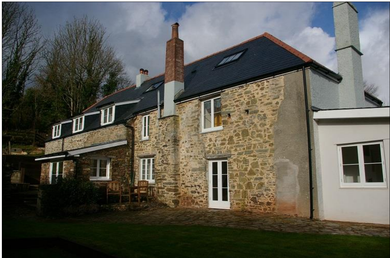
66. THE SOUTH ELEVATION OF THE FARMHOUSE.
