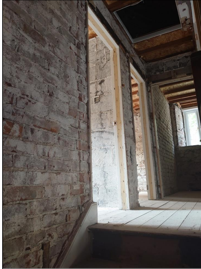
FIGURE 20: THE FIRST FLOOR, MUCH ALTERED BRICK PARTITIONS ON THE FIRST FLOOR OF THE COTTAGE; FROM THE EAST-NORTH-EAST.
