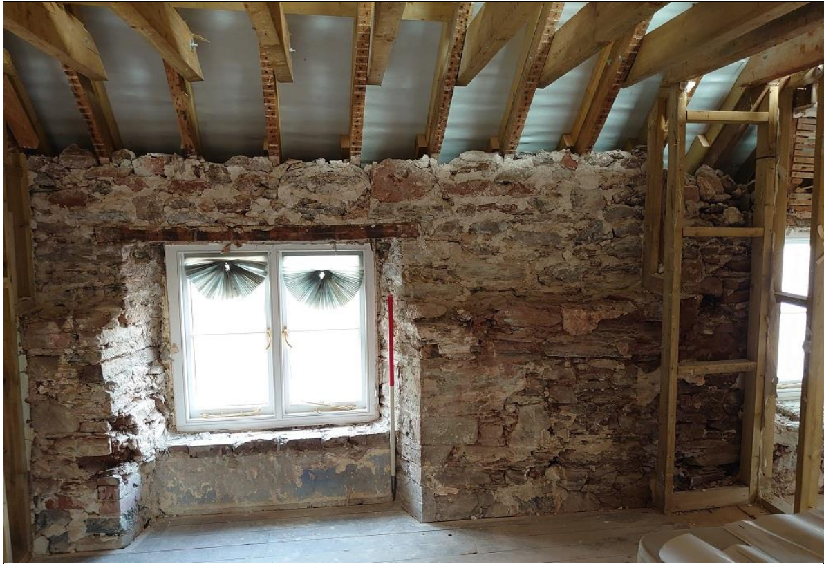
77. THE SOUTH WALL OF THE FARMHOUSE, WHERE MEDIEVAL WALLING, WITH FINE DRESSED DETAILS CAN BE SEEN TO BE RAISED BY POST MEDIEVAL RUBBLE (1M SCALE); FROM THE SOUTH.
