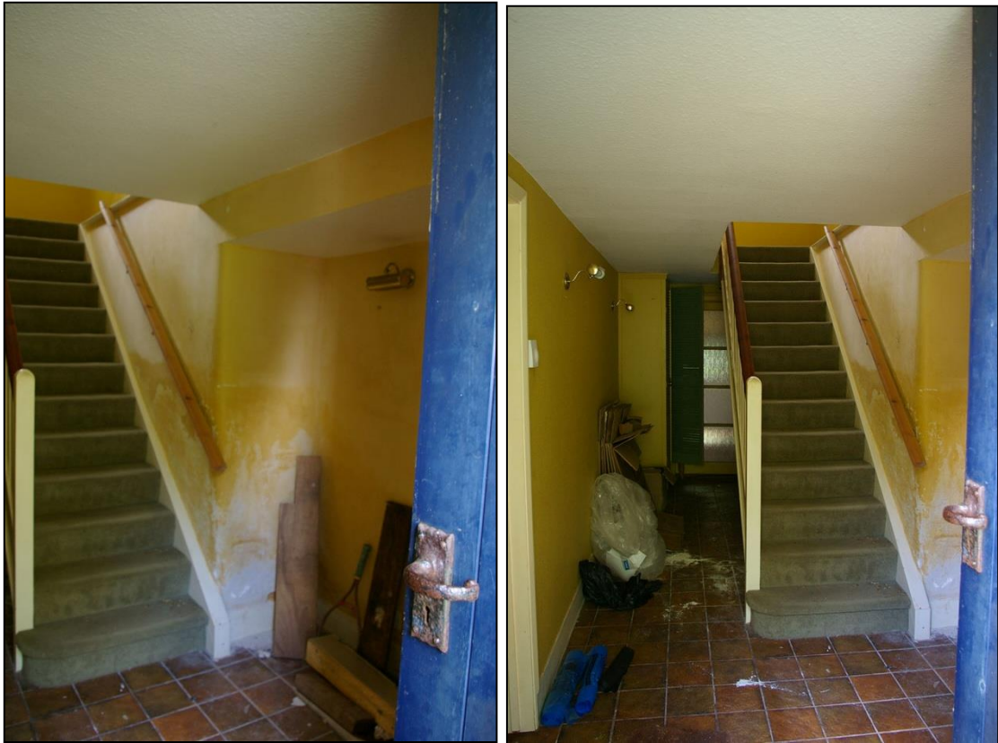
9. LEFT: INTO THE ENTRANCE HALLWAY AND STAIRS, ROOM 1, SHOWING HOW THIS DOOR HAS BEEN FORCED UP AGAINST THE PARTY WALL TO THE COTTAGE, WHICH HAS A LARGE BLOCKED DOORWAY WITHIN IT; FROM THE NORTH-EAST. RIGHT: THE HALLWAY, ROOM 1, ENTRANCE AND STAIRS, QUARRY TILED FLOOR, MODERN PARTITIONS DIVIDING THE SPACE AND PLASTER BOARDED CEILING AND MODERN GLAZED DOORS; FROM THE NORTH.
