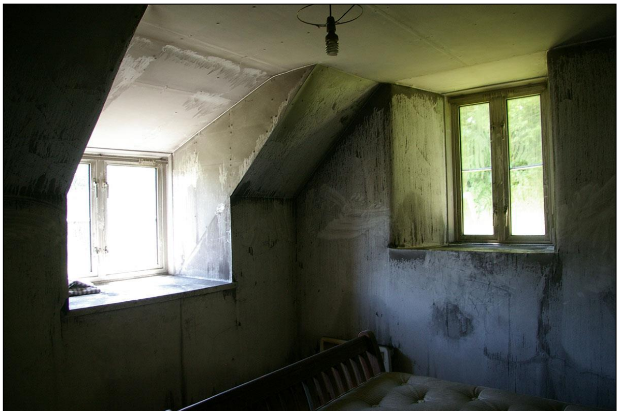
30. BEDROOM 1 WITH FORCED WINDOW OPENINGS AND PVC UNITS; FROM THE NORTH-EAST.
