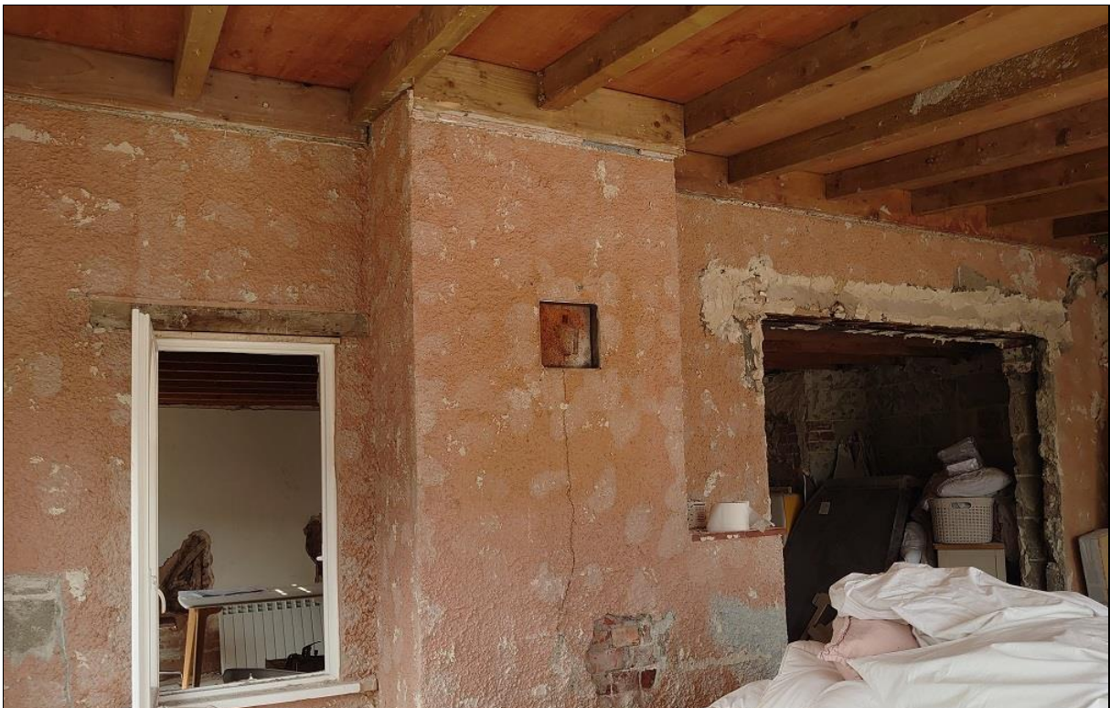
FIGURE 11: THE OUTER FACE OF THE EAST GABLE WITH EARLIER BRICK STACK; FROM THE EAST-SOUTH-EAST.
