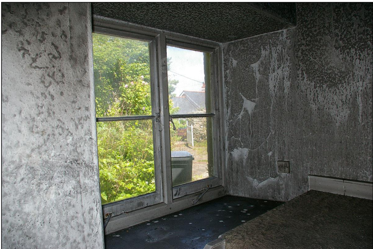
20. DEEP BEADED OPENING, PLANK SILL AND TWO LIGHT BEADED CASEMENT IN CHAMFERED PEGGED FRAME, A 19 TH CENTURY FEATURE CW1; FROM THE SOUTH-WEST.
