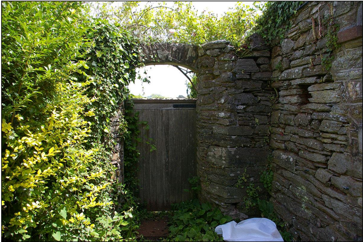
43. DETAILED VIEW OF THE FINE HEAVY SLATESTONE AND SOME DRESSED BLOCKS AND PUTLOGS, ALL OF WHICH IDENTIFY THESE GARDEN WALLS, AS IN FACT RUINS OF AN EARLIER QUITE FINE BUILDING, LIKELY PART OF THE COMPLEX WHICH SUPPORTED THE MANOR HOUSE WHICH STOOD ON THE SITE; FROM THE WEST.
