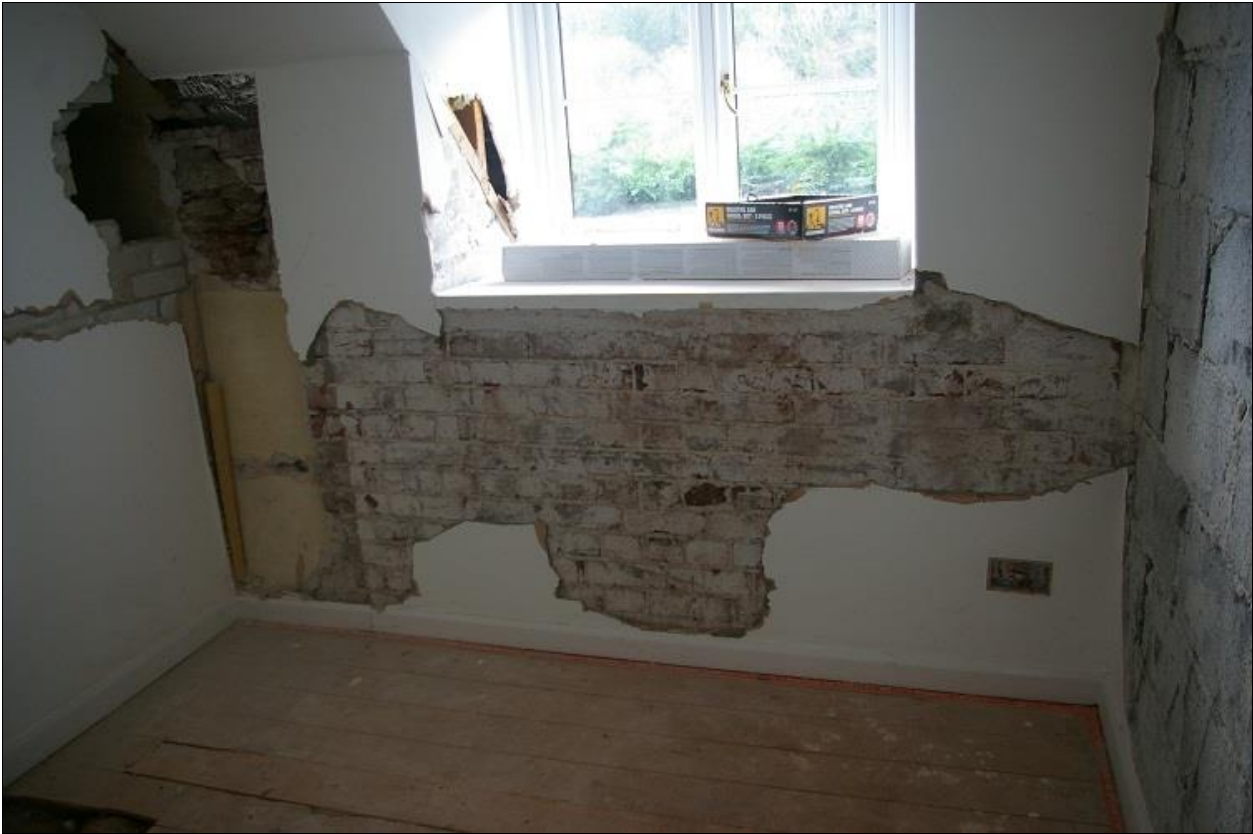
71. BRICK WALLING RAISING THE OLDER RUINED MEDIEVAL WALLS FORMING THE COTTAGE.
