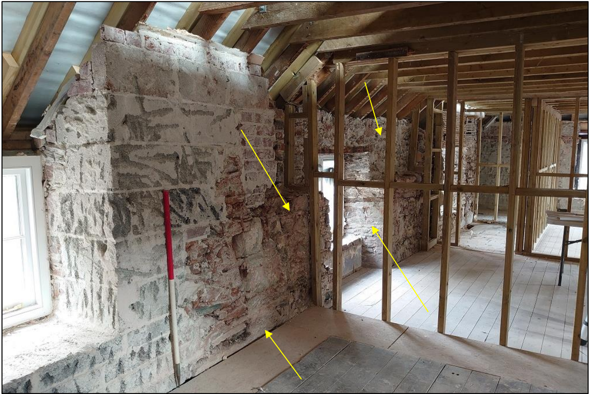
FIGURE 17: THE NORTH WALL OF THE FARMHOUSE, SHOWING 20TH CENTURY CONCRETE BLOCK, POST MEDIEVAL RUBBLE AND GOOD MEDIEVAL WALLING, IN THE COMPLEX PHASED REMAINS OF THE BUILDING (1M SCALE); FROM THE WEST-SOUTH-WEST.
