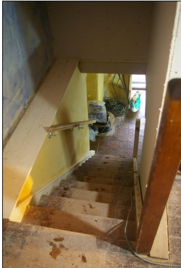
59. VIEW DOWN THE STAIRS IN THE FARMHOUSE, BUILT AGAINST THE THICK SLIGHTLY BATTERED FORMER GABLE WALL, SHOWING IT IS FAR THICKER TO THE GROUND FLOOR, WITH A MARKED LEDGE, WHERE THE MEDIEVAL WALL STOPS, HAVING BEEN RUINED AT SOME STAGE, FROM THE SOUTH.
