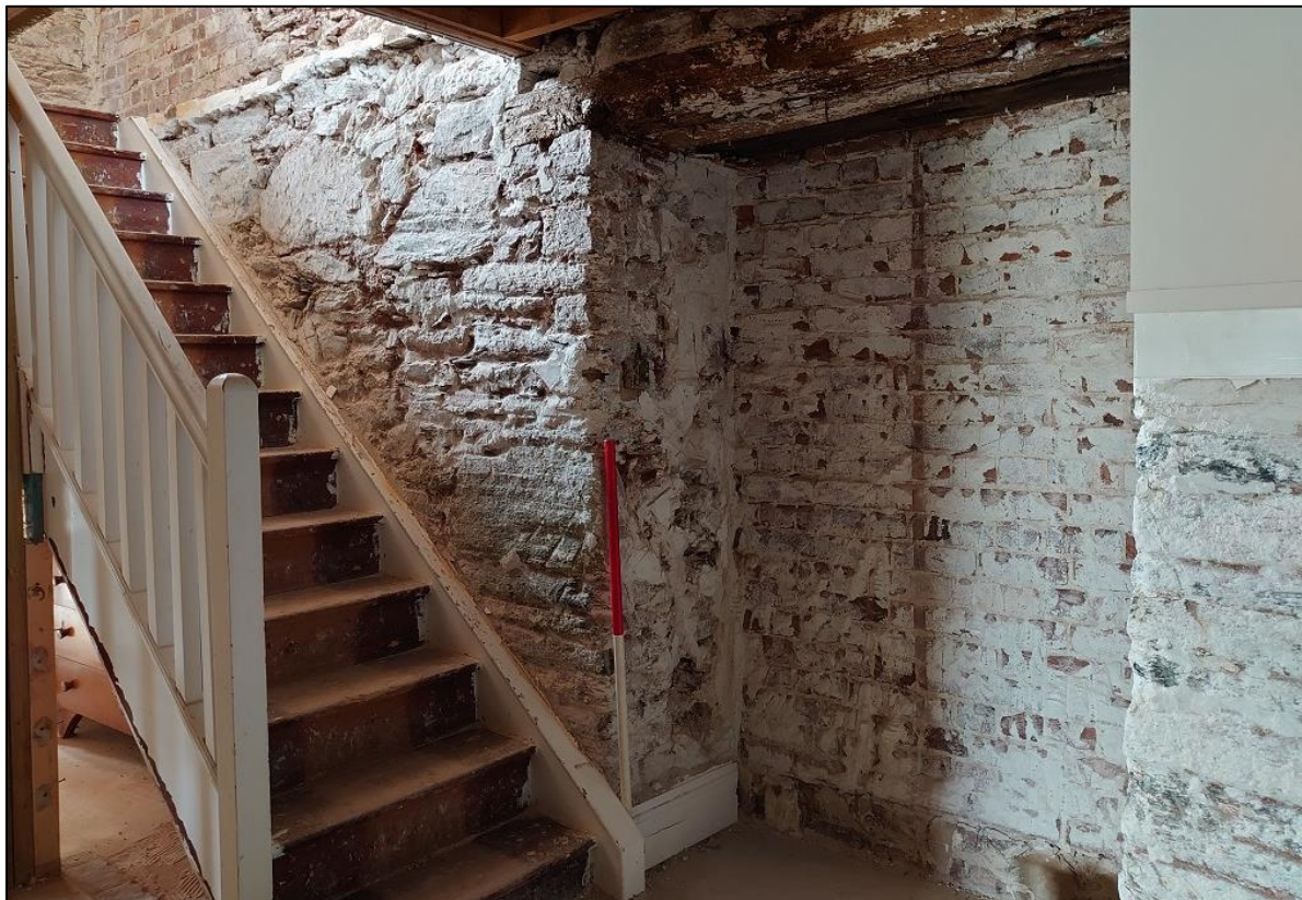
FIGURE 15: THE BLOCKED DOORWAY BETWEEN THE COTTAGE AND MAIN FARMHOUSE, BLOCKED WITH 19 TH CENTURY BRICKWORK (1M SCALE); FROM THE NORTH-EAST.
