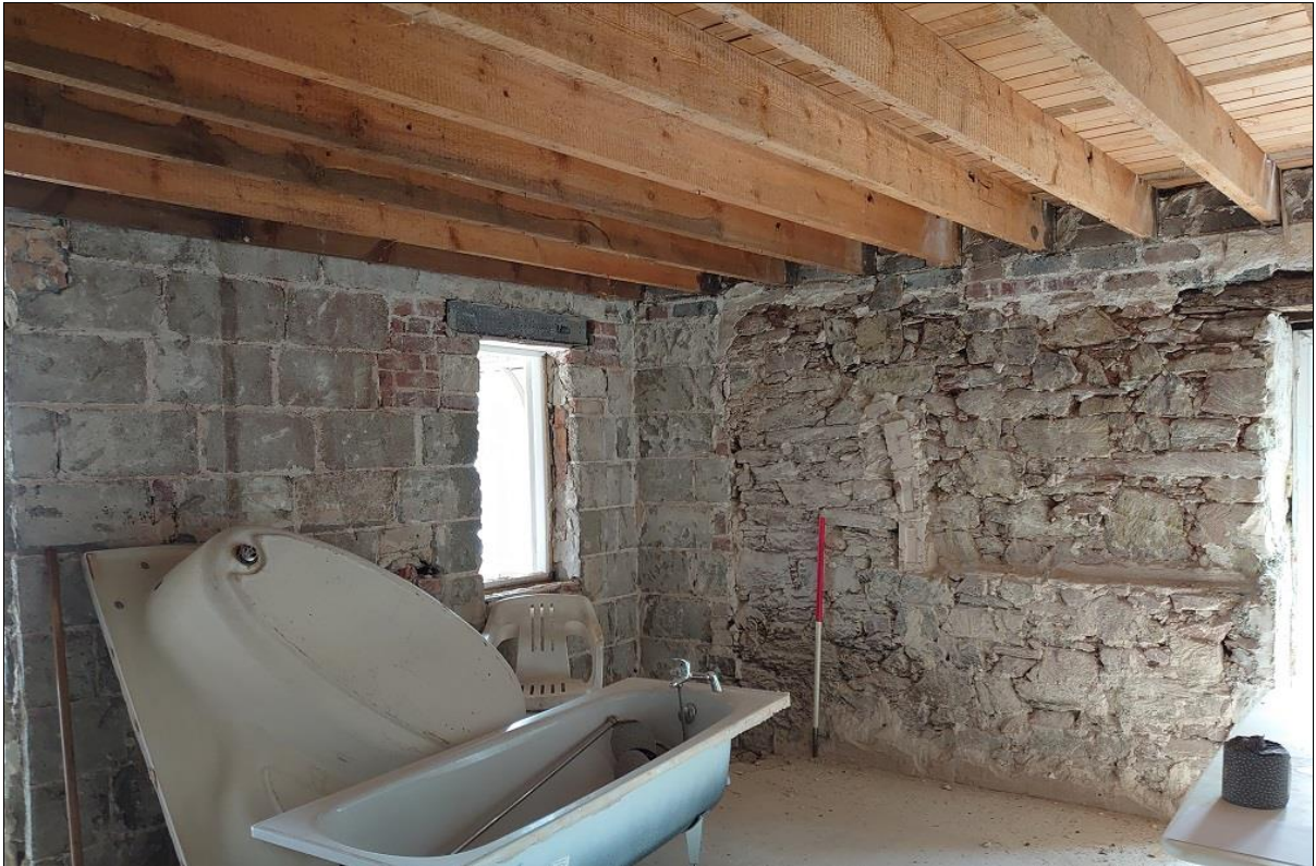
FIGURE 10: THE GROUND FLOOR, BATSON FARMHOUSE, SOUTH WALL, WITH MEDIEVAL AND POST -MEDIEVAL STONE WALLING AND THE CONCRETE BLOCK AND BRICK EAST GABLE, INNER FACE (1M SCALE); FROM THE NORTH-WEST.
