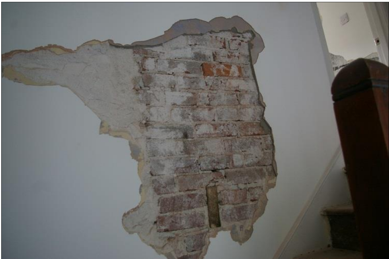
70. BRICK NOGGIN WALL FORMING PARLOUR AND BEDROOM IN THE COTTAGE.
