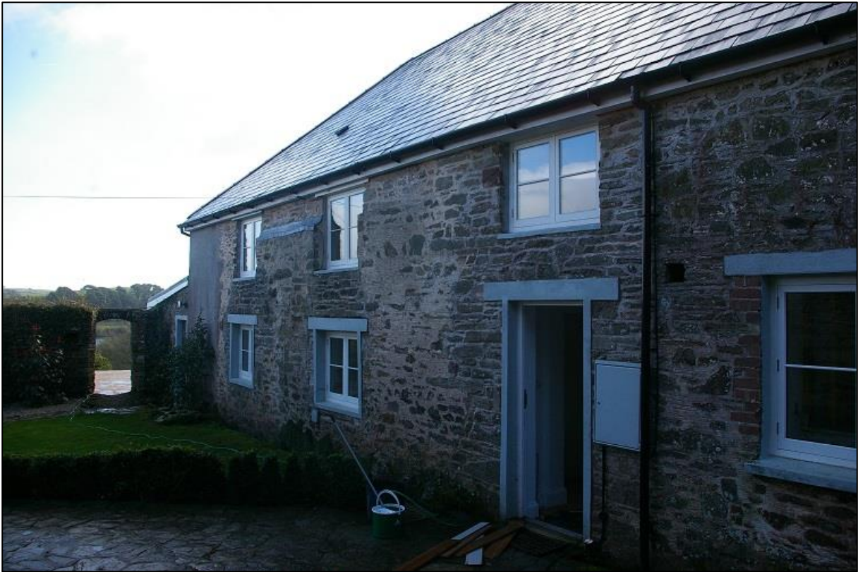
61. FRONT OF THE HOUSE, NORTH ELEVATION.
