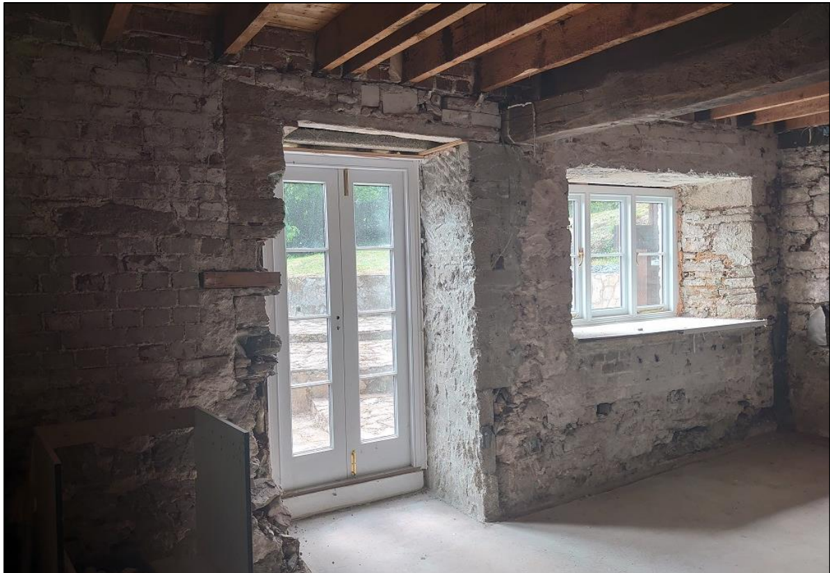
FIGURE 19: THE SOUTH WALL OF THE COTTAGE, WITH MEDIEVAL STONEMWORK, POST MEDIEVAL RUBBLE AND 19TH CENTURY BRICKWORK, INFILLING THE EARLIER WINDOW; FROM THE NORTH-EAST.
