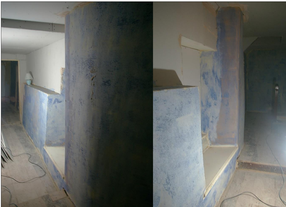
55. LEFT: THE SOUTH WALL OF THE FARMHOUSE, SHOWING THE BATTERED LOWER EARLIER SECTION OF WALL AND THE TALL ANGLED WEST PROJECTION, WITH DISTINCTIVE CURVE; FROM THE WEST-NORTH-WEST.
