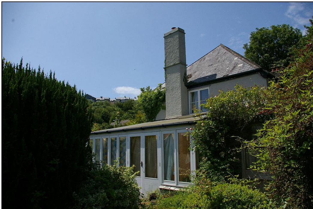
42. THE EAST GABLE END OF THE FARMHOUSE, WITH HIPPED ROOF, BOX STACK AND SHAFT AND LARGE MODERN CONSERVATORY; FROM THE NORTH-EAST.
