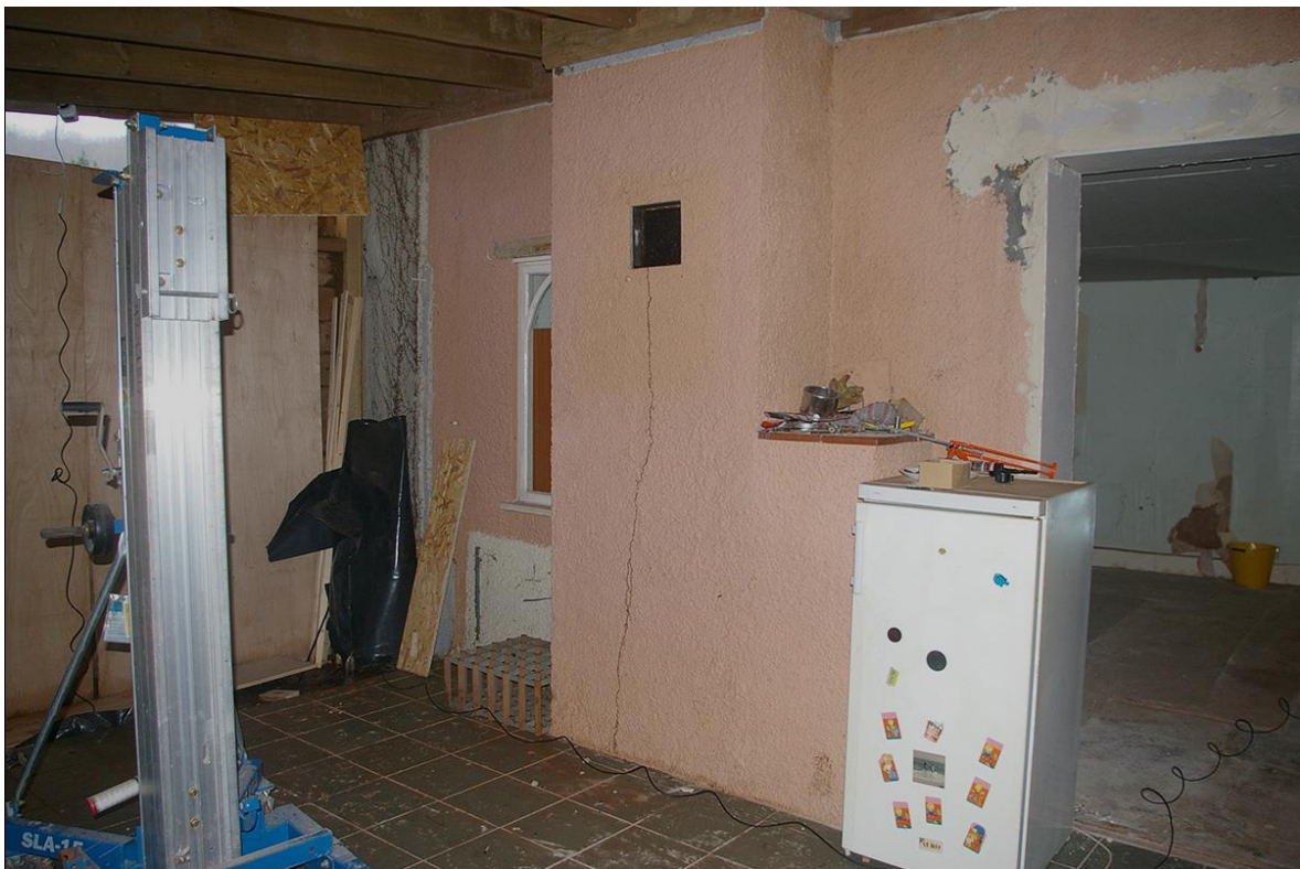
53. THE MODERN BOXY STACK SERVING THE SITTING ROOM FIREPLACE, ENCLOSED WITHIN THE CONSERVATORY; FROM THE NORTH-EAST.
