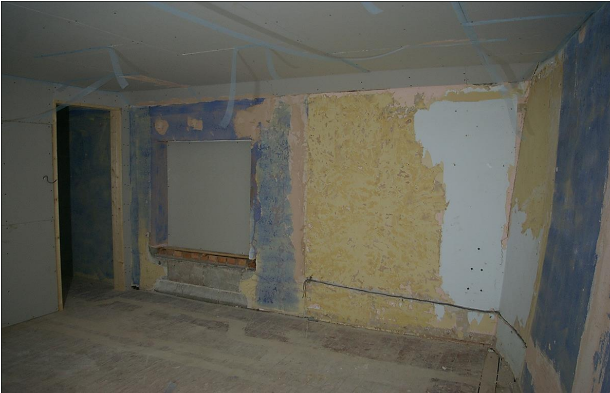
54. ROOM 9, BEDROOM 1, TO THE SOUTH OF THE BUILDING, SHOWING THE BATTERED AND ANGLED FRAGMENT OF EARLIER WALL TO THE SOUTH-EAST CORNER; FROM THE SOUTH-WEST.
