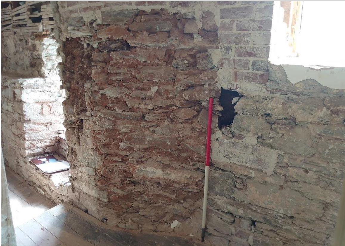
75. THE 17 TH CENTURY FABRIC OF A RUBBLE-BUILT STAIR TURRET, INFILLING BETWEEN TWO FRAGMENTS OF EARLIER MEDIEVAL STONework, REMAINS OF DETACHED BLOCKS, PART OF A COMPLEX EARLIER SITE, ALL CONTAINED WITHIN THE SOUTH FIRST FLOOR WALL OF THE FARMHOUSE (1M SCALE); FROM THE NORTH-WEST.
