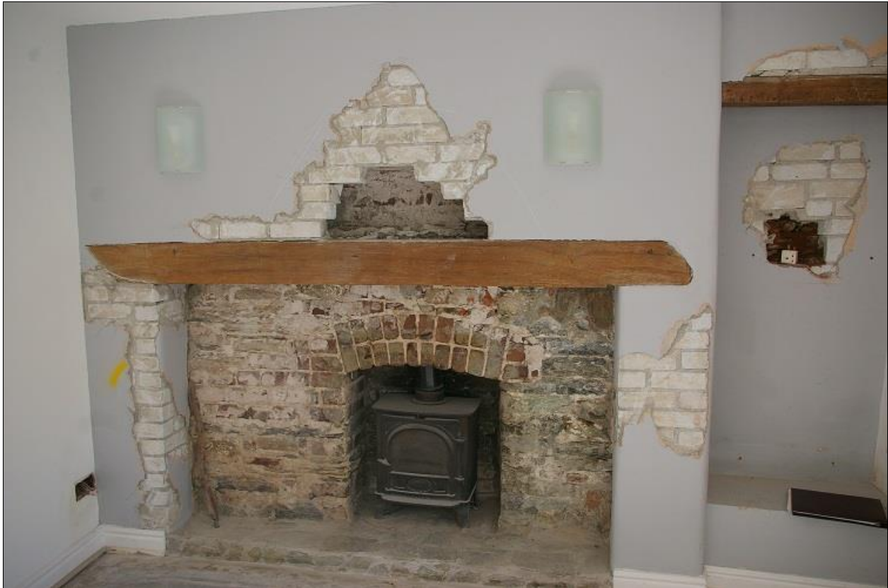
69. POST MEDIEVAL SMALL BOX HEARTH SET INTO THICK MEDIEVAL WALLING, FORMING A SMALL FIREPLACE, COVERED OVER BY MODERN BRICK.
