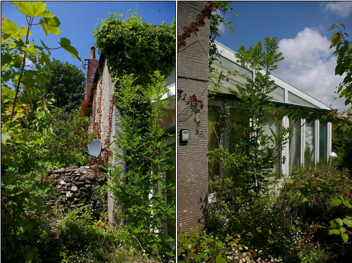
40. LEFT: VIEW ALONG THE BACK OF THE FARMHOUSE, SHOWING HOW IT IS ALMOST TOTALLY OBSCURED BY OVERGROWTH; FROM THE EAST.
