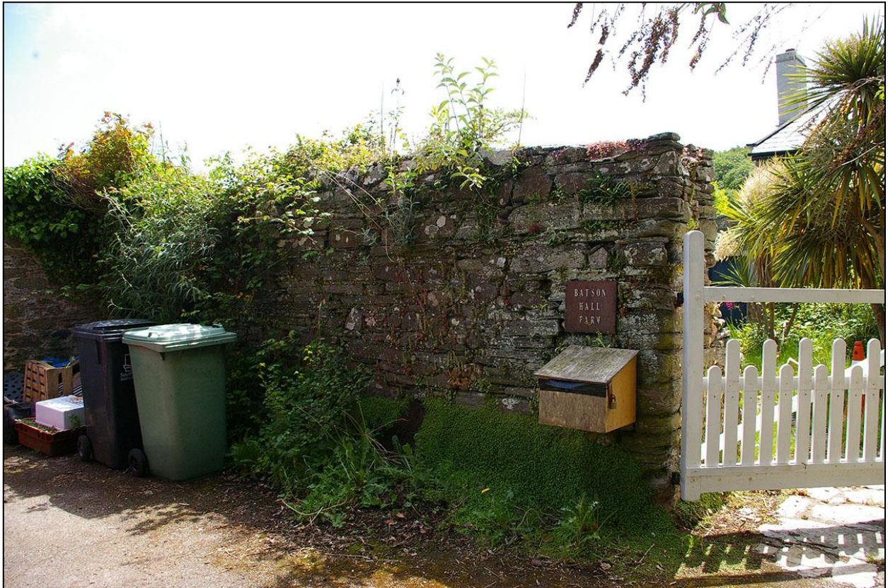
45. THE NORTH OUTER FACE OF THE HEAVY SLATESTONE WALL, WHICH IS THE FORMER GABLE END OF AN EARLY BUILDING; FROM THE NORTH-WEST.
