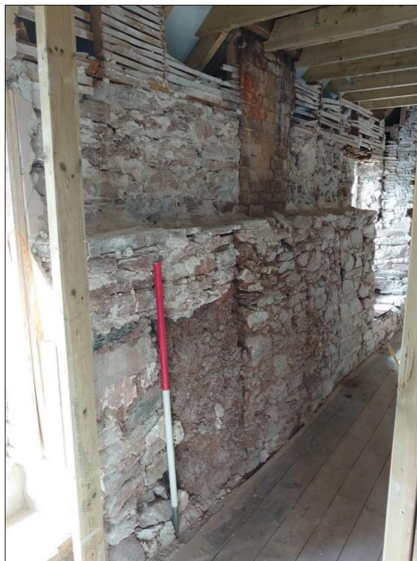
76. THE SOUTH WALL OF THE FARMHOUSE, AT FIRST FLOOR, WITH AT LEAST TWO PHASES OF POST MEDIEVAL FLUE CUT INTO BELOW MEDIEVAL STONework AND ABOVE AN EARLIER, LIKELY 17 TH OR 18 TH CENTURY RAISE AT THE EAVES (1M SCALE); FROM THE NORTH-EAST.
