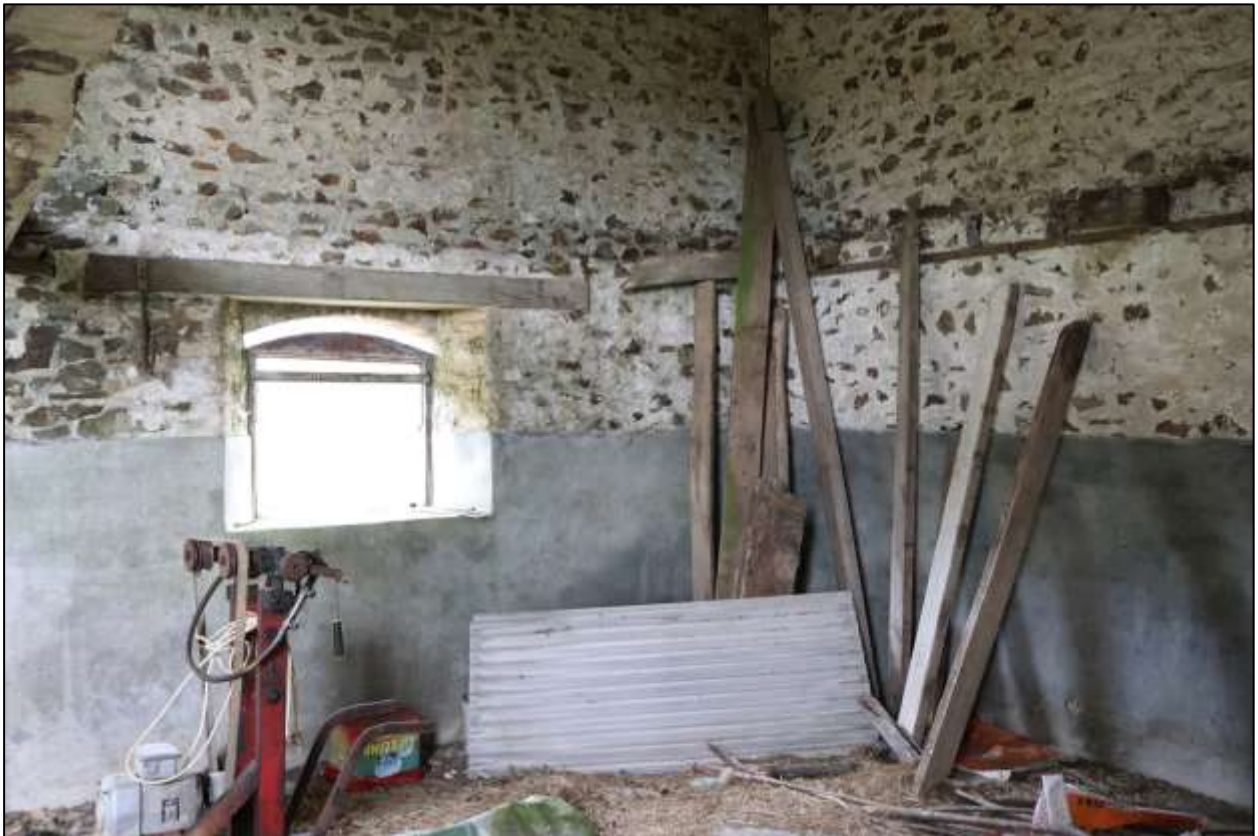
FIGURE 20: THE NORTH-WEST CORNER OF THE BARN, SHOWING THE SCARRING FOR THE LOFT FLOOR; VIEWED FROM THE SSE.
