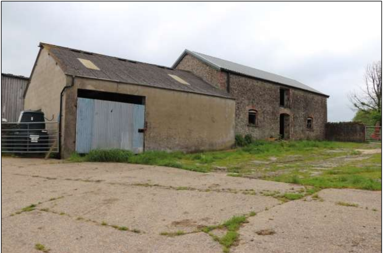
FIGURE 7: THE WEST ELEVATION OF BARN AND NORTH EXTENSION; VIEWED FROM THE NORTH-WEST (SCALE 2M).
