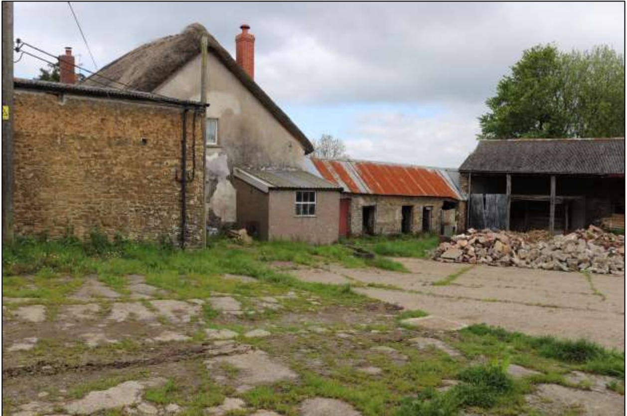
FIGURE 10: THE EAST GABLE END OF HOUSE; VIEWED FROM THE SOUTH-EAST.
