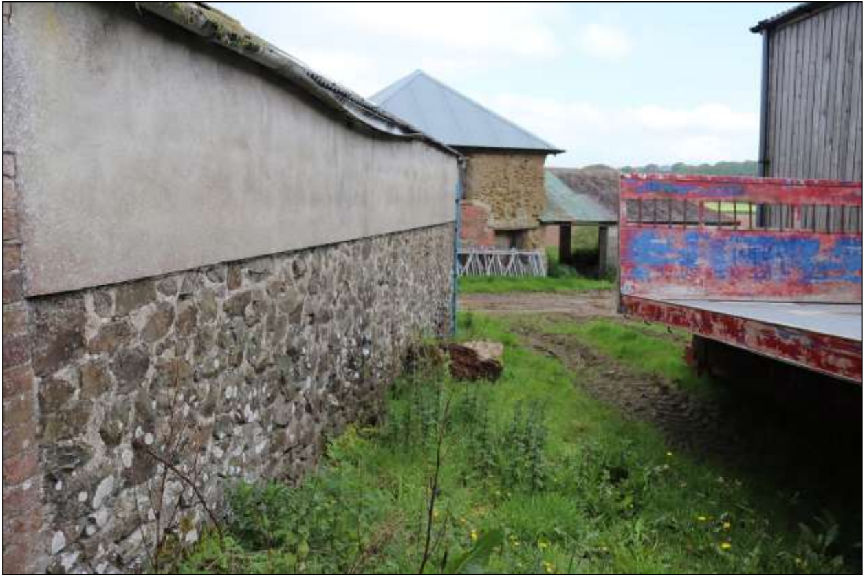
FIGURE 14: THE EAST (REAR) ELEVATION OF THE EXTENSION; VIEWED FROM THE SSE.
