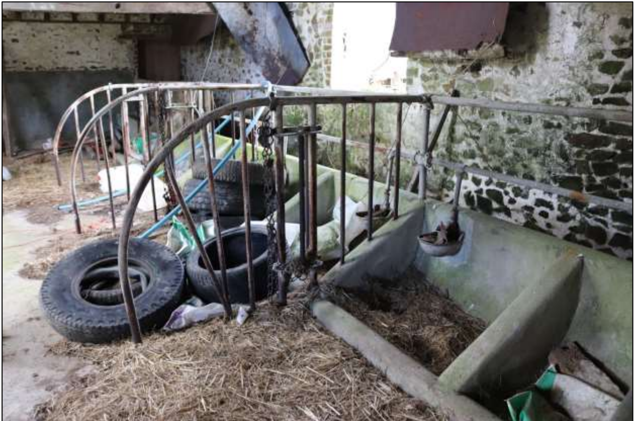
FIGURE 19: DETAIL OF THE STALLS AND FEED TROUGH; VIEWED FROM THE SOUTH-WEST.
