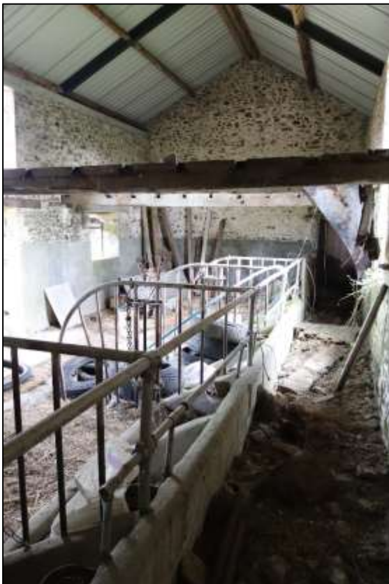
LEFT FIGURE 21: THE INTERIOR OF THE BARN; VIEWED FROM THE SOUTH-EAST.
