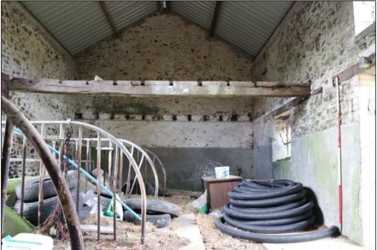
FIGURE 18: THE INTERIOR OF THE BARN; VIEWED FROM THE NORTH (SCALE 2M).
