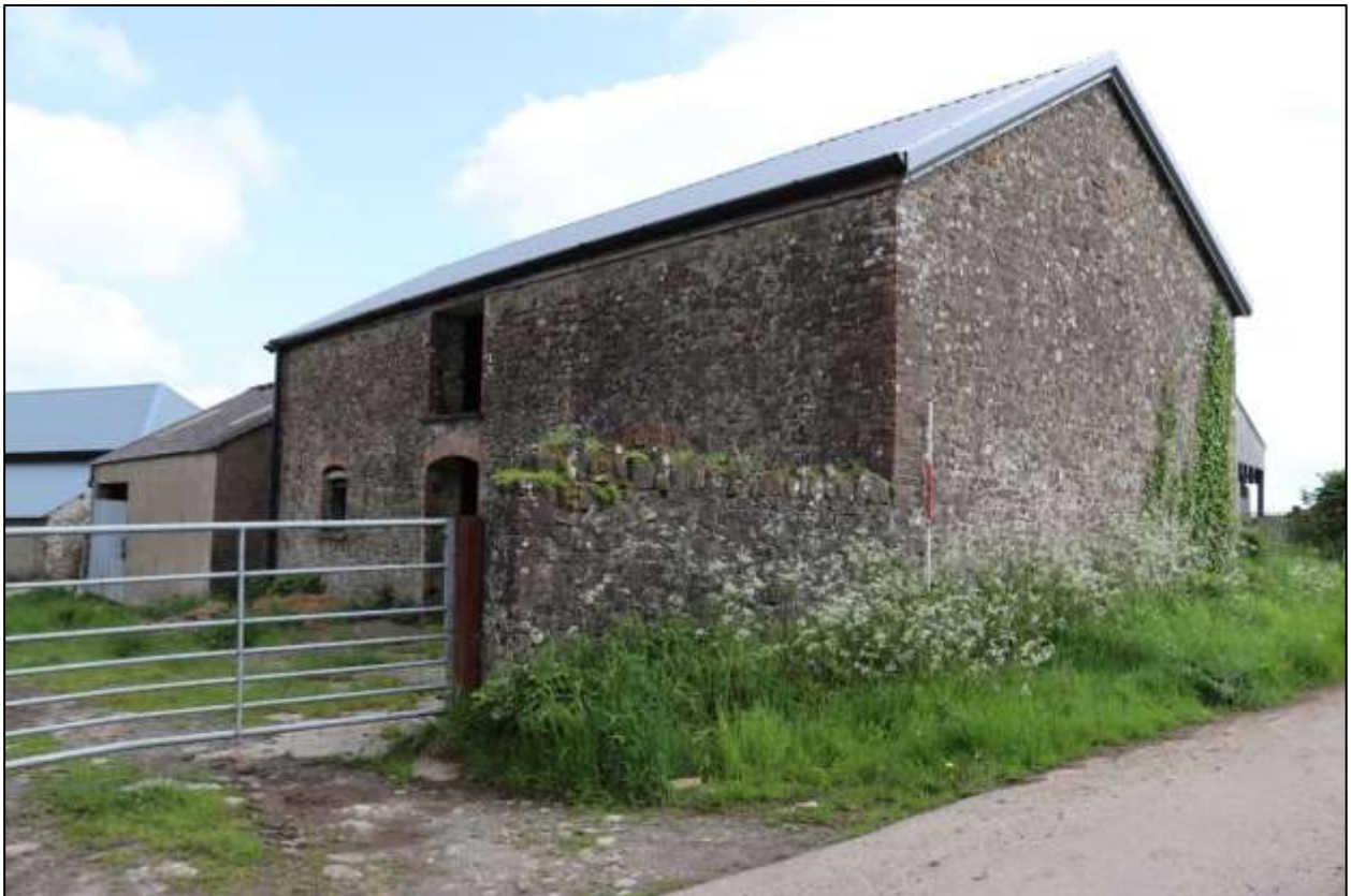
FIGURE 5: THE SOUTH ELEVATION OF THE BARN, BLIND AND SLIGHTLY ANGLED TO THE ROAD; VIEWED FROM THE SOUTH-WEST (SCALE 2M).
