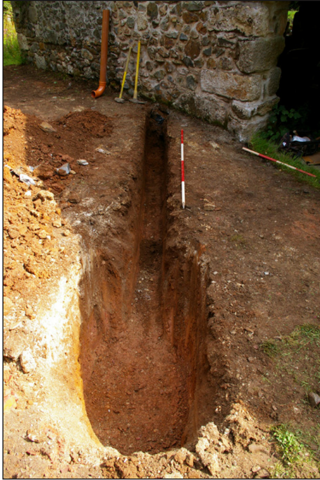
Figure 3: The pipe trench, viewed from the south (2m scale).
