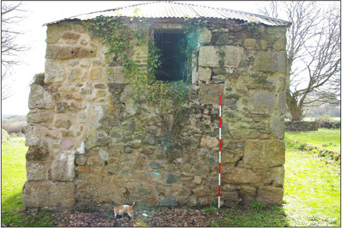
Figure 12: The north elevation, viewed from the north.
