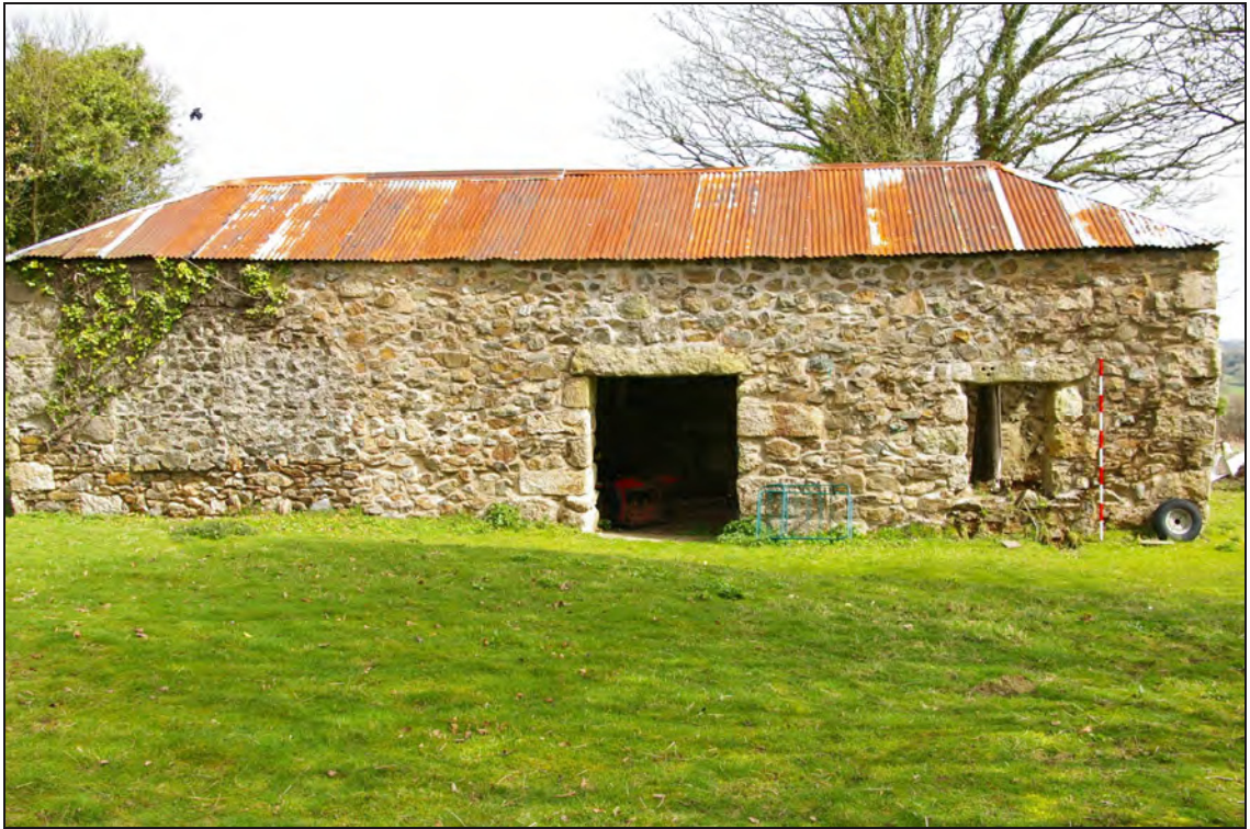
Figure 10: The west elevation of the building, viewed from the west.
