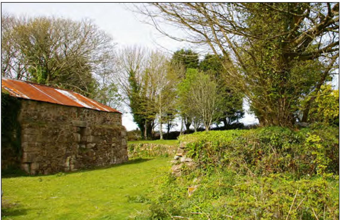
Figure 5: The former engine house, viewed from the south-east.
