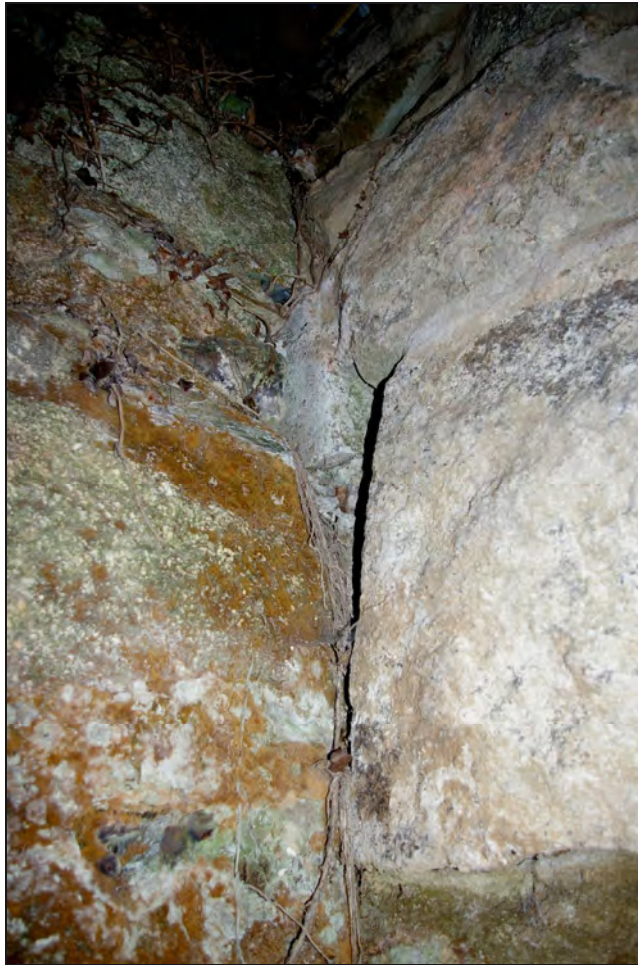
Figure 16: A cement block visible within the construction of the north-eastern corner of the building
