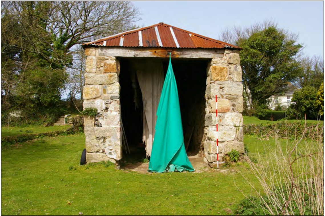
Figure: 8 The south elevation of the building, viewed from the south.
