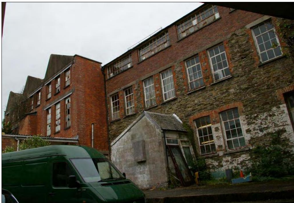
Figure 8: The west elevations of the east and north wings of the factory from under the entrance archway, viewed from the south-west.
