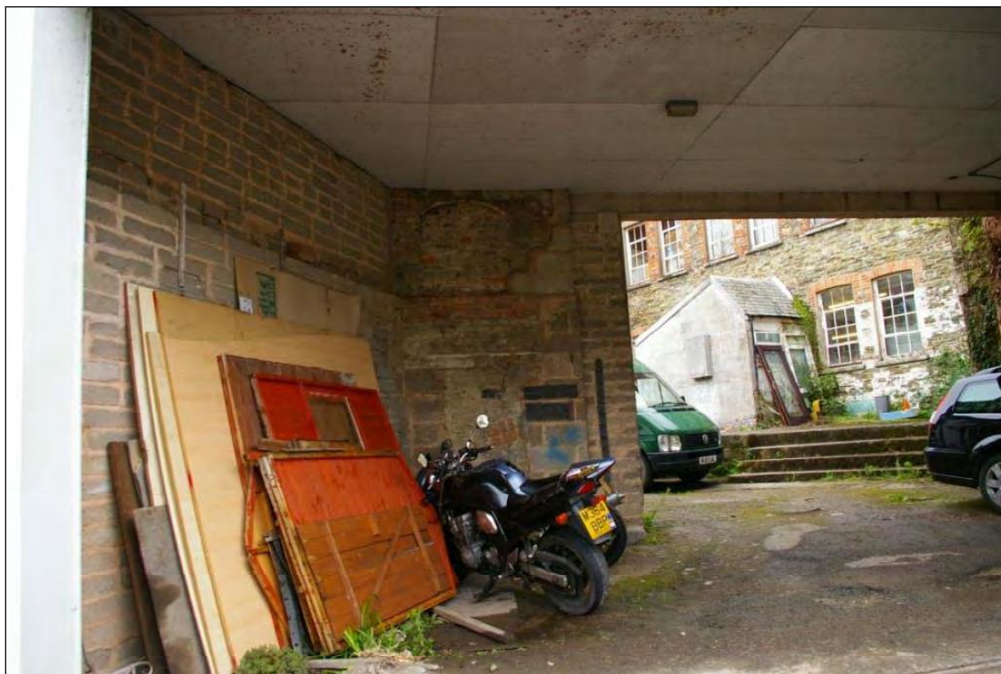
Figure 10: The west wall of the building containing the entrance archway, showing various phases of fireplace and the enclosed yard beyond, viewed from the south-west.
