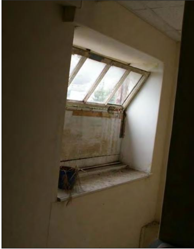
Figure 16: The narrow window in the kitchenette area, viewed from the south-east.
