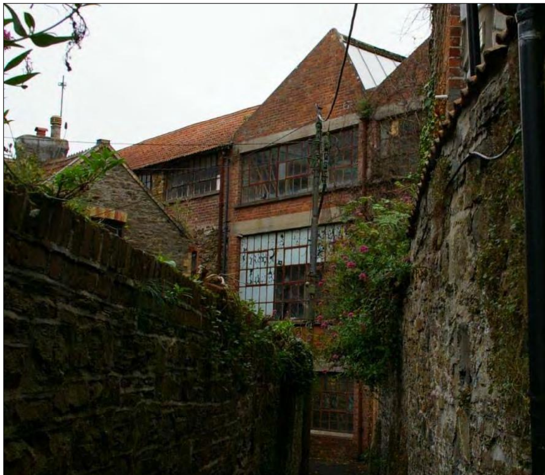
Figure 24: View down Ladywell Lane to the modern brick east elevation of the north wing of the factory, with large glass panels and triple pitched roof with skylights, viewed from the north-east.
