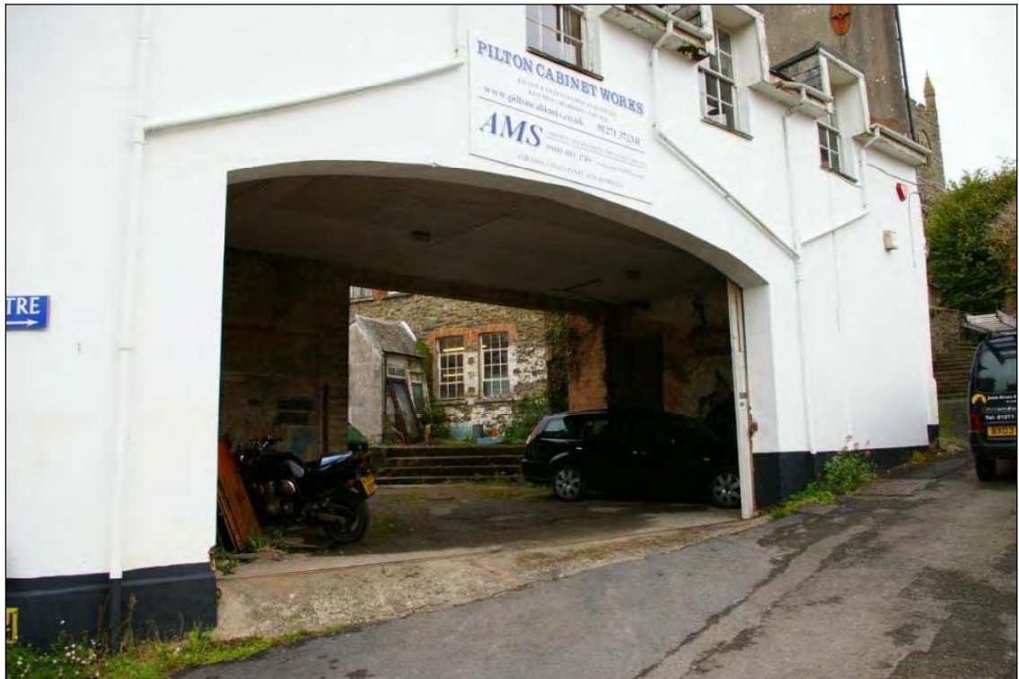
Figure 9: The entrance archway from Ladywell Lane to the factory complex with view into the enclosed yard, viewed from the south-west.
