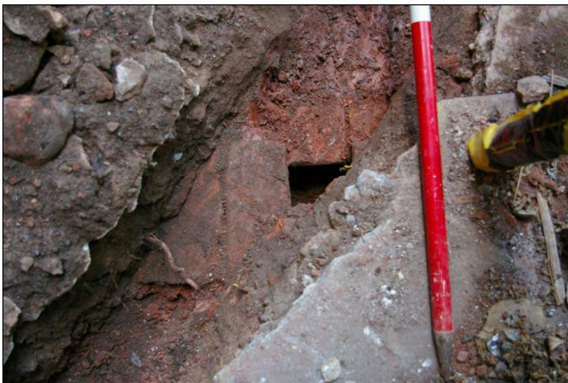
Figure 14: The brick capped drain exposed in Trench 1, viewed from the north-east (2m scale).
