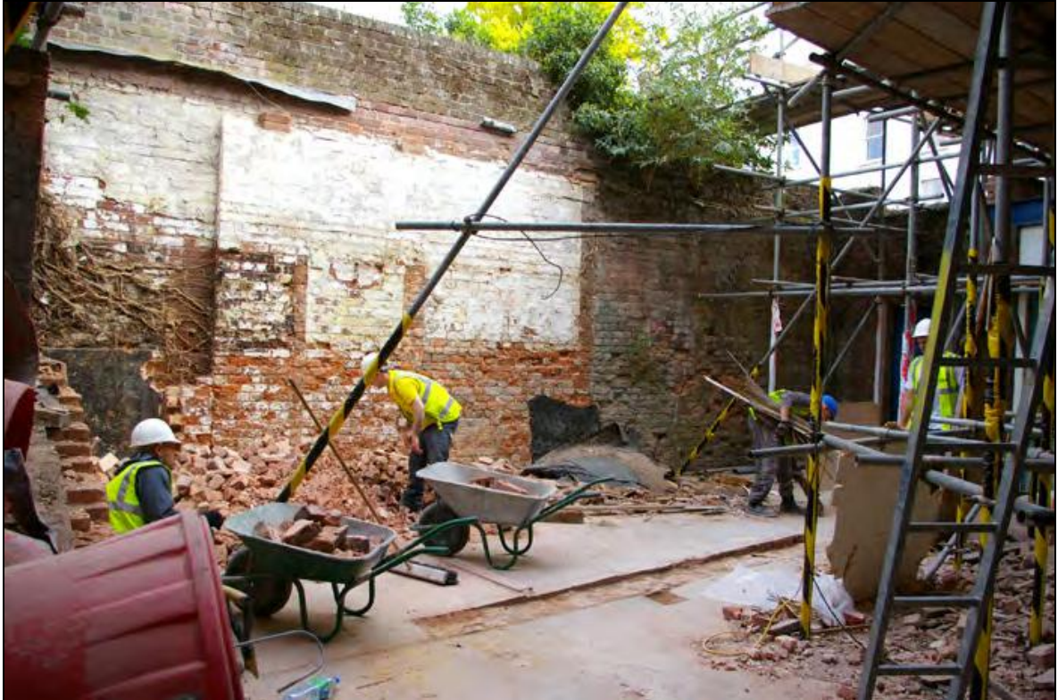
Figure 5: View into the Yard/Office/Toilet area during demolition, viewed from the south-east.
