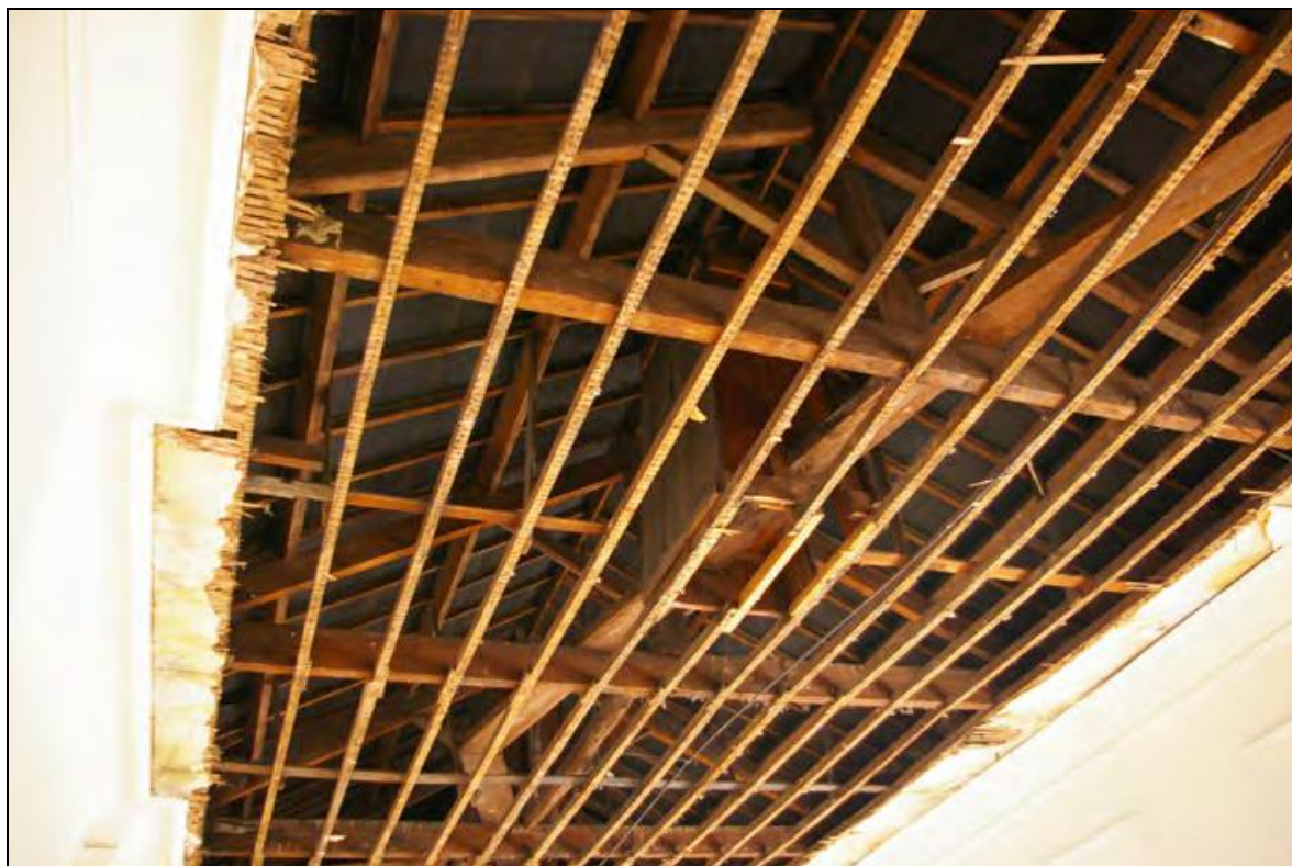
Figure 7: View to where the plaster ceiling has been removed, exposing rafters and leaving lathes to the edges, viewed from the east end of the room.
