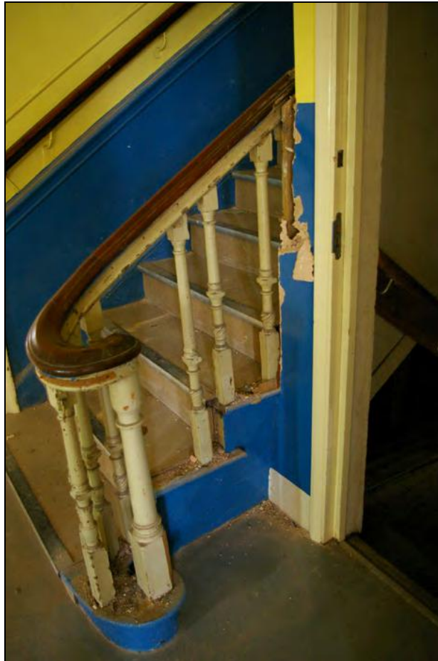
Figure 4: View of the base of the stair with curtail step.
