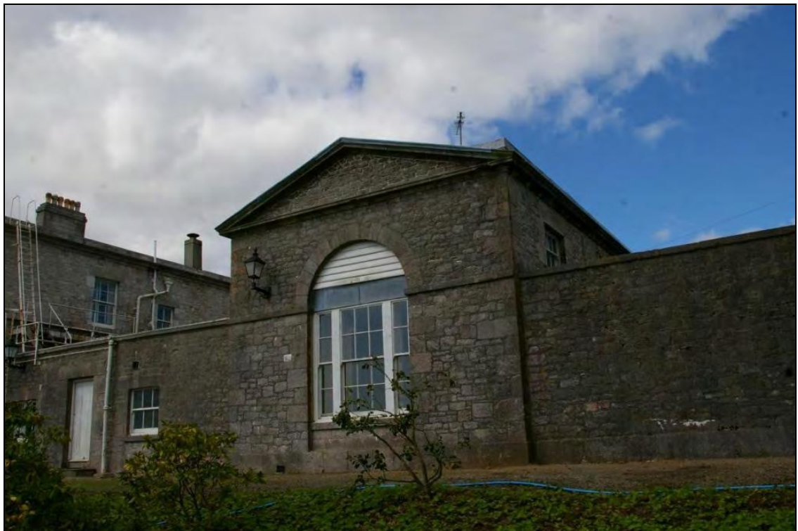
Figure 12: The south elevation of the East Pavilion, viewed from the south-east.
