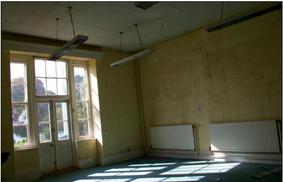
Figure 15: The south wall of the former kitchen, viewed from the north-east.
