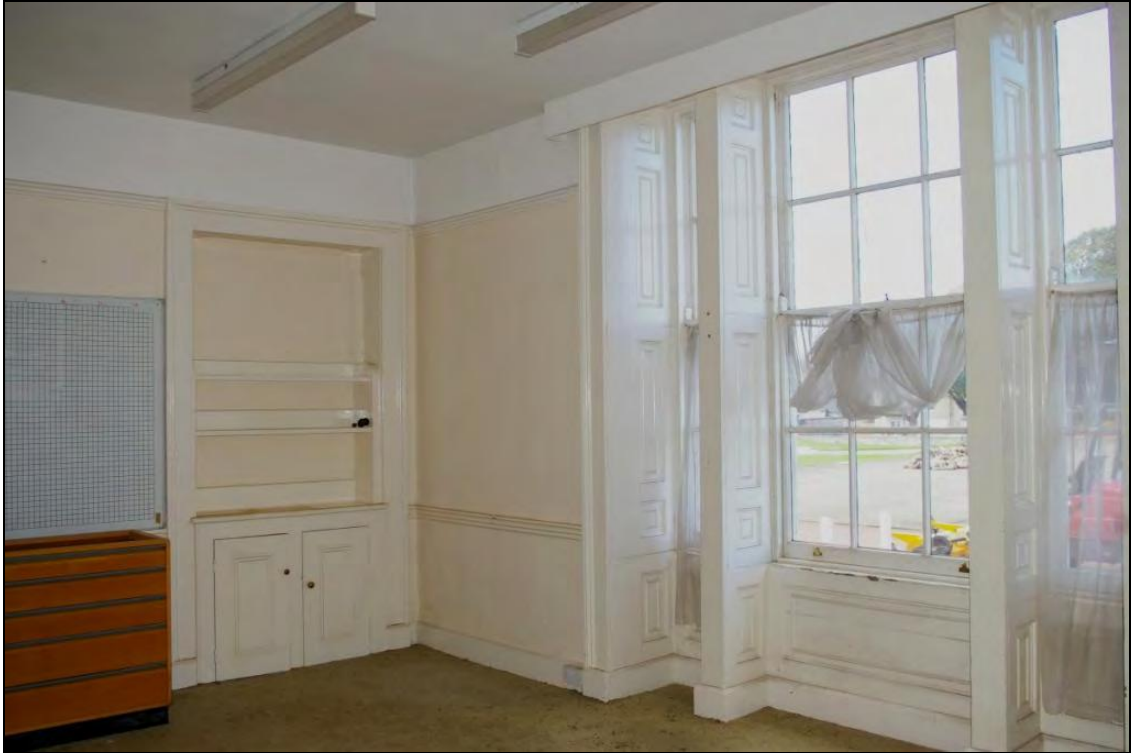
Figure 23: The north and west walls of the north cottage, showing three light central window in the north wall and the possible blocked door or window in the west wall, from the south-east.
