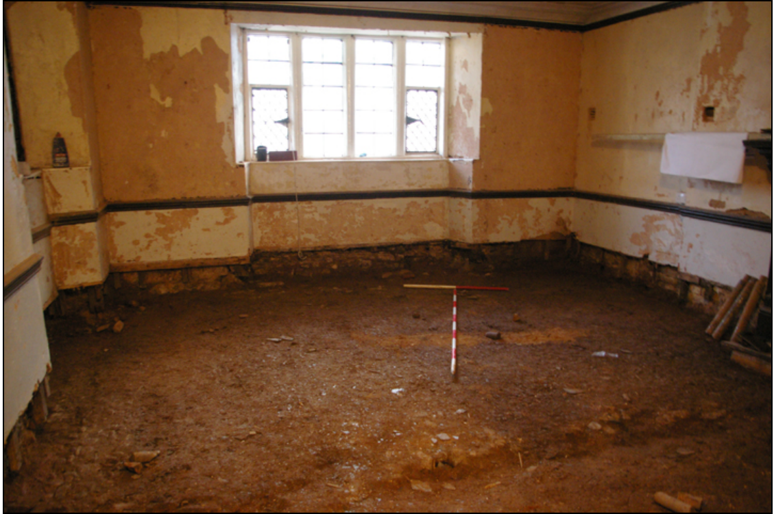
Figure 24: Room 5 post floor reduction, showing cobbled surface, viewed from north-west (1 & 2m scale).
