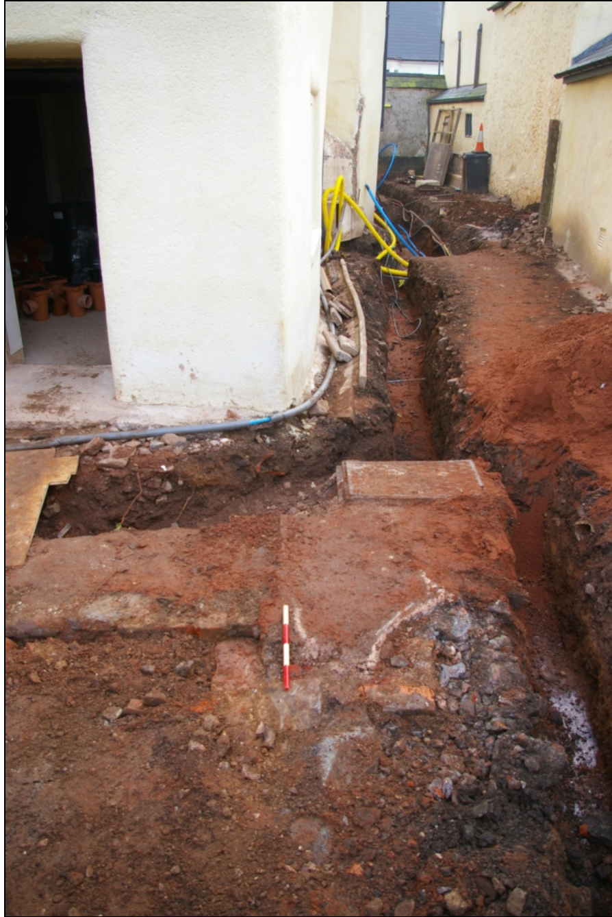
Figure 10: Southeast corner of the wall footing, following the partial removal of the concrete floor, viewed from west (0.4m scale).
