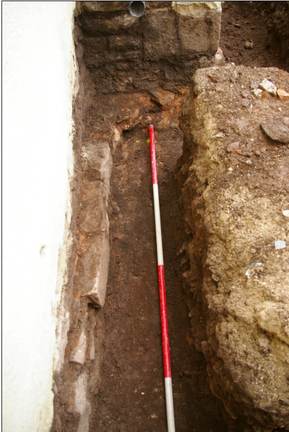
Figure 15: Shot of the footings the main hall (Room 3) and projecting stack, viewed from north (2m scale).
