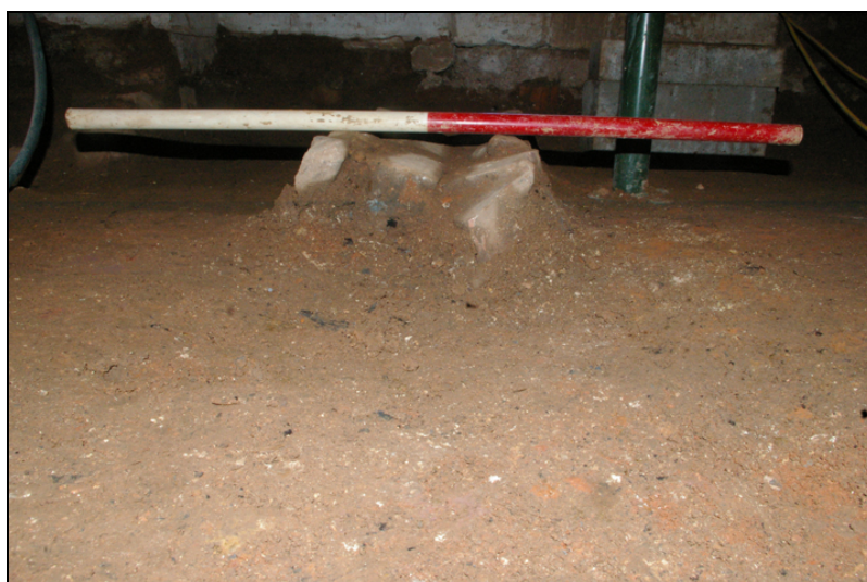
Figure 22: Room 4, Drain {215}, viewed from east (1m scale).
