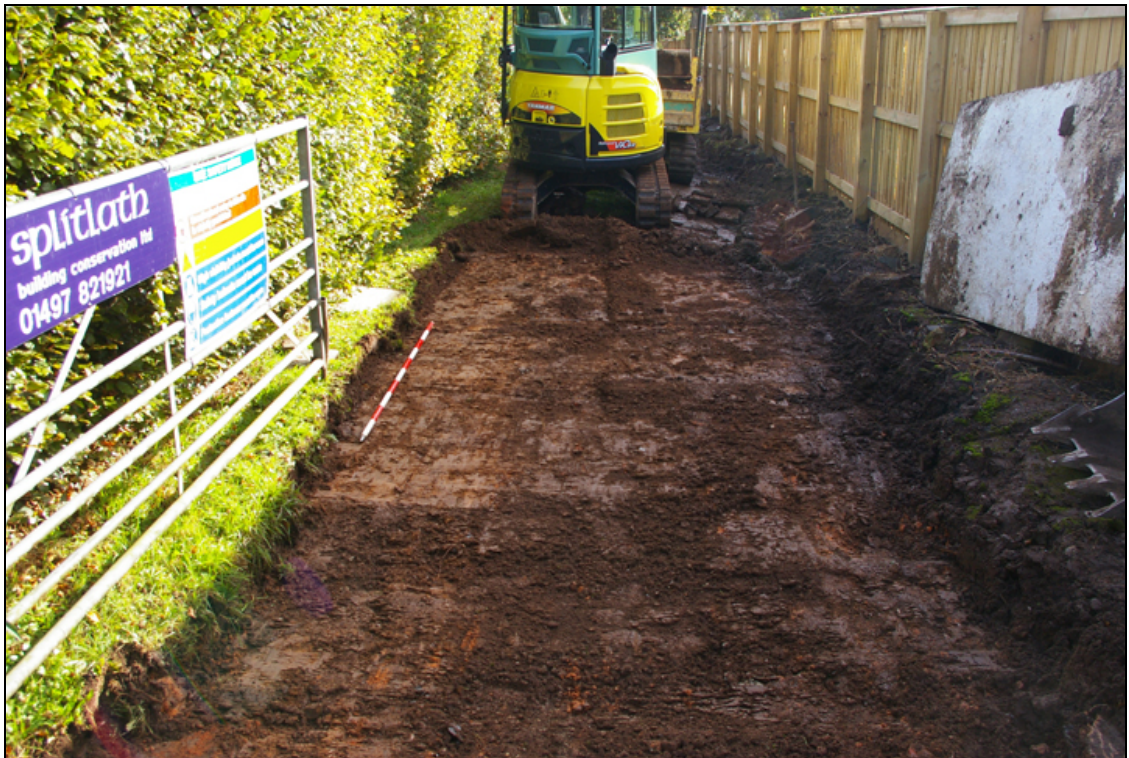
Figure 5: Driveway, post-excavation, viewed from west (2m scale).
