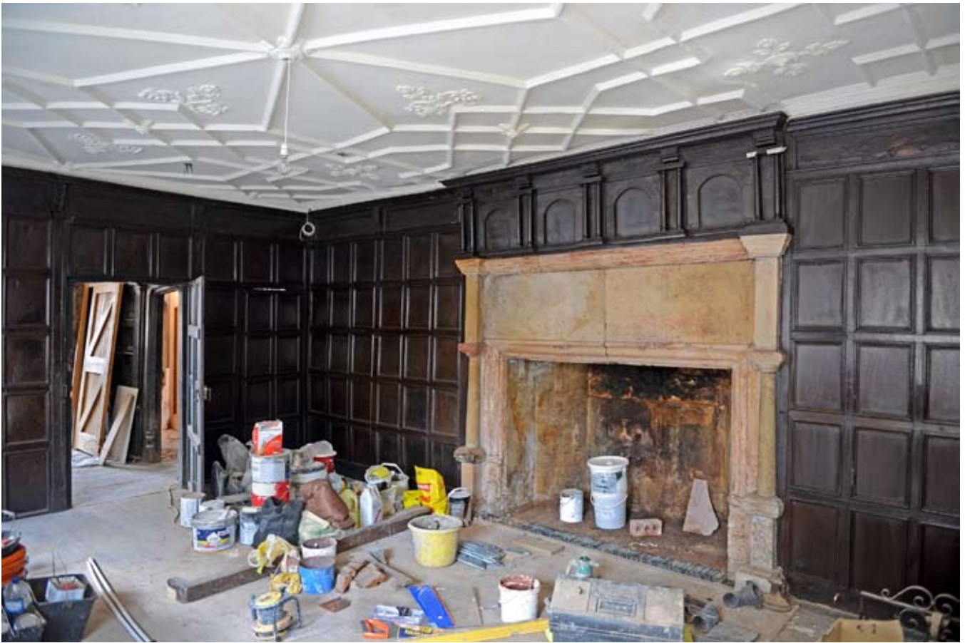
The parlour looking northwest, 12.03.2014.
