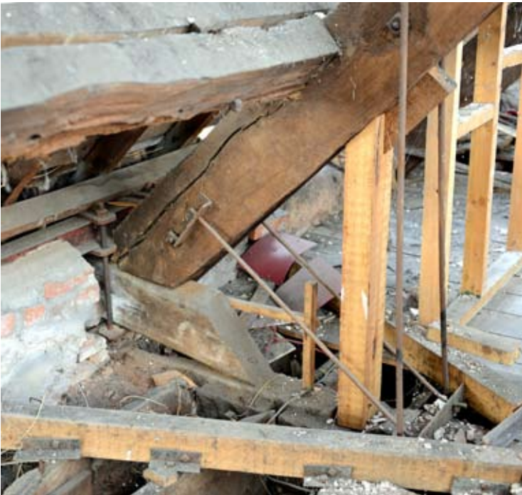
Detail of the west end of the same trusses showing the repairs of 1890-1, 17.10.2012.
