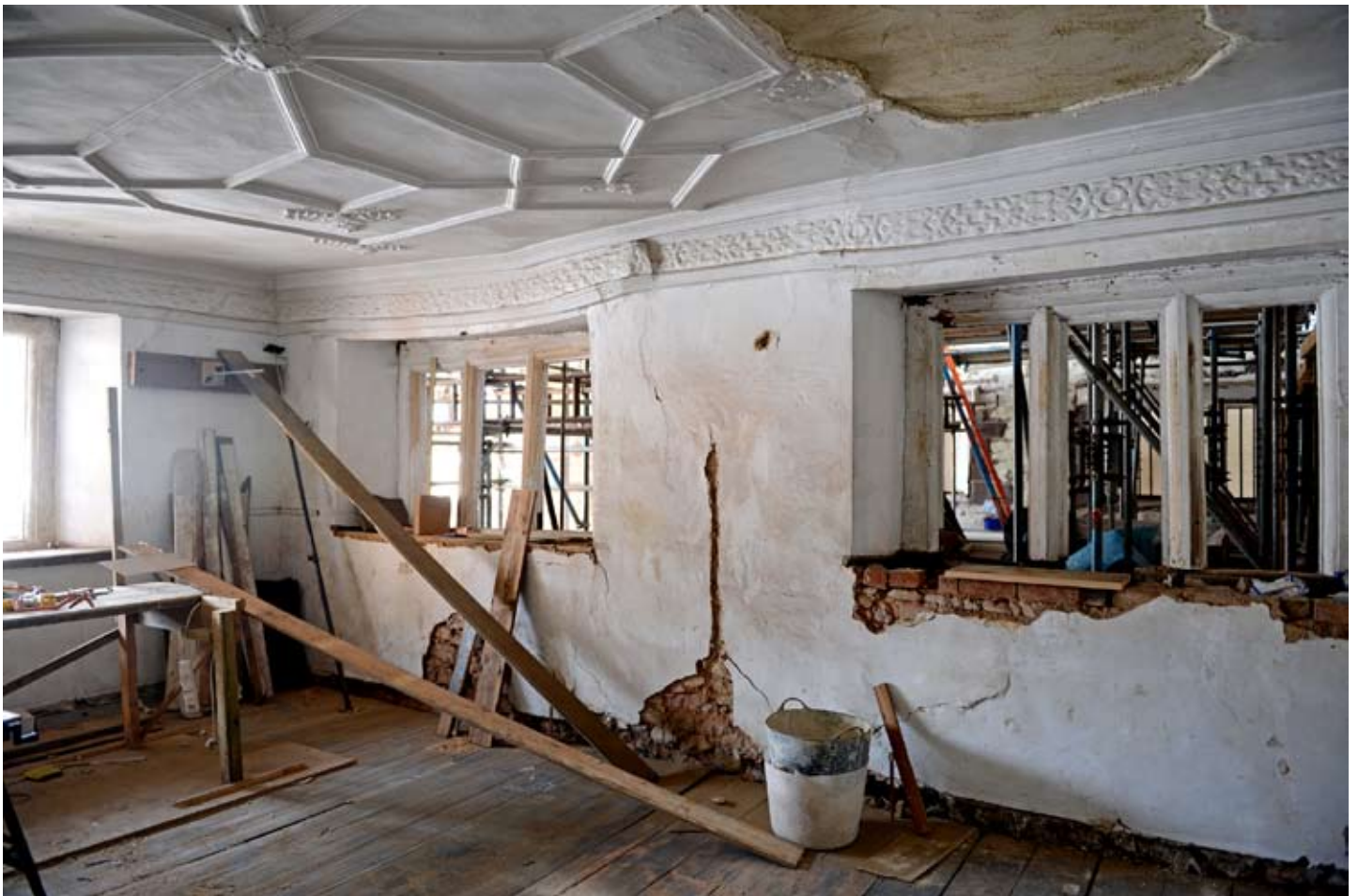
The south wall during repairs, 18.06.2013.
