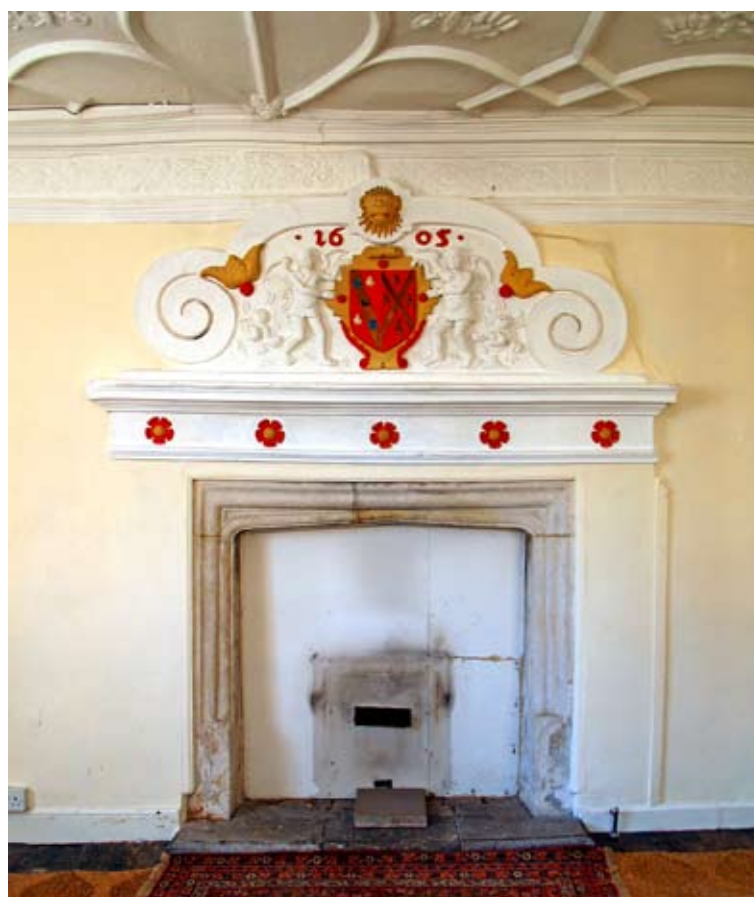
The fireplace and plaster overmantle in the Great Chamber; 02.06.2009.
