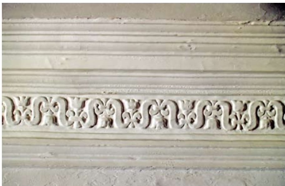
Detail of the plaster cornice, 02.06,2009
