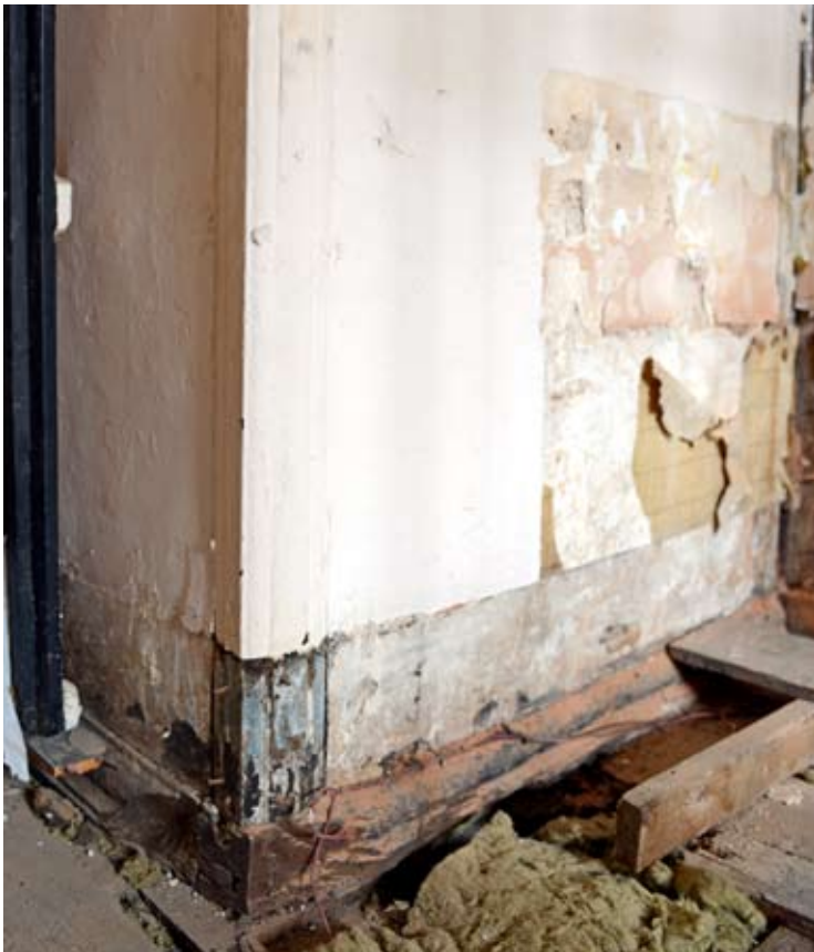
The east wall of the kitchen chamber backs onto the Great Chamber. It is close studded with rod-and-daub infill and clad with lath and plaster. Notice the chiselled assembly marks in the sill and the early 18th century painted black skirt to right, 18.06.2013.
