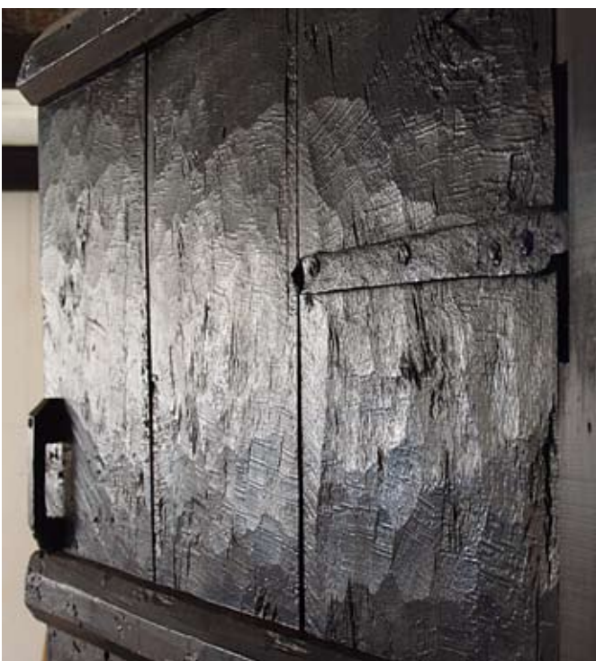
Detail of the back of G.D. 12D showing the adze marks, 09.06.2009.
