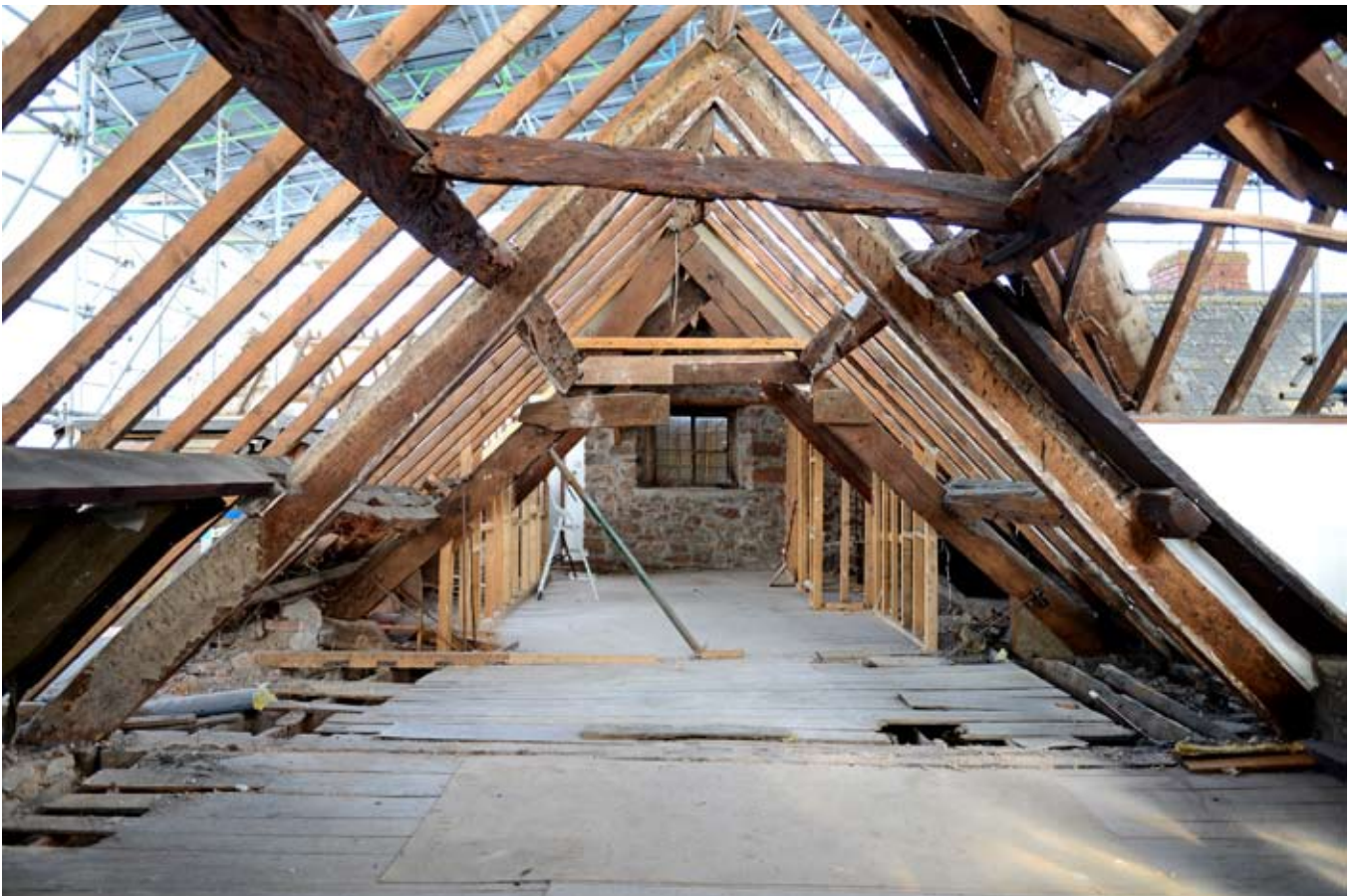
The main block roof looking north, 17.10.2012.
