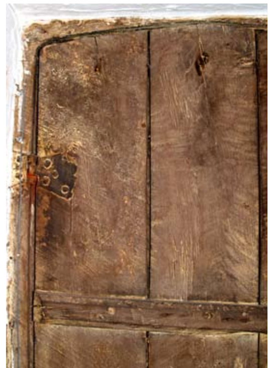
The corridor side of the doorway into the parlour; 06.11.2009.
