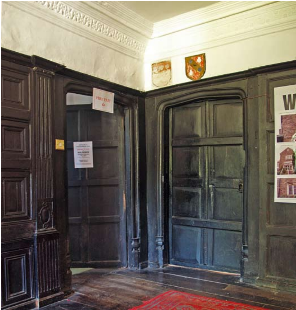
The doorways in the northeast corner of the Hall, 02.06.2009.
