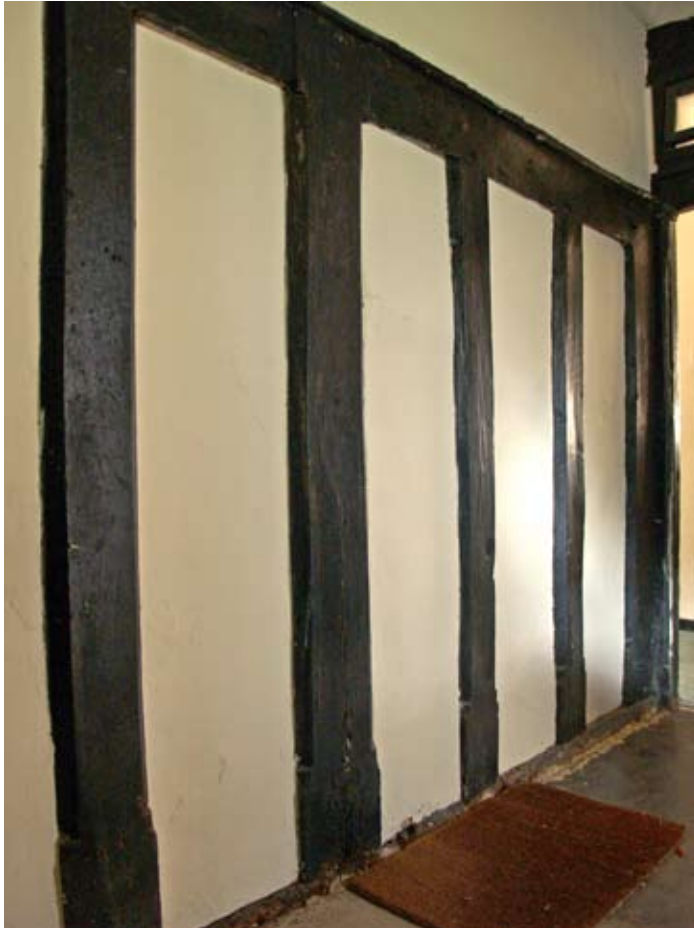
Detail showing that the centre stud rises through the headbeam and is chamfered above. This suggests that the upper part was also panelled originally, 06.11.2009.
