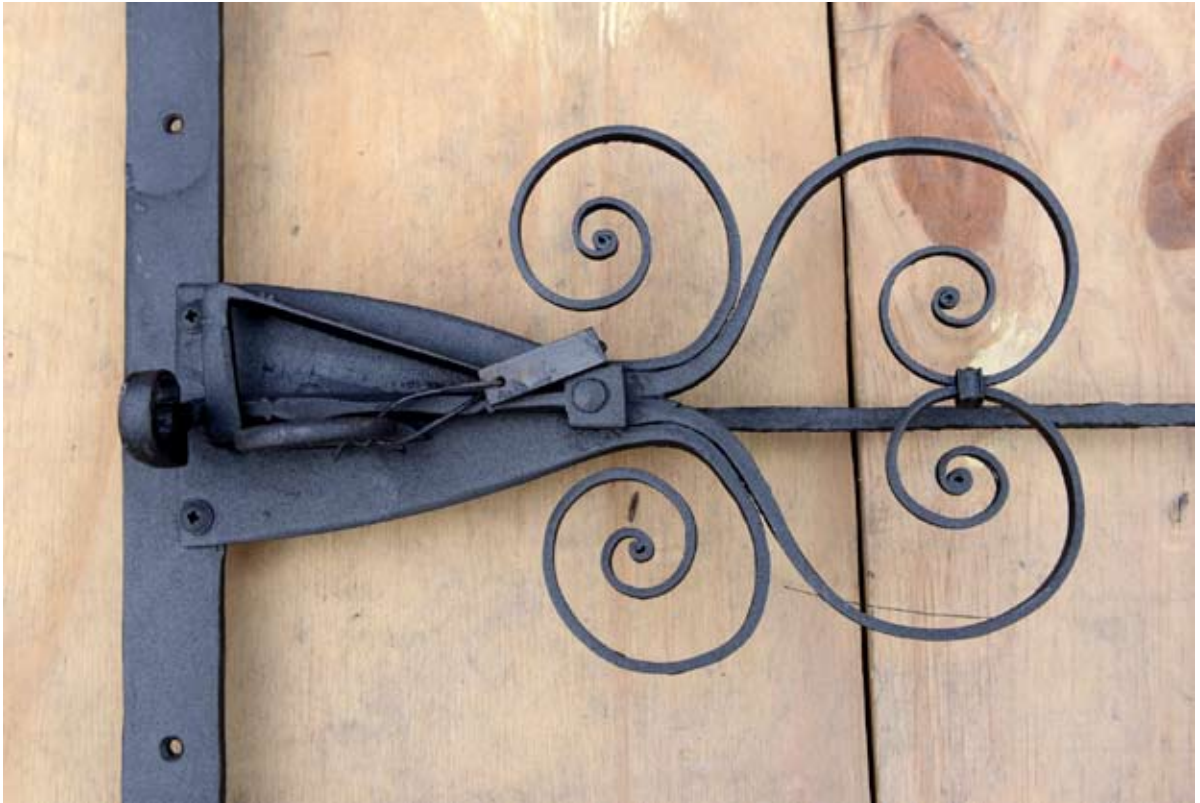
Detail of the inside of the catch on the inside of the central 1890-91 casement in W.G. 07, serving the parlour, with replacement screw fittings. Photographed during repairs and conservation at Brockweir, 20.05.2013.
