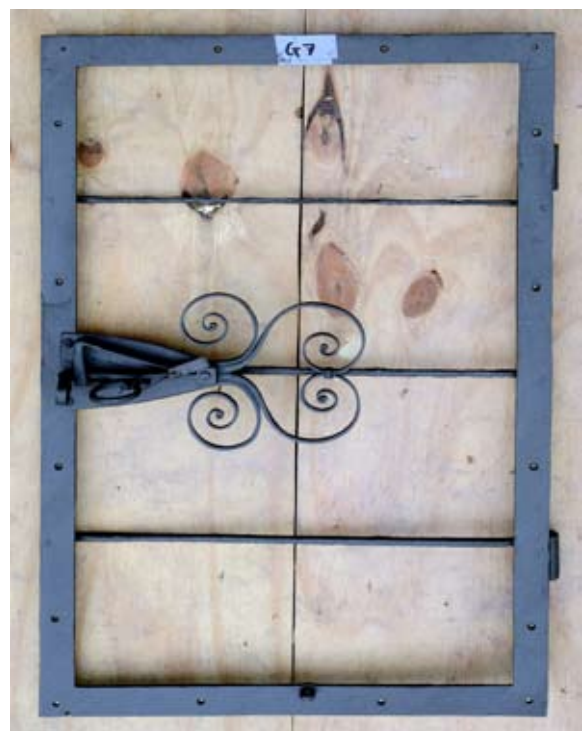
The inside of the central 1890-91 casement in W.G. 07 during repairs, 20.05.2013.
