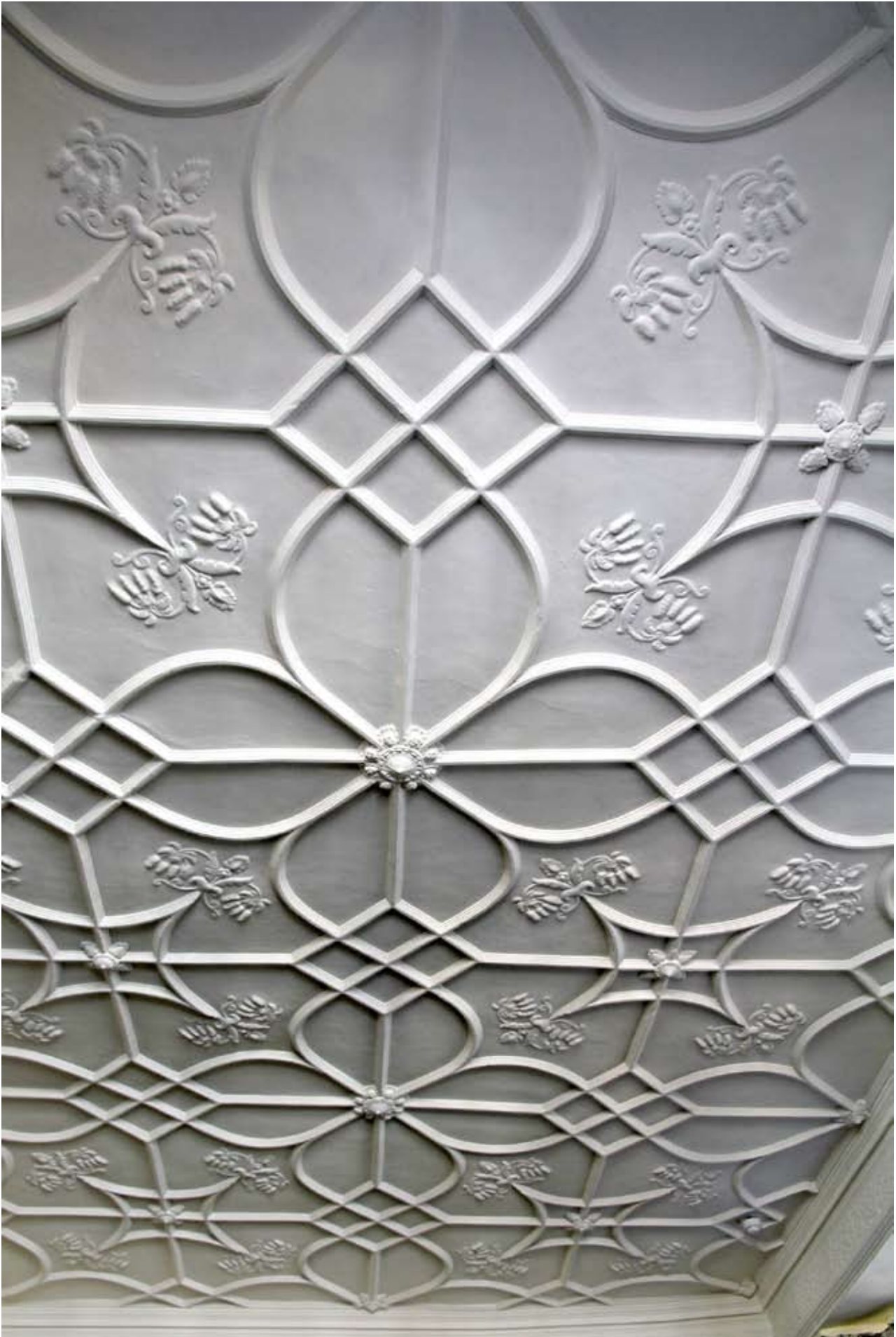
The ceiling of the Great Chamber, restored and cleaned, 18.06.2014.
