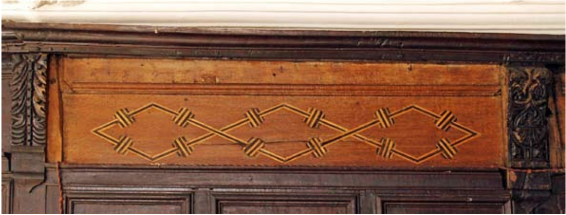
Detail of one of the marquetry inlay panels that was cleaned up in the late 20th century, 02.06.2009. It was varnished over in 2012-13.
