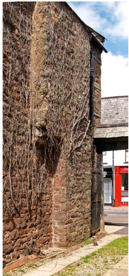
The two-phase chimneystack on the south side of the southern front wing, 09.06.2009.
