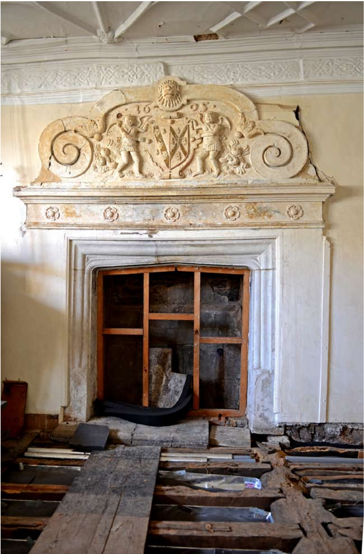
The fireplace and plaster overmantle in the Great Chamber undergoing repairs, 30.01.2013.
