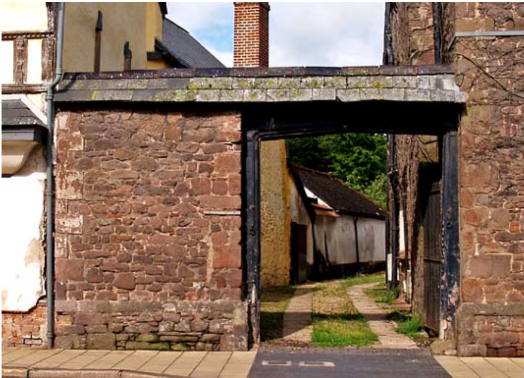
The front of the gateway and boundary wall, 03.07.2009.
