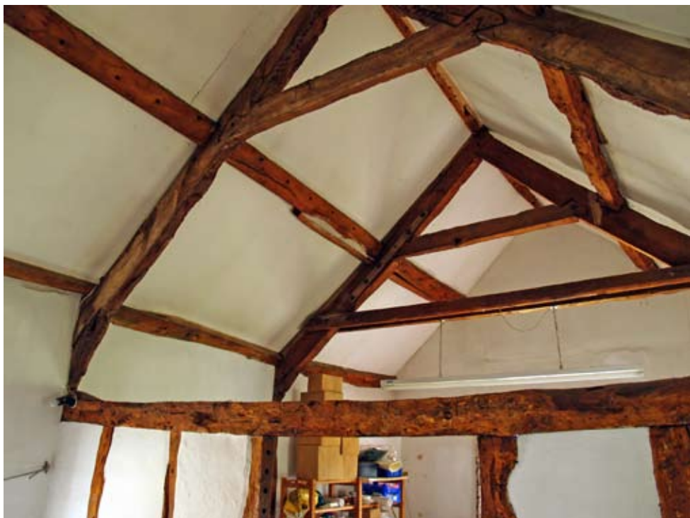
The roof of the rear block from the east showing the top of the close-studded partition, 09.06.2009.
