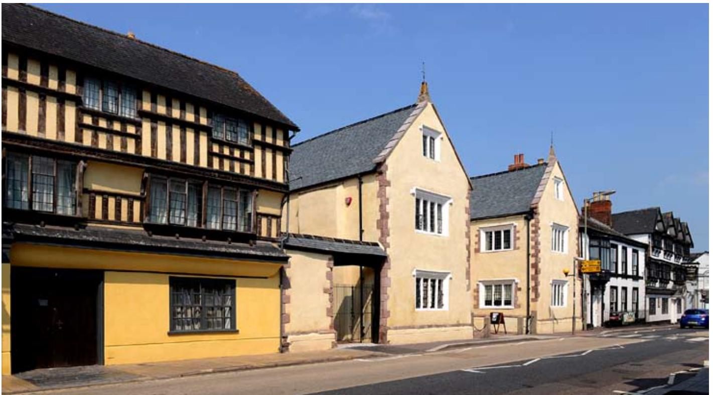
The west side of Fore Street on 24.07.2014 following the repairs to the Walronds looking north with the Merchant's house left and Manor House next door but one to right.
