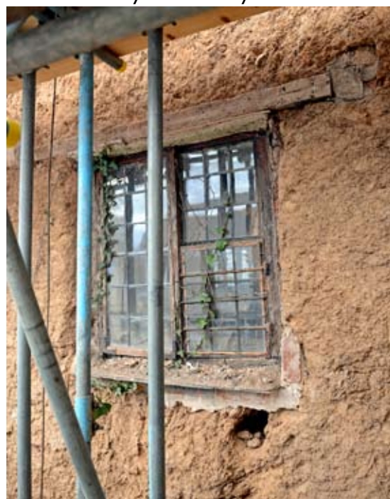
The first floor window, W.F. 20, on the south side on 29.10.12
