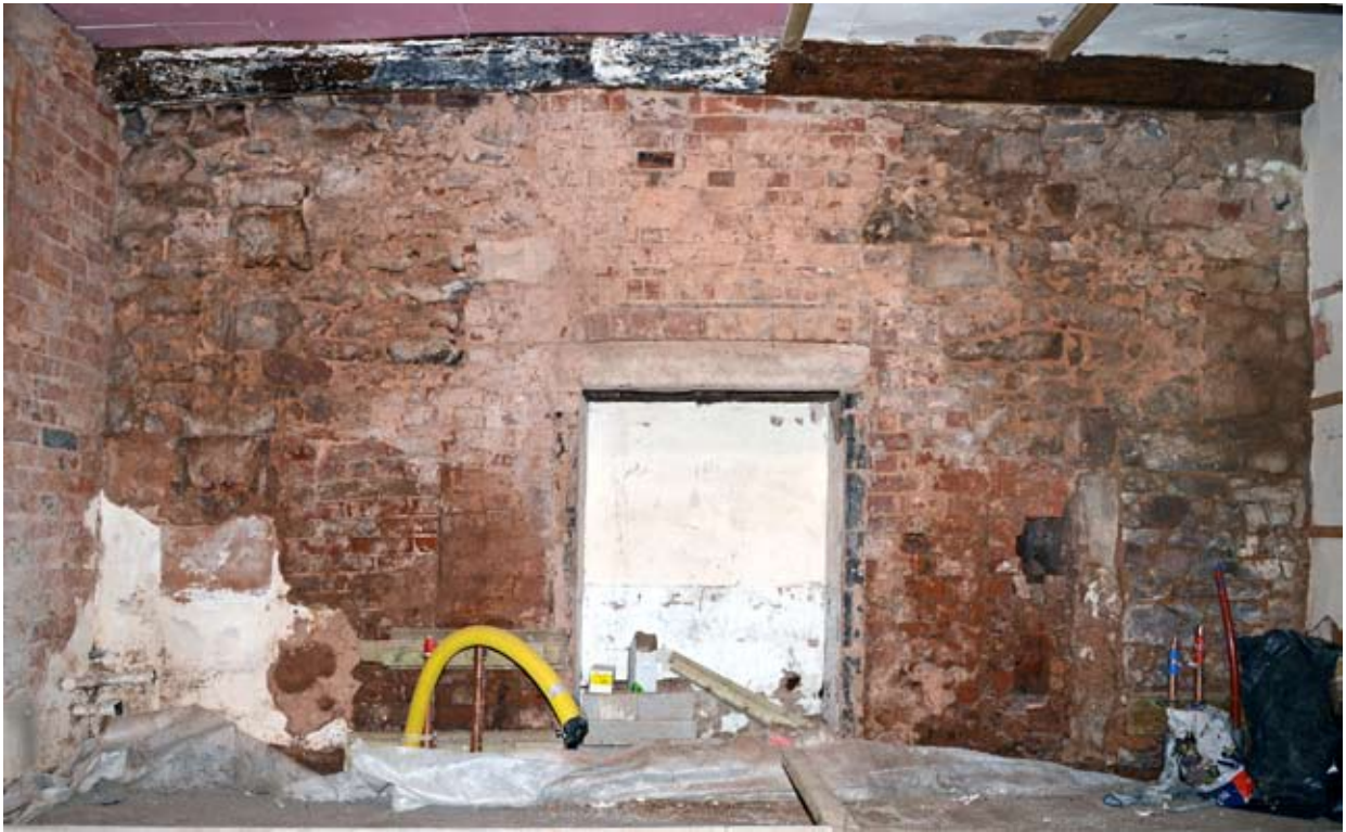
The west wall and remains of a sequence of kitchen fireplaces, 30.01.2013.
