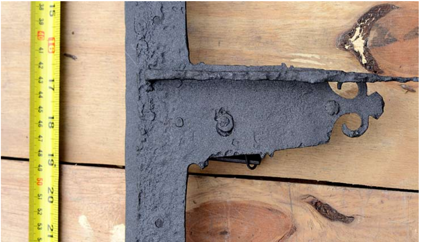
Detail of the backplate and catch of the northern casement of the east-facing first floor window W.F.08 from outside (above) and inside (below). Uniquely at the Walronds before 1890-91 the backplate is welded to the frame and maybe re-used from fragments recovered from the burnt out remains of the the 16th century house. The catch may date from c1605. The photographs were taken during repair and conservation work at Brockweir, 20.05.2013.
