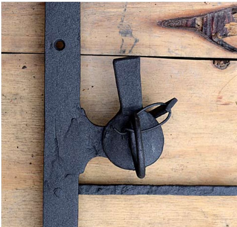
The southern casement of the east-facing first floor window w.F.08 is a typical Burrow wrought-iron casement from 1890-1. Both photographs show the inside of the casement with the whole casement above and a detail of the turnbuckle catch below, which is welded rather than rivetted to its inner frame. The photographs were taken during repair and conservation work at Brockweir, 20.05.2013.
