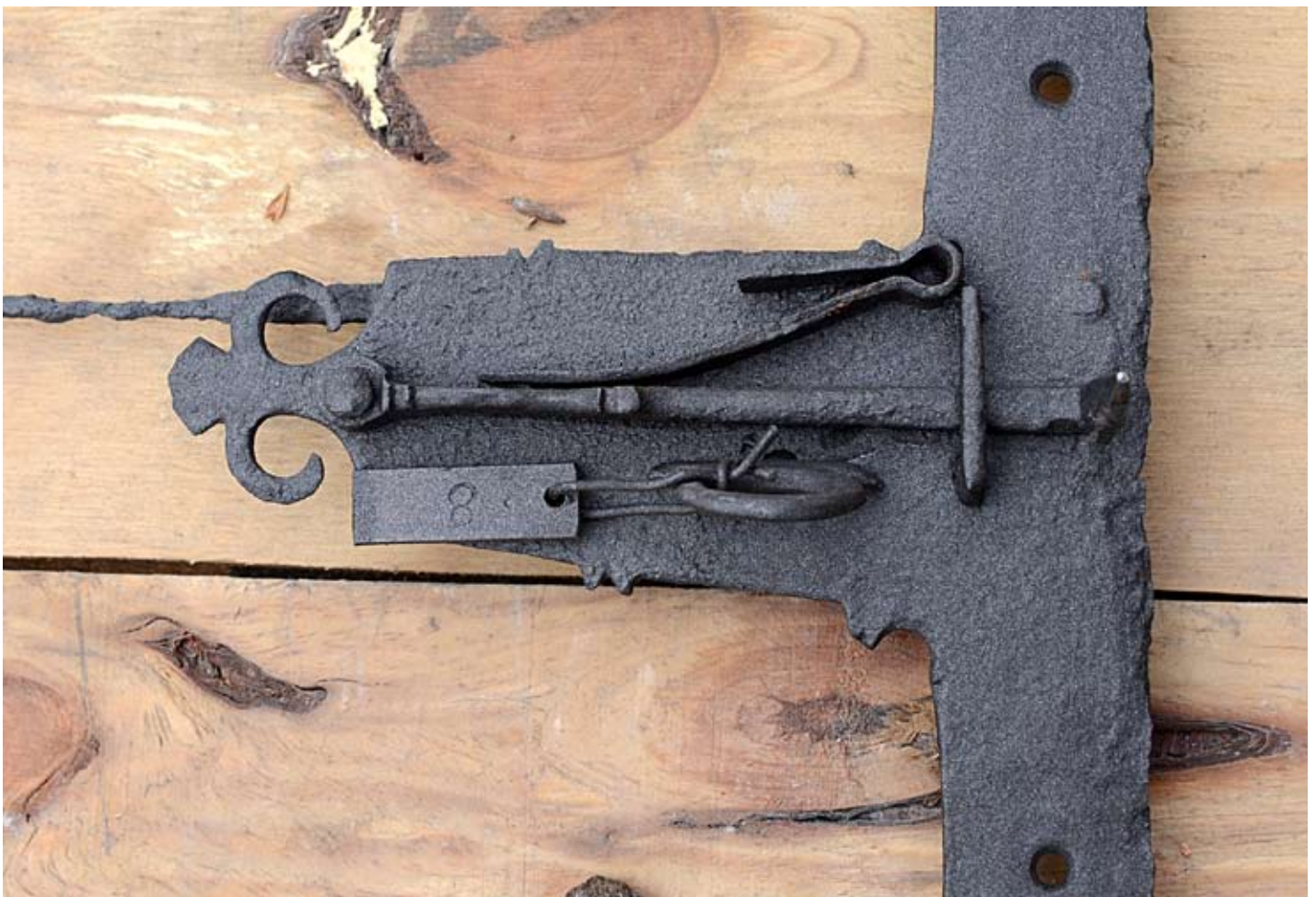
Detail of the backplate and catch of the northern casement of the east-facing first floor window W.F.08 from outside (above) and inside (below). Uniquely at the Walronds before 1890-91 the backplate is welded to the frame and maybe re-used from fragments recovered from the burnt out remains of the the 16th century house. The catch may date from c1605. The photographs were taken during repair and conservation work at Brockweir, 20.05.2013.
