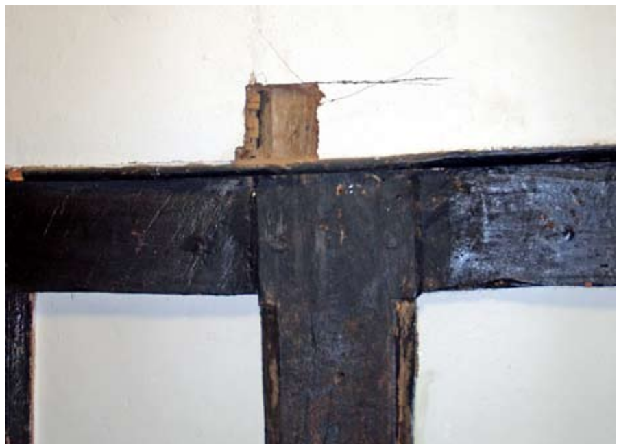
Detail showing that the centre stud rises through the headbeam and is chamfered above. This suggests that the upper part was also panelled originally, 06.11.2009.
