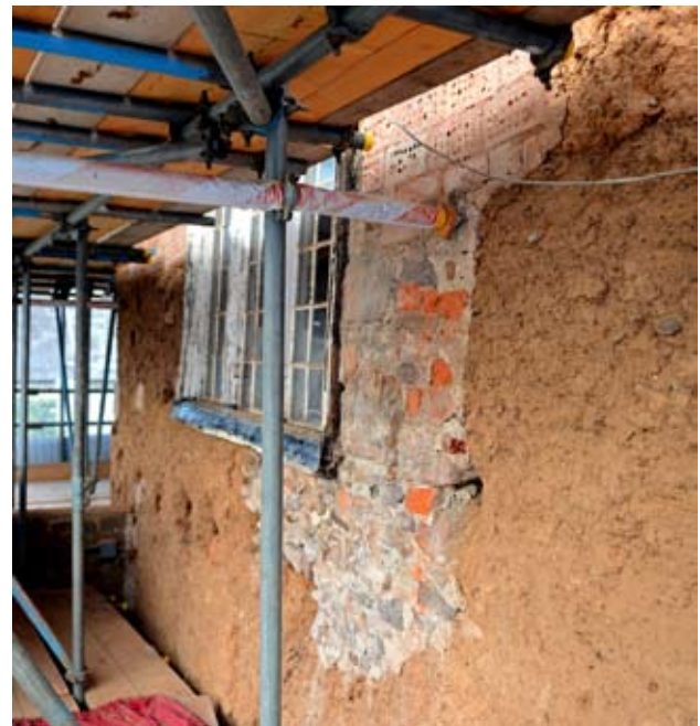
The probably c1970 brick repair to the gable in the west end above the first floor window, W.F. 19, 29.10.12.
