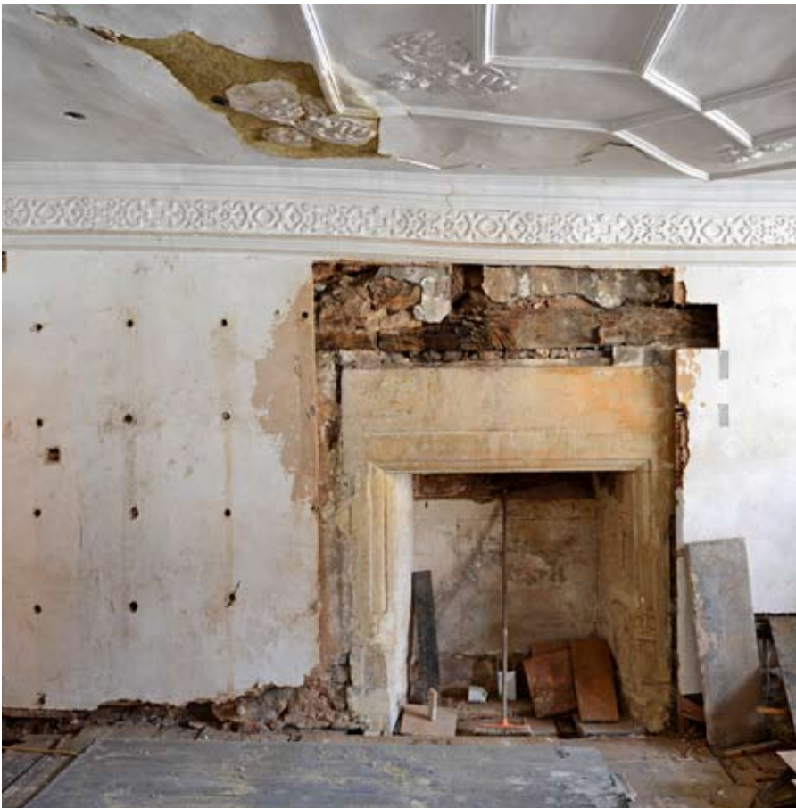
The northwest corner of the chamber with the floor joists exposed, 30.01.2013.
