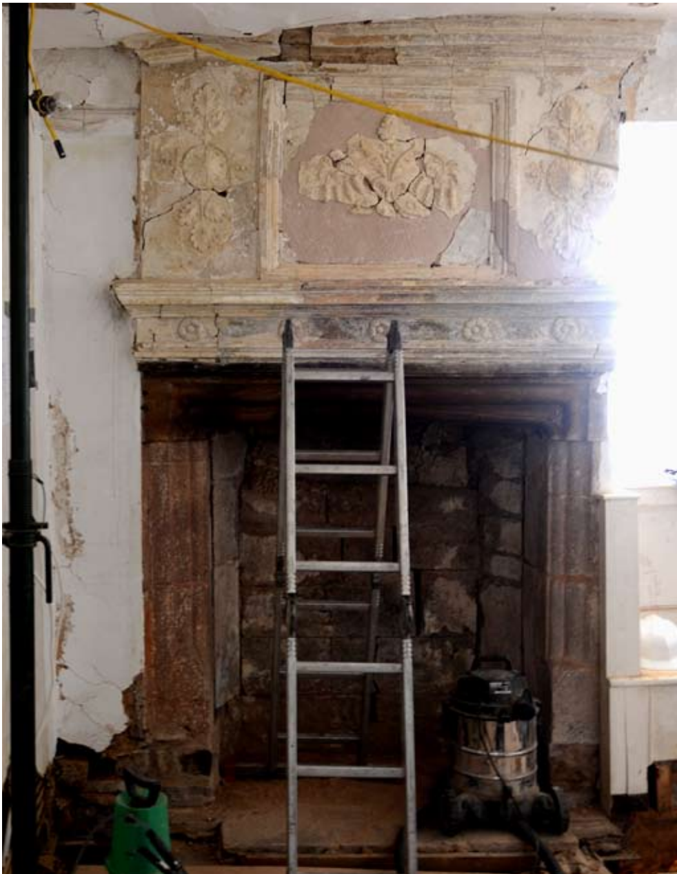
The fireplace and overmantle during repairs, 04.03.2013.
