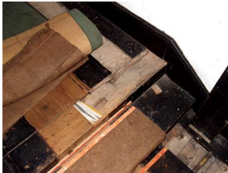
The sill of the close-studded crosswall, 06.10.2009.
