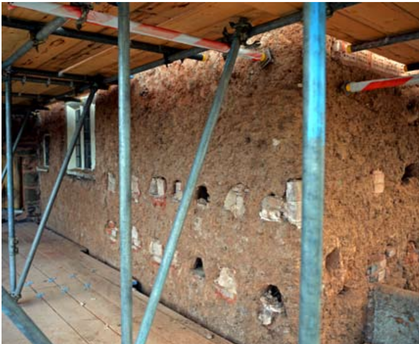
The blocked pigeon holes in the north wall and the chimney flue and blocked window in the south wall, both 29.10.12
