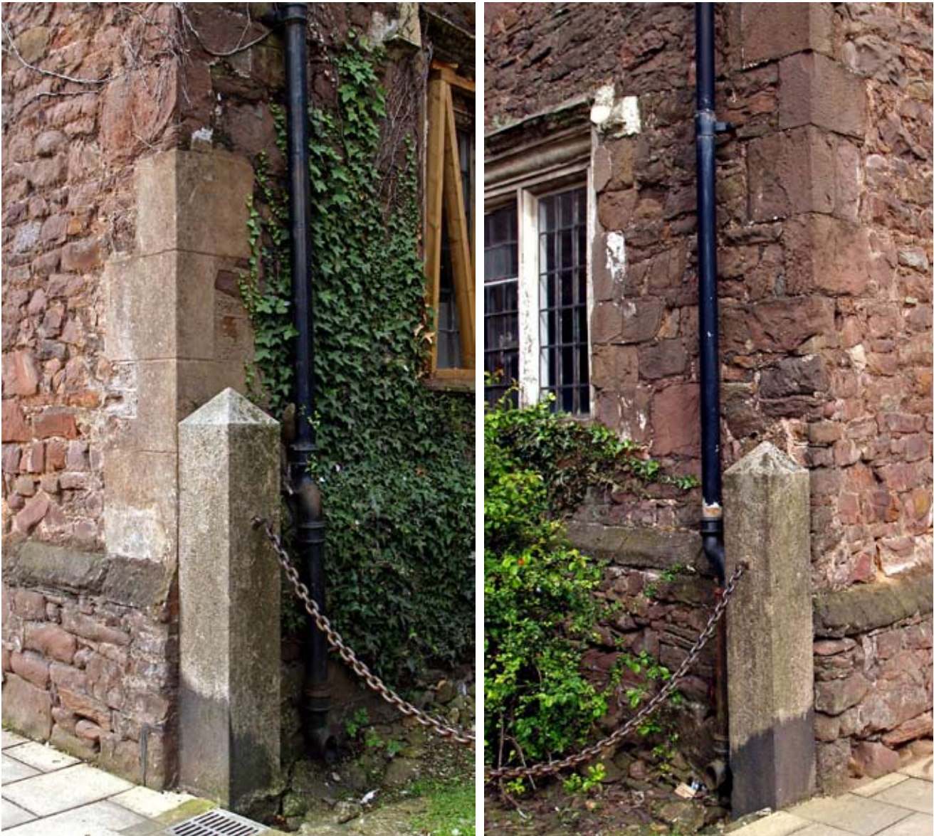
The proud quoins stop each side high enough to indicate the c1605 design of a front wall to the forecourt. The inner corners of the front wings are presented, north to left and south to right, both photographs from 06.08.2009.
