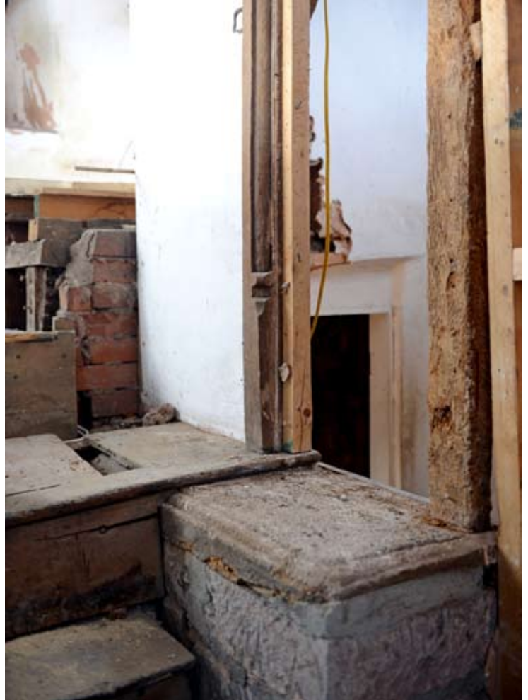
The moulded oak slab capping the stairwall and the surviving doorjamb to the tiny room over the main stair, 30.01.2013.
