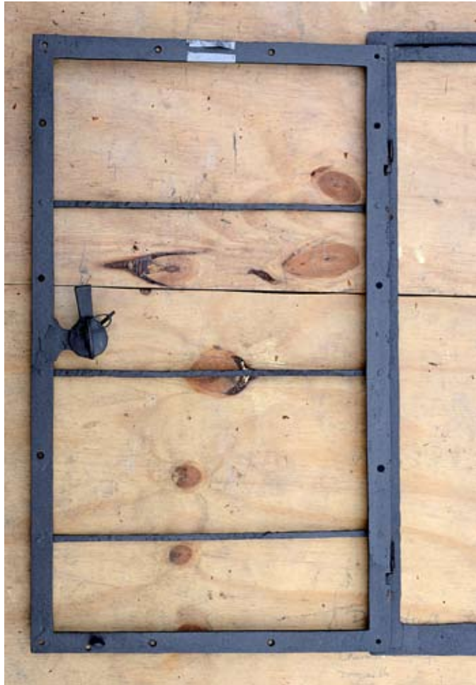
The southern casement of the east-facing first floor window w.F.08 is a typical Burrow wrought-iron casement from 1890-1. Both photographs show the inside of the casement with the whole casement above and a detail of the turnbuckle catch below, which is welded rather than rivetted to its inner frame. The photographs were taken during repair and conservation work at Brockweir, 20.05.2013.
