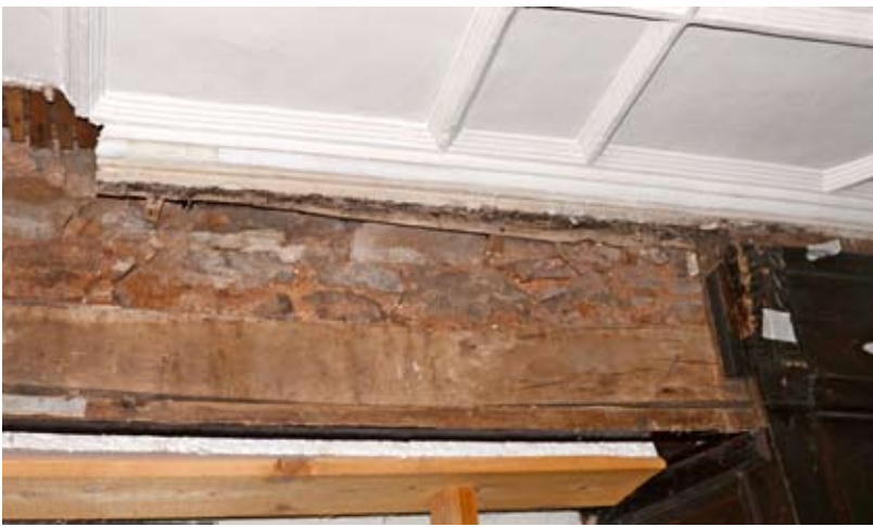
The ragged edge of the wall plaster at the east end of the south wall ( over WG. 07) seems to indicate an original plastered wall which was cut out when the panelling was installed, 30.01.2013.
