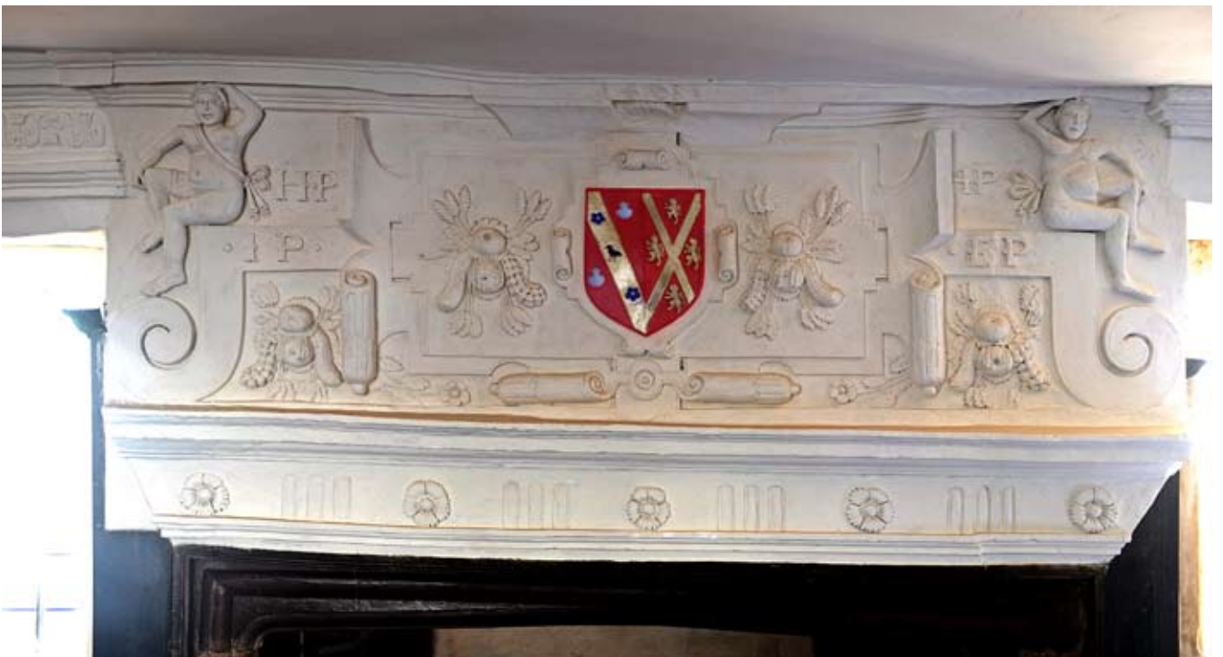
The ornamental plasterwork overmantel before repair, 01.07.2009, during repair, 18.06.2013, and after repair, 23.05.2014
