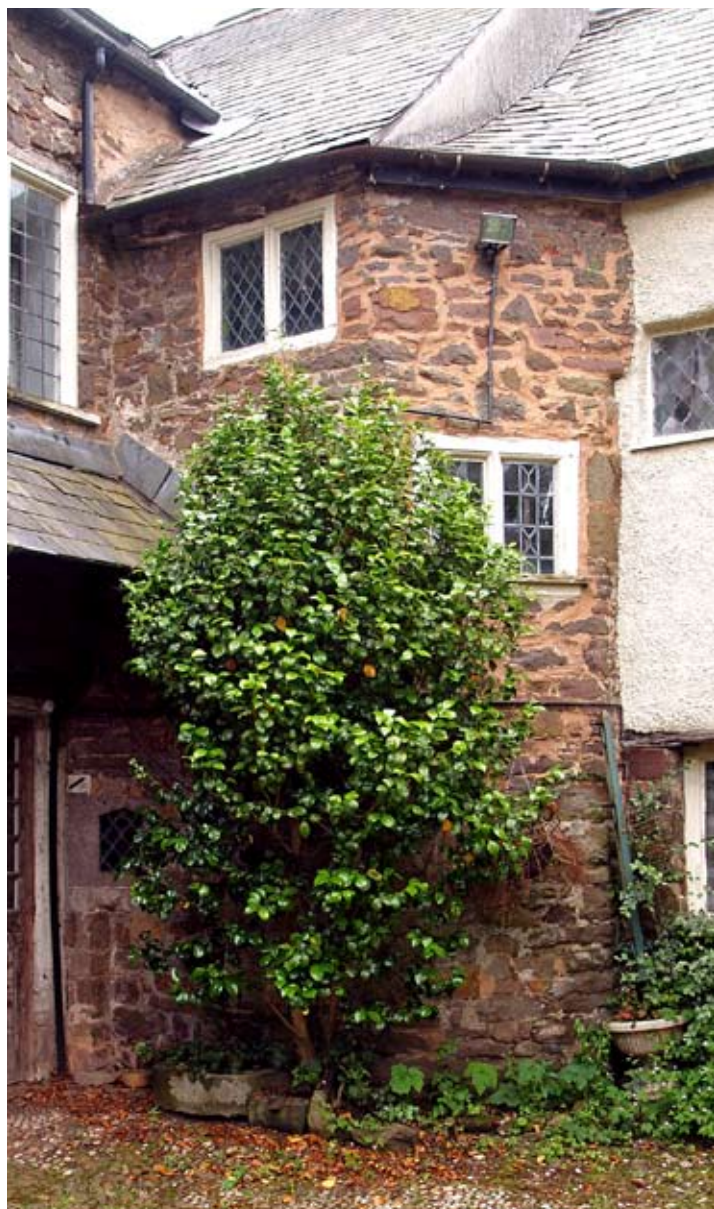
The service stair turret, 09.06.2009
