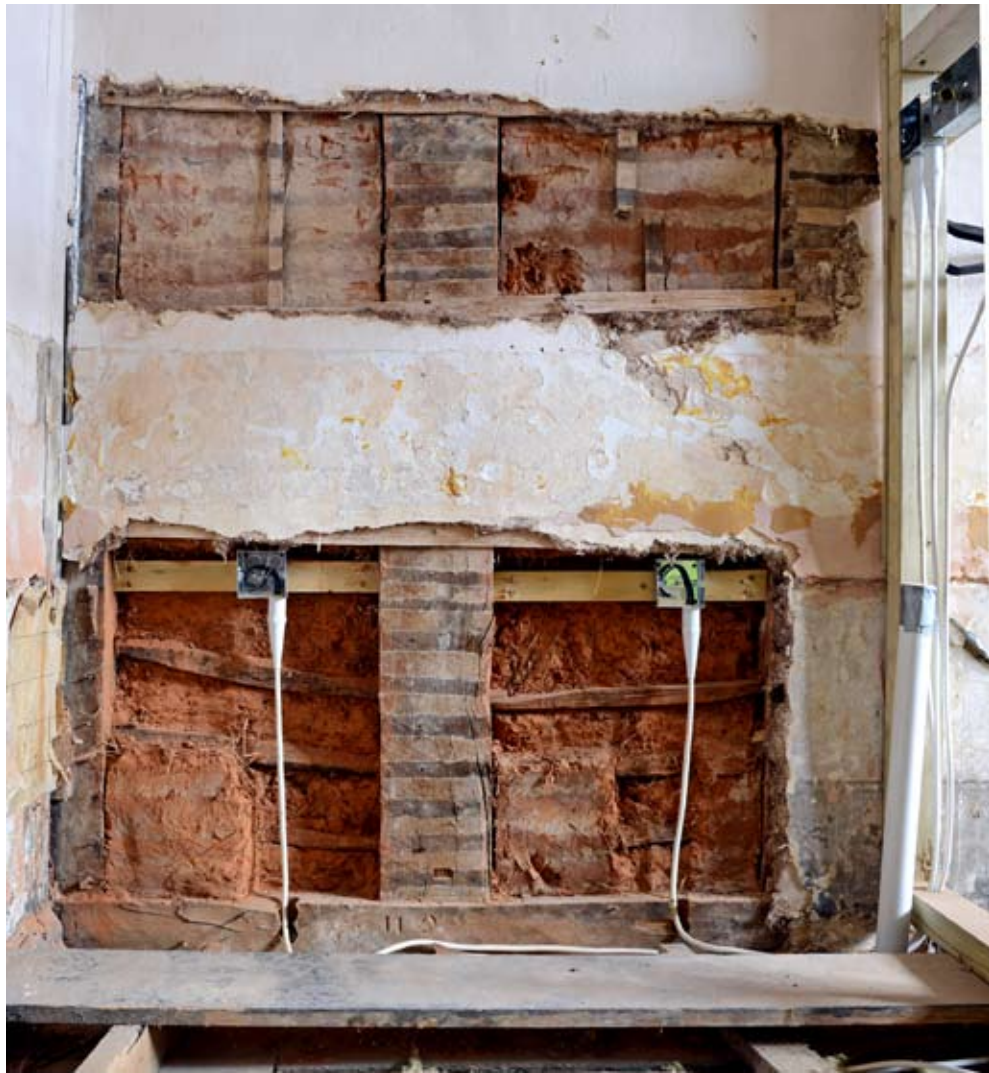
The east wall of the kitchen chamber backs onto the Great Chamber. It is close studded with rod-and-daub infill and clad with lath and plaster. Notice the chiselled assembly marks in the sill and the early 18th century painted black skirt to right, 18.06.2013.
