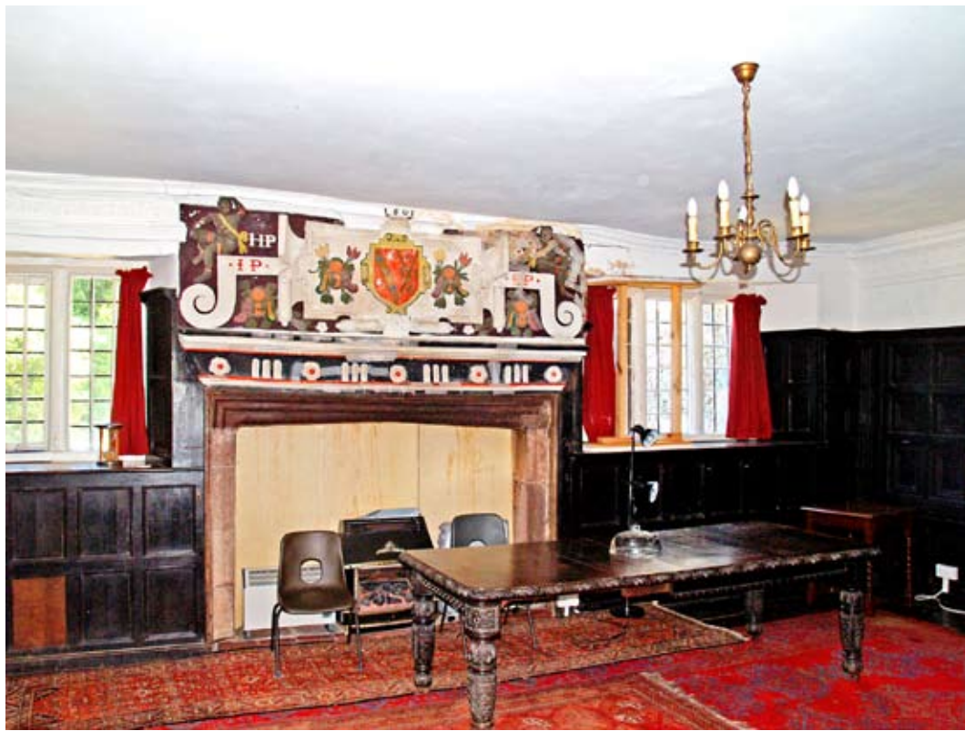
The west wall contains the fireplace and overmantle flanked by windows, 02.06.2009
