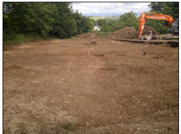
Figure 13: The site, post-excavation, from the west (scales 1&2m).
