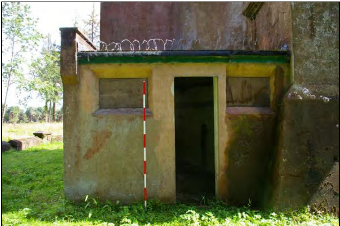
Figure 8: The concrete block service extension; from the west.
