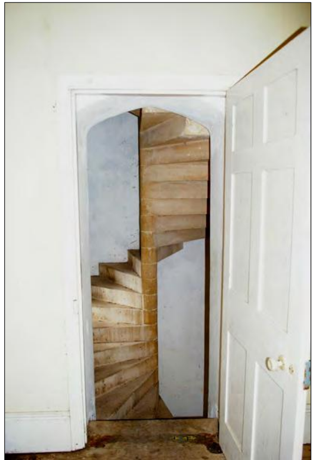
Figure 13: The first floor doorway to the stair, viewed from the east.
