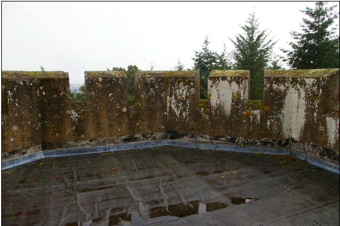
Figure 20: The flat roof and parapet of the tower, from the north-east.
