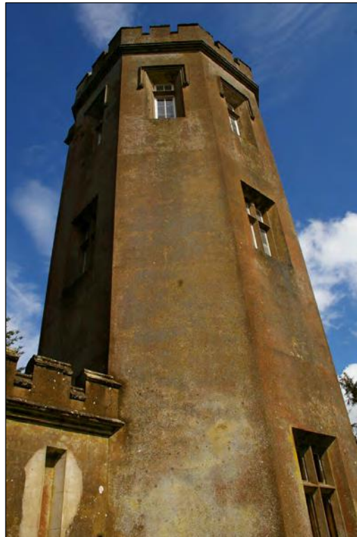
Figure 11: View up the south-west side of the tower.
