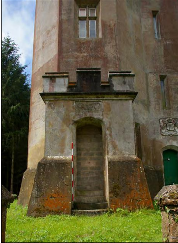
Figure 9: The main entrance porch, viewed from the east
