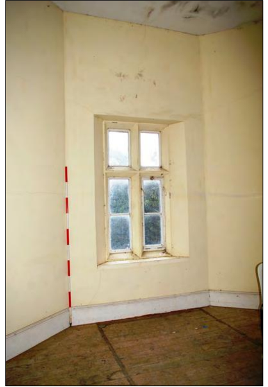
Figure 13: The east side of the second floor room, showing the mullion-and-transom windows; from the north-west.
