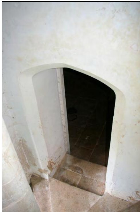
Figure 16 The door to the kitchen, from the north.
