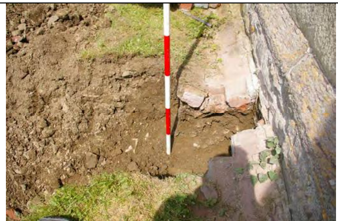
Photo 6: Brick drain at West end of church and trench. Looking North.
