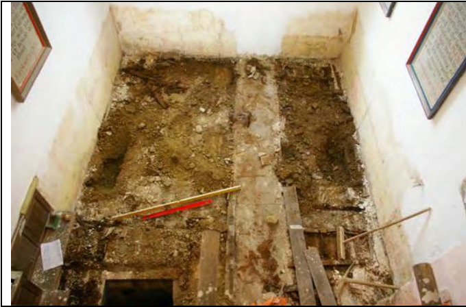
Photo 1: beneath the plank floor in the North transept. Looking North.
