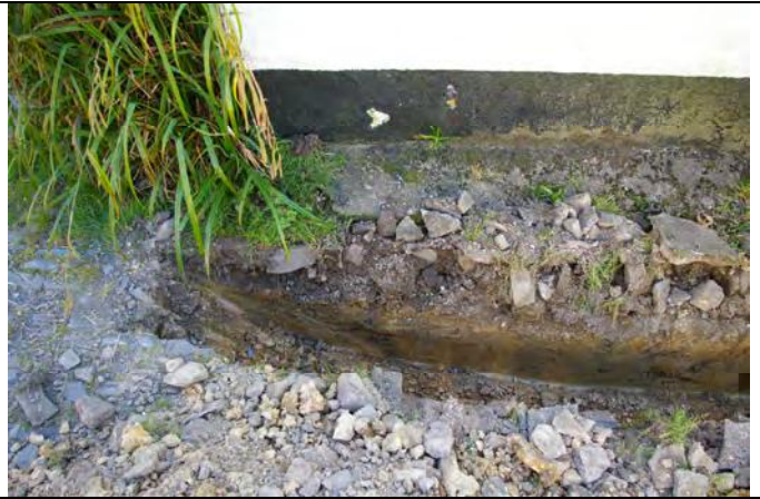
Photo 2: Section at East end of trench. Looking South.
