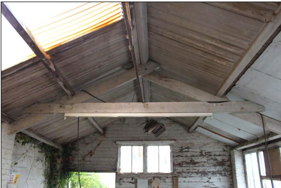
Figure 24: Roof structure of Building 5, viewed from the south.
