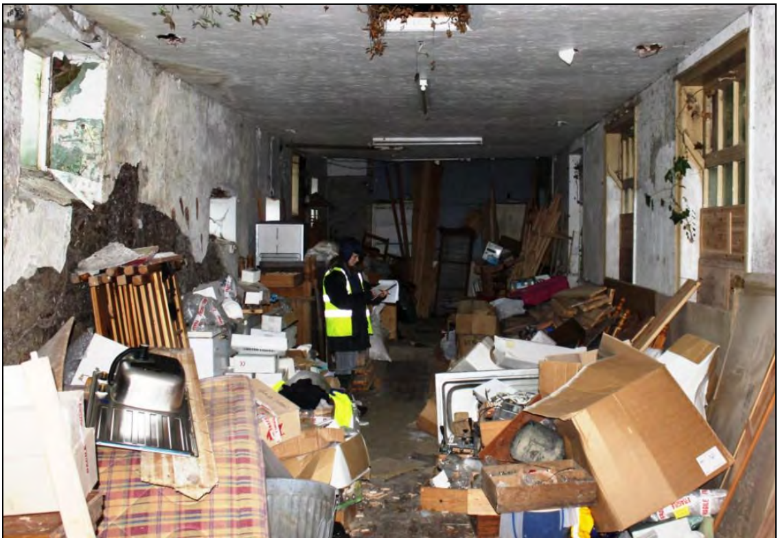
Figure 20: Inside Building 3, viewed from the north.
