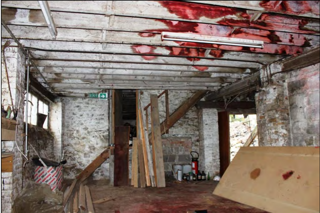
Figure 23: Main ground floor area of Building 5, viewed from the northeast.
