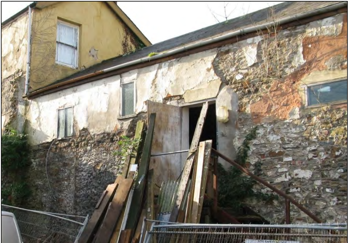
Figure 19: East elevation of Building 3, viewed from the north-west.
