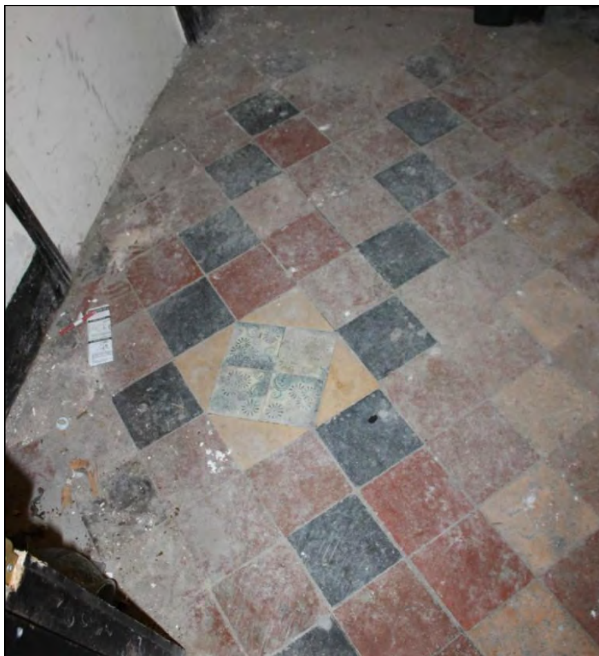
Figure 31: Quarry tile floor in stair hall of Building 7, viewed from the north-east.
