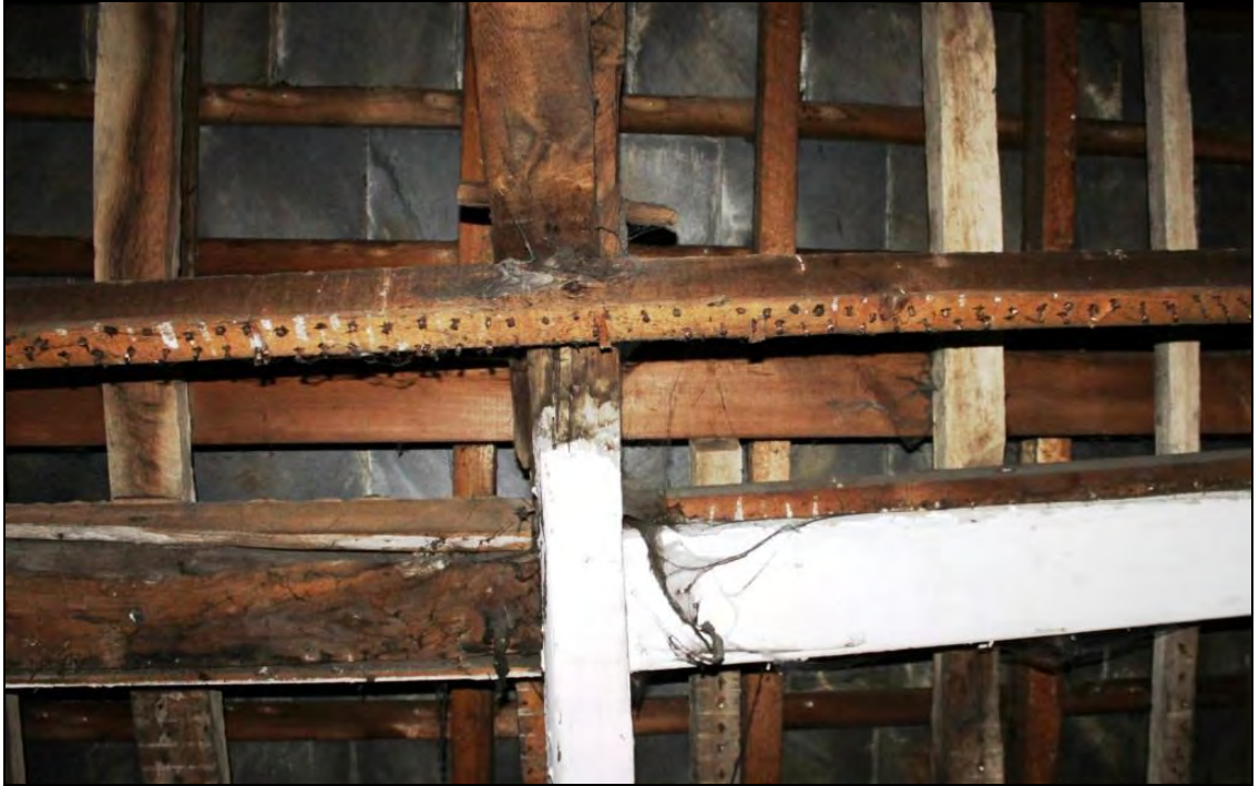
Figure 17: Detail of roof.
