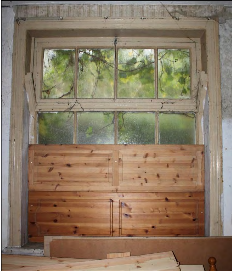
Figure 21: Example of the windows within the west wall of Building 3.
