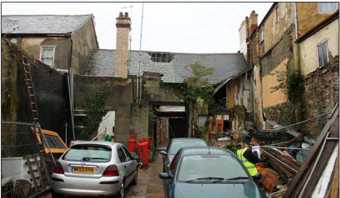
Figure 10: Rear elevation of Building 1, viewed from the north.
