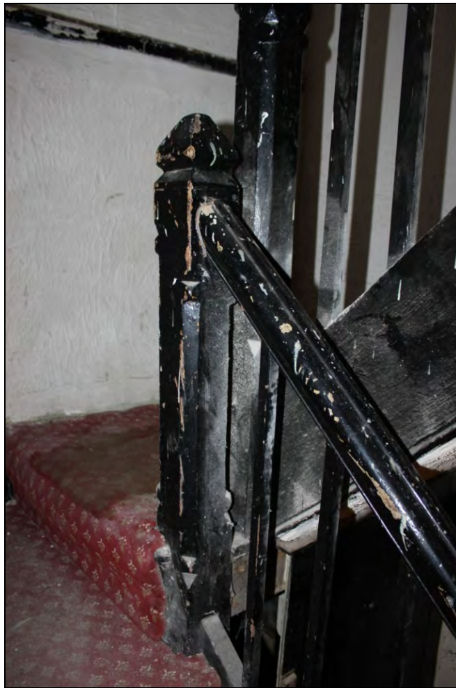
Figure 32: Detail of stair to Building 7, viewed from the east.
