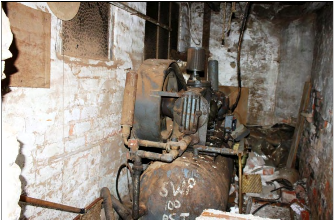
Figure 25: Engine Room and engine at south end of Building 6, viewed from the west.
