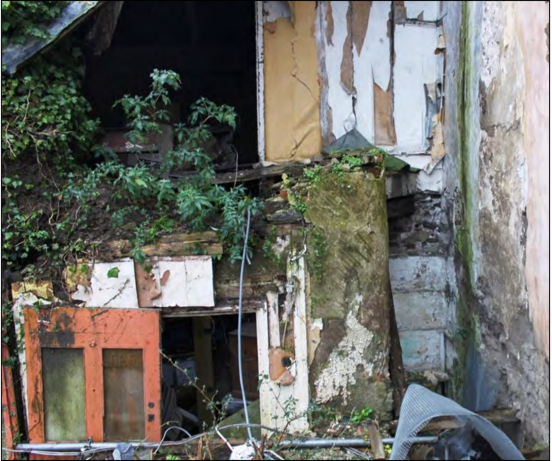
Figure 18: External shot of Room 1 and former stair, viewed from the north (inside Building 2).
