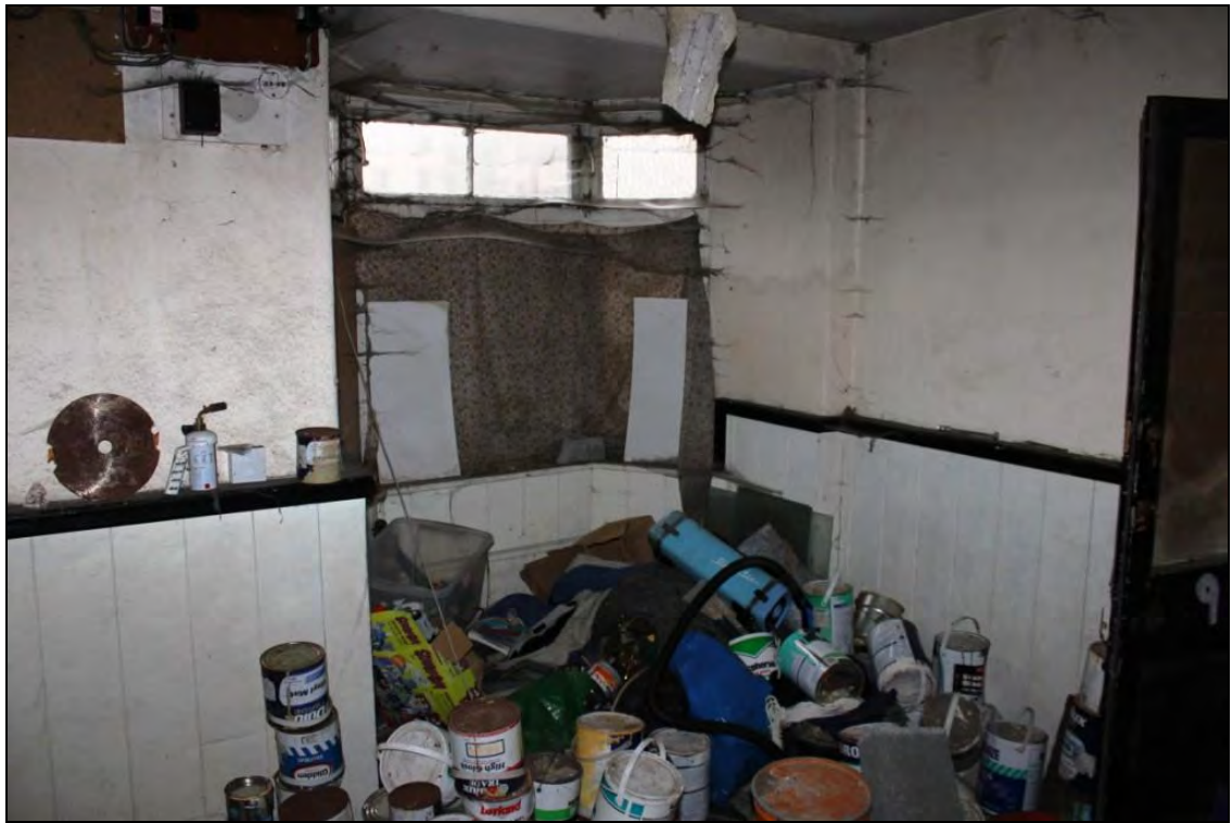
Figure 13: Bay window in Room 2, viewed from the northeast.
