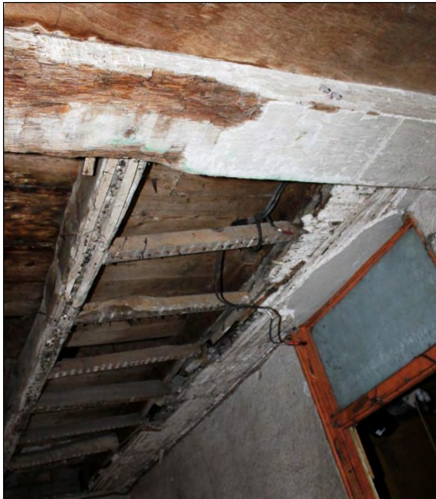
Figure 11: Ceiling above central passageway in Building 1, from the northwest.
