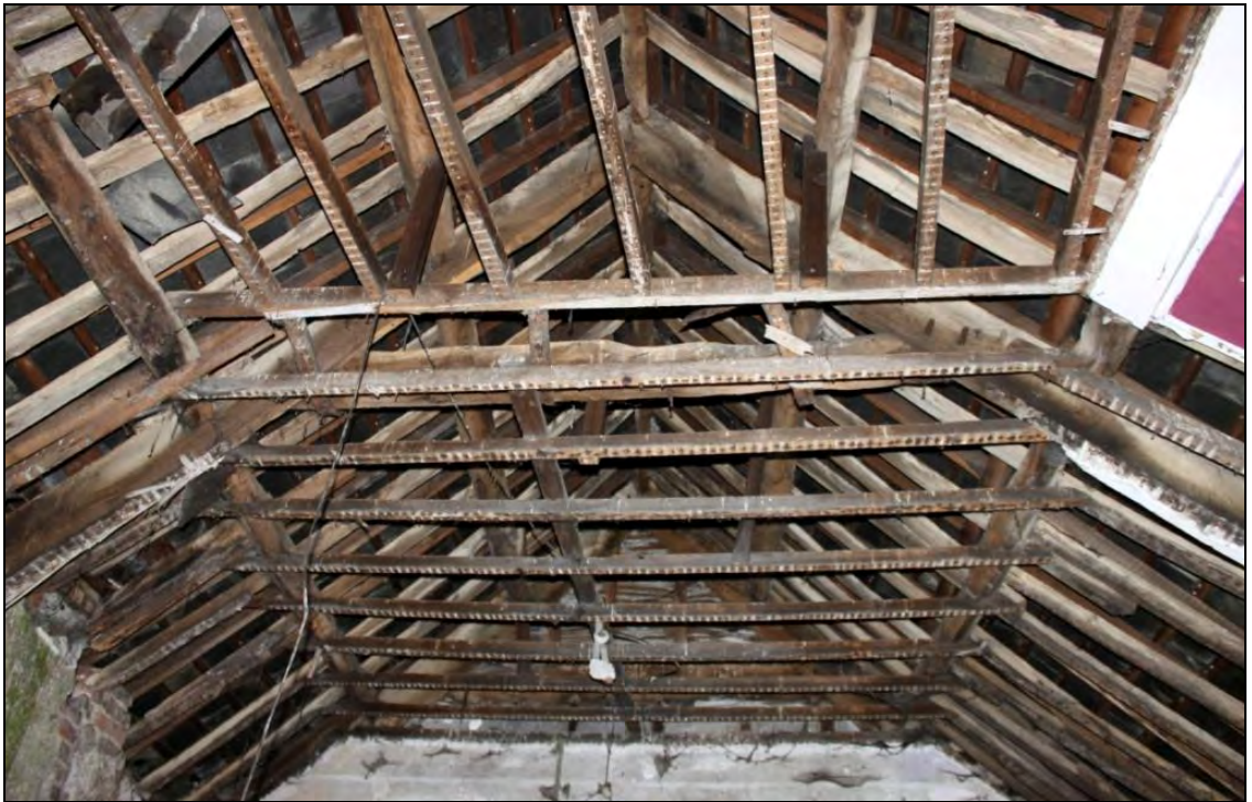
Figure 16: 17 th Century roof structure of Building 1, viewed from the west.
