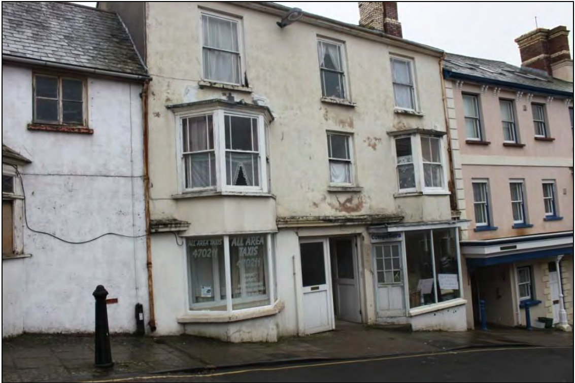
Figure 27: Street frontage (south facing elevation) of Building 7, viewed from the southwest.
