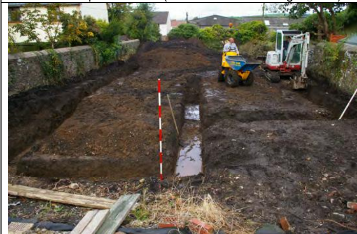
Photo 7: Middle Footings Trench aligned N-S.
