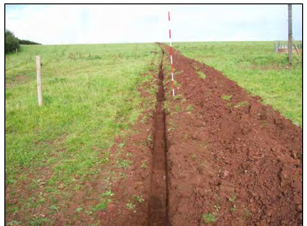
Photo 4: N Cable Trench SW end, Post-Excavation, looking NE (scale 2m).
