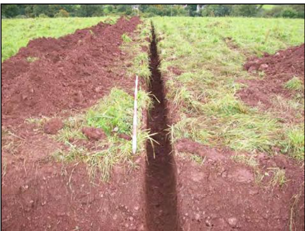
Photo 3: Cable Trench NE end, Post-Excavation, looking SW (scale 2m).
