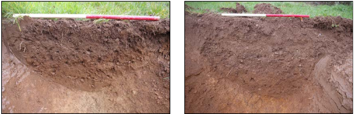
Figure 5: Left – Sample section 1, viewed from south-west (1m scale). Right – Sample section 2, viewed from the north (1m scale). For locations of the sections see Figures 11. 13.4, 13.5.
