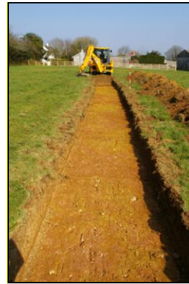
Figure 11: Trench #2 post-excitation, looking north (2m scale).
