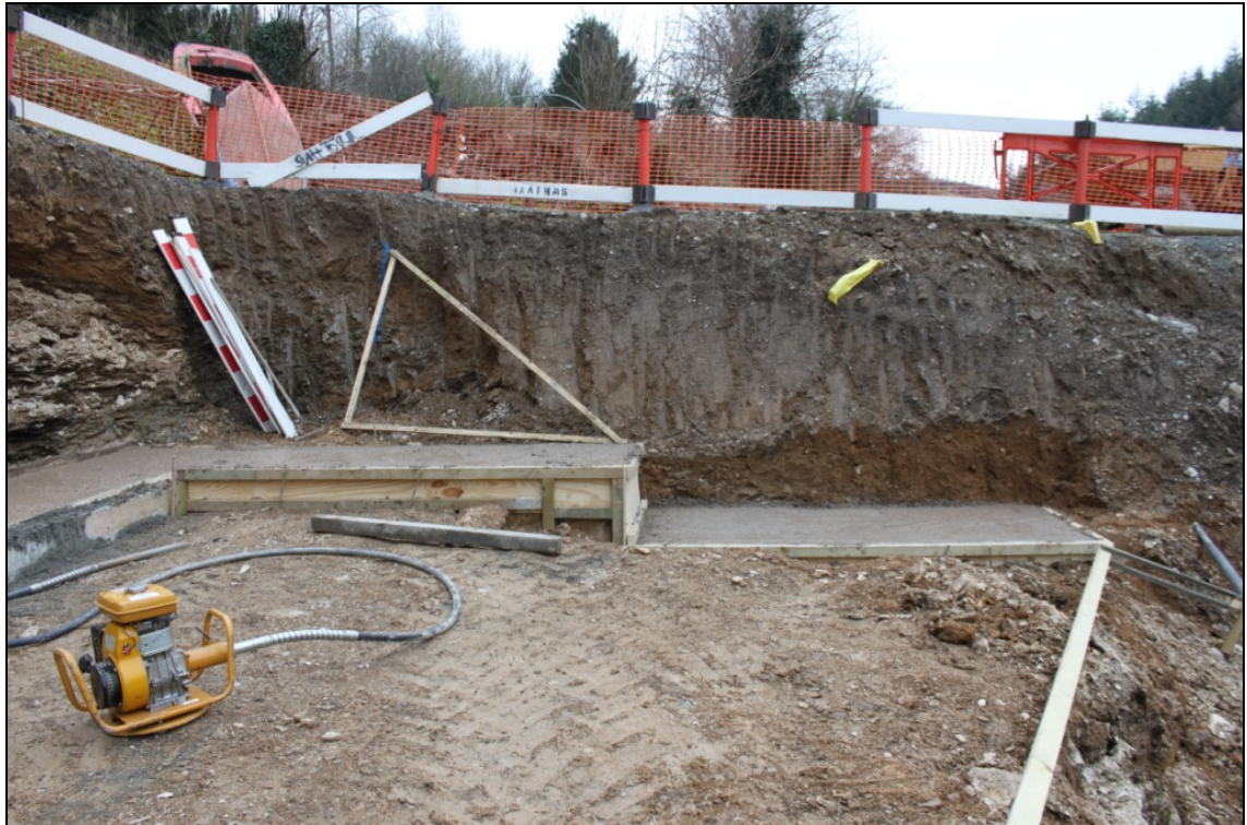
Figure 4: The south-western corner of development area, emphasising the depth for footings compared to existing ground level, viewed from the east (no scale).
