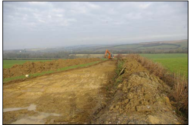
Figure 9: South end of access road post-excitation, looking north-west (no scale).
