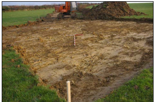
Figure 13: Turbine base post-excavation, looking south-east (1&2m scale).
