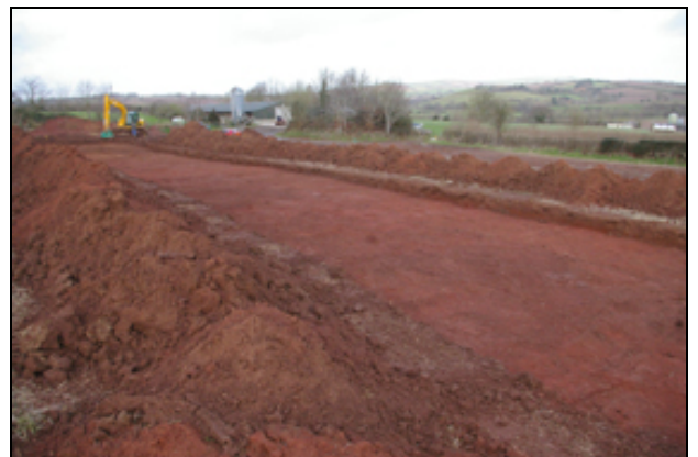
Photo 6: The site, post excavation, looking north-east.
