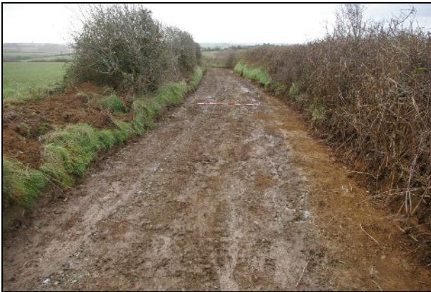
Figure 16: Existing track-way post maintenance, looking south (2m scale).
