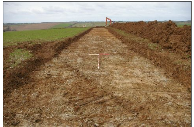
Figure 17: Post-Excavation of access track, looking west (1&2m scale).
