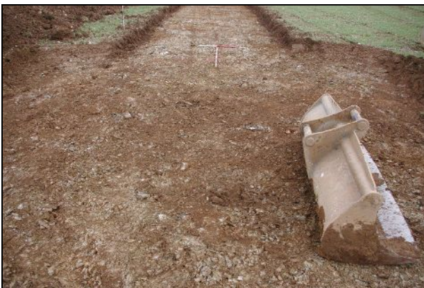
Figure 18: Post-Excavation of turbine base, looking east (1&2m scale).
