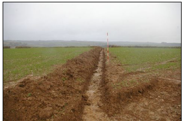
Figure 19: Post-Excavation of cable trench, looking north-west (1&2m scale).
