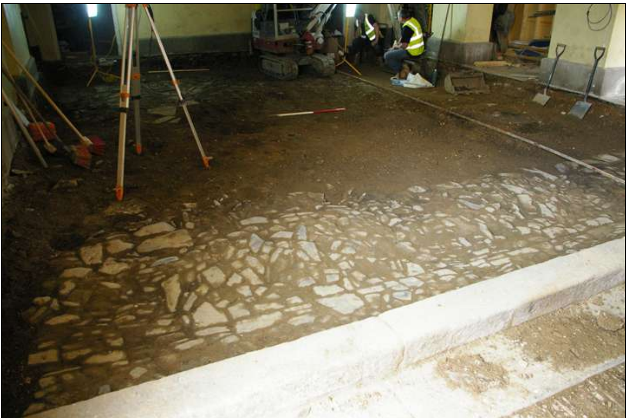
Site shot mid-excavation showing Posthole [17] and Cobbled Floors (108) and (109); viewed from the north-west (1m scale).
