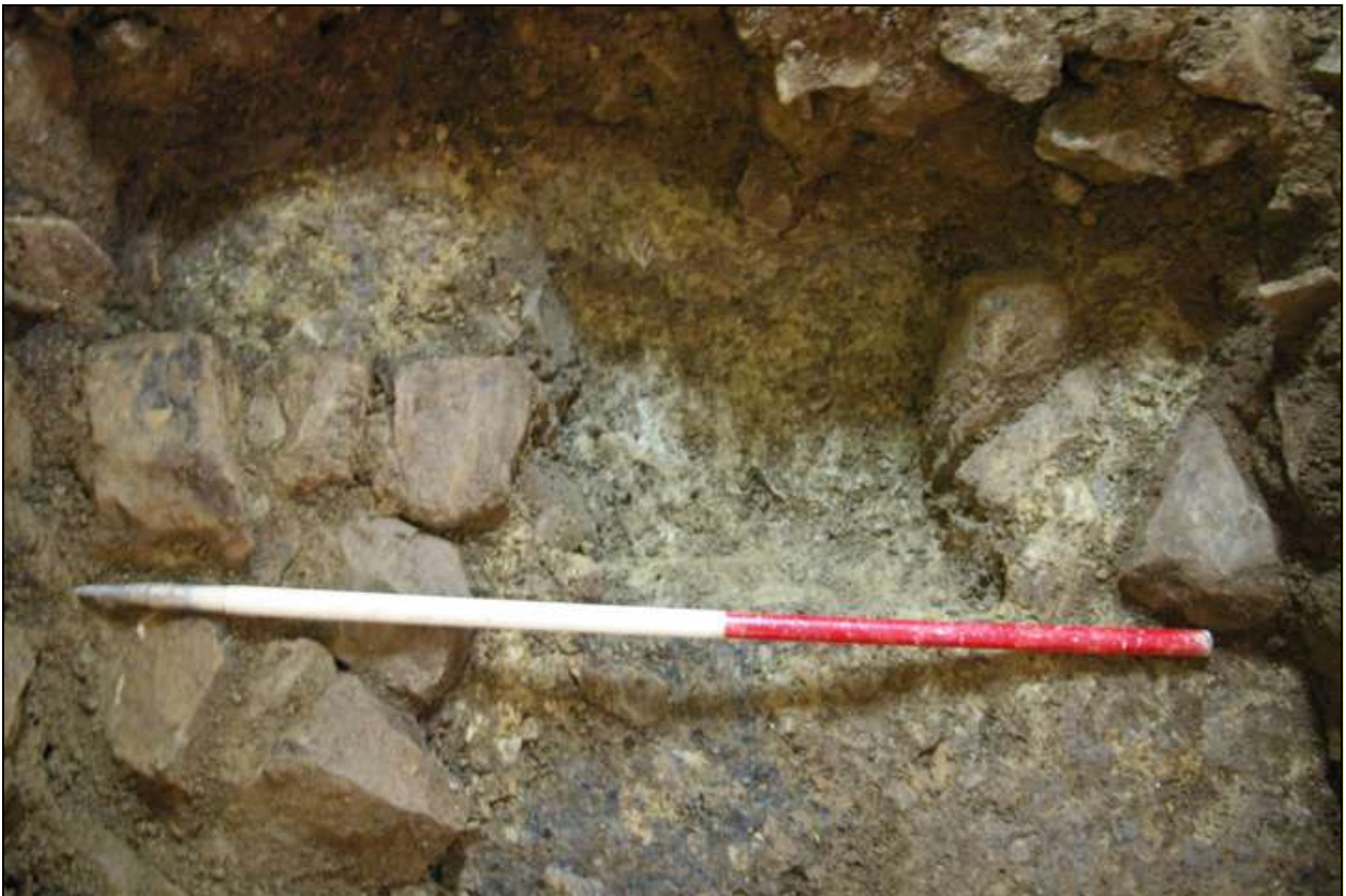
Wall {126} and Foundation Cut [124]; viewed from the west and above (1m scale).
