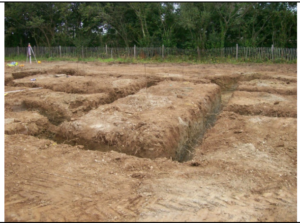
Figure 2: Post-ex footings trench for plot 4, viewed from the south-west (no scale).
