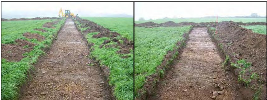
Figure 13: Left: Trench 1, post excavation, viewed from southeast; Right: Trench 2, post excavation, viewed from the southwest (2m scale).
