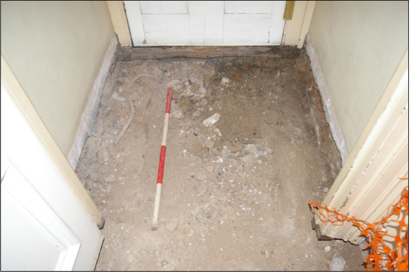
Figure 2: Shot of the lobby showing the water pipe and lines of footings, from the northwest with flash (1m scale).
