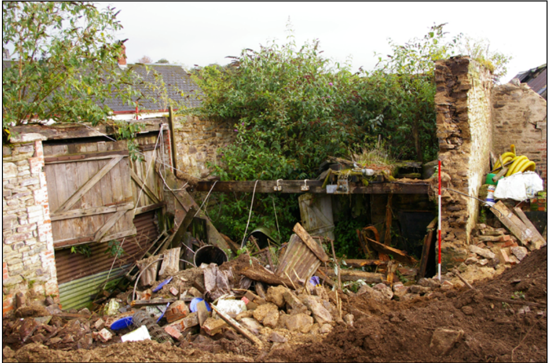
Figure 13: The north -east, east and south walls of building 4, viewed from the south-west.
