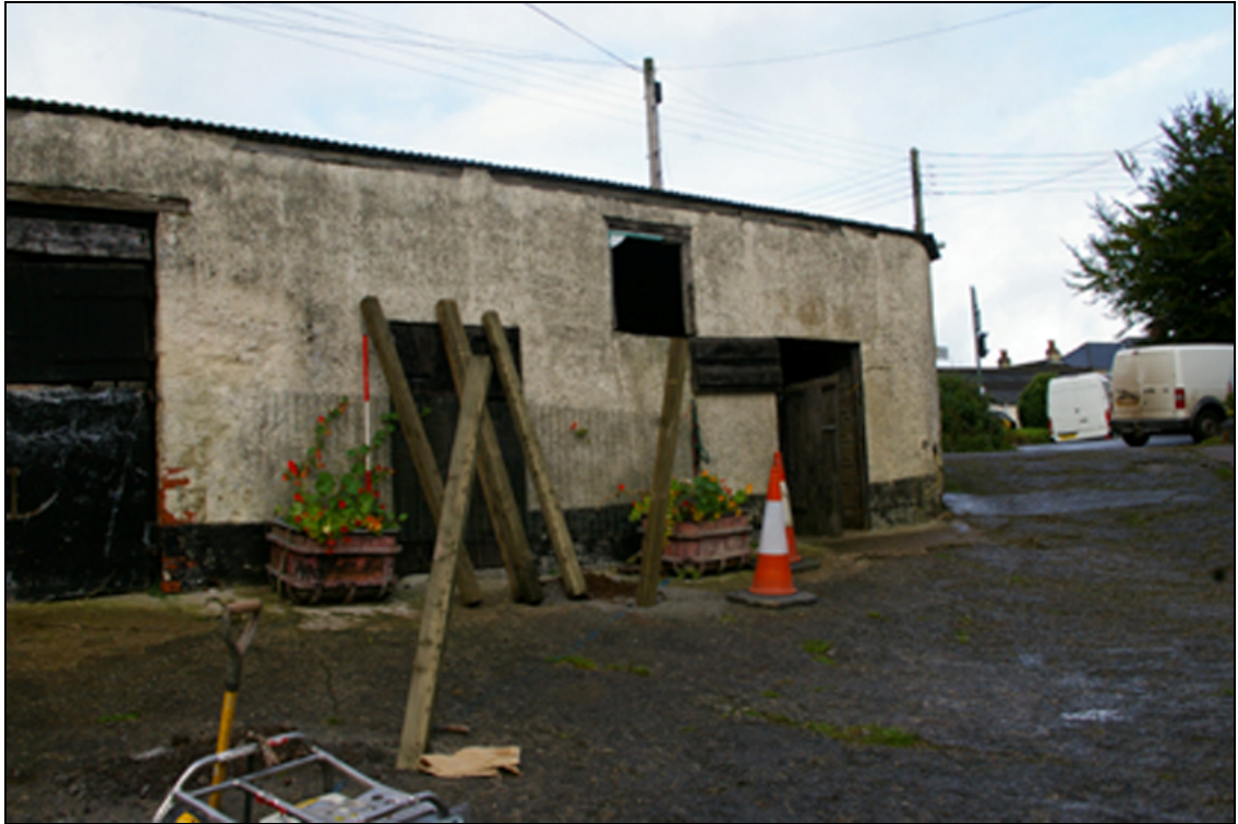
Figure 5: The Exterior east wall of Building 2, viewed from the south-east.
