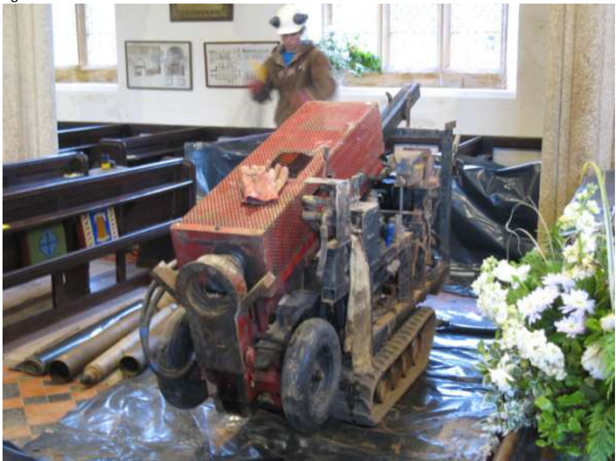
Figure 6: As above, work starts on Borehole #2.
