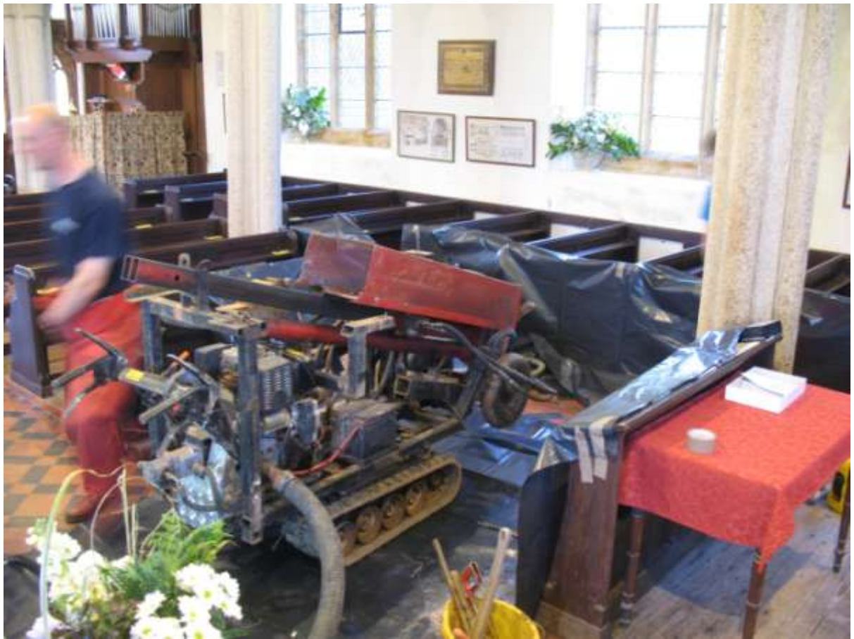
Figure 1: View of the mini-corer, before work starts on Borehole #1.
