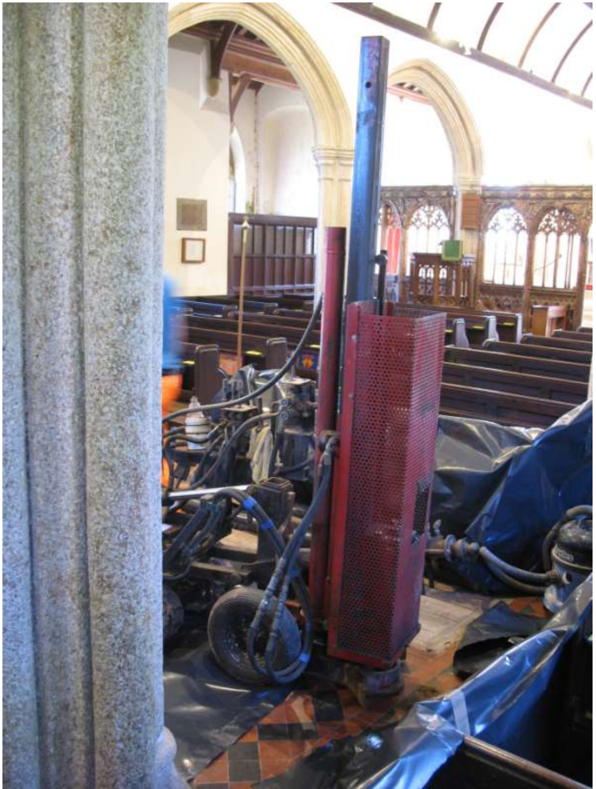
Figure 2: As above, as work begins.
