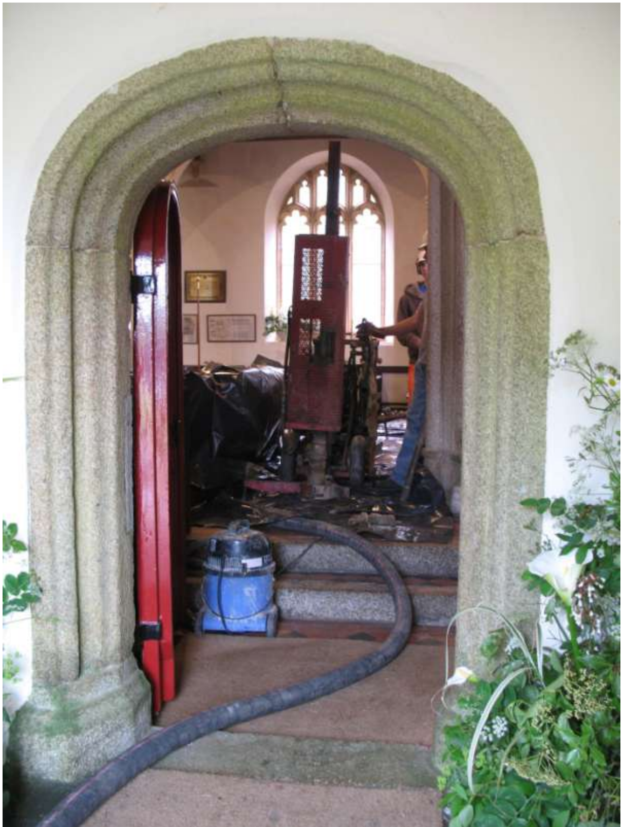
Figure 7: View through the church door as work commences on Borehole #3.
