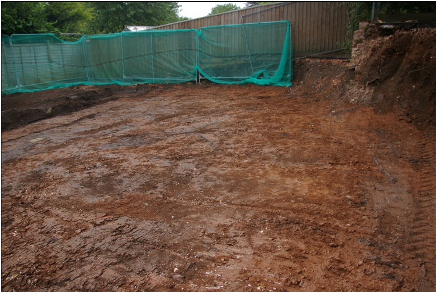
Figure 3: The stripped development area, viewed from the northeast.
