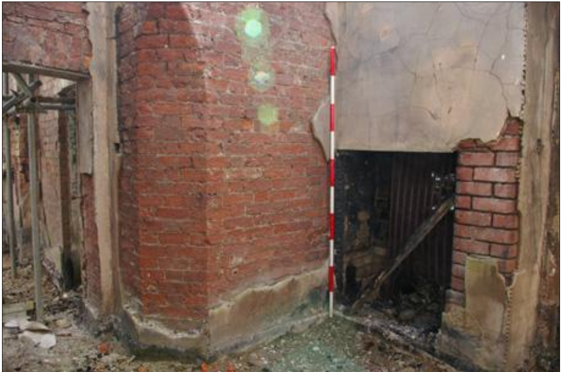
Figure 11: The south-west corner of the kitchen (R2), with brick built fireplace (for a range), viewed from the north-east (2m scale).
