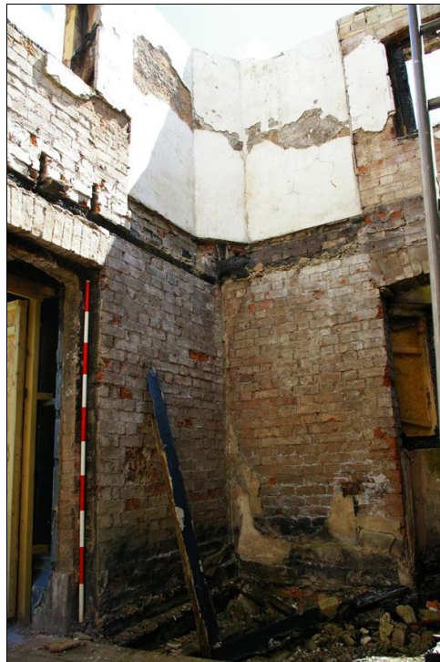
Figure 10: The north-east corner of R1, with the projecting wall sections and in-filled corners at first floor level, viewed from the south-west (2m scale).
