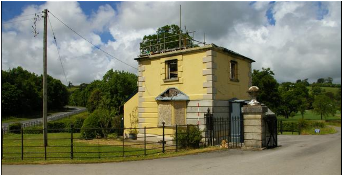
Figure 3: The exterior south and east elevations of the Lodge, viewed from the south-east (2m scale).
