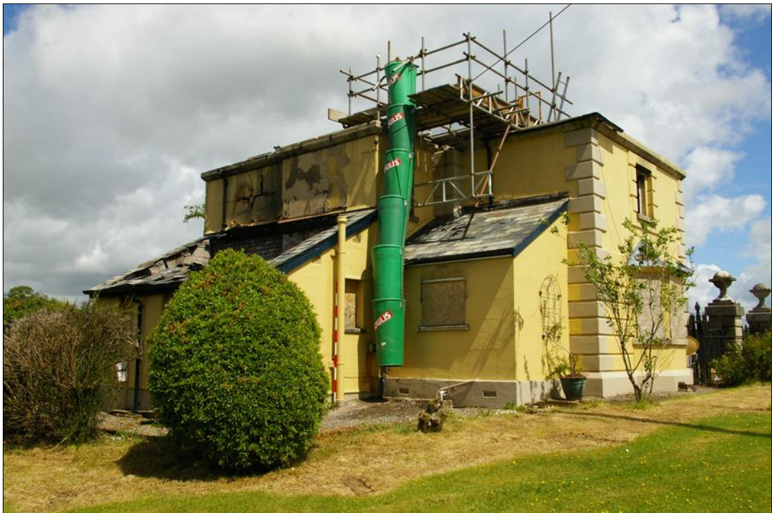
Figure 7: The south and west exterior elevations of the Lodge, viewed from the south-west (2m scale).
