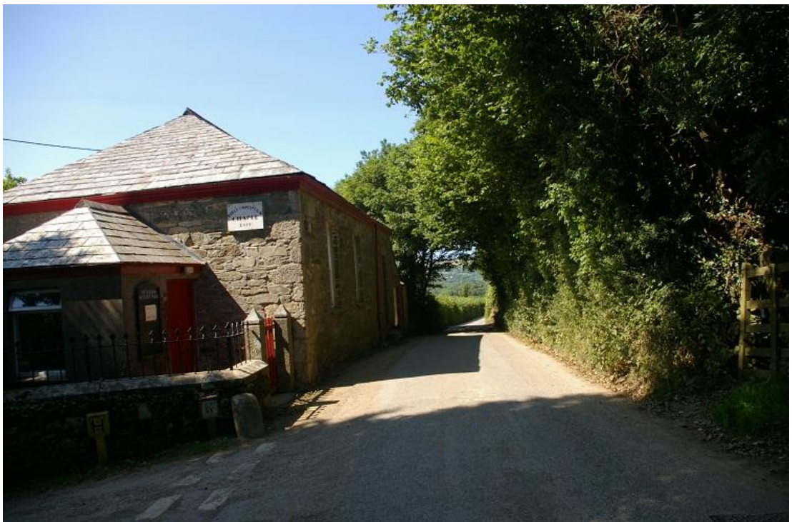
Treveighan Methodist Chapel, on high ground alongside a parish road, with wide views to the surrounding area but limited by its heavily wooded grounds; from the south-east.
