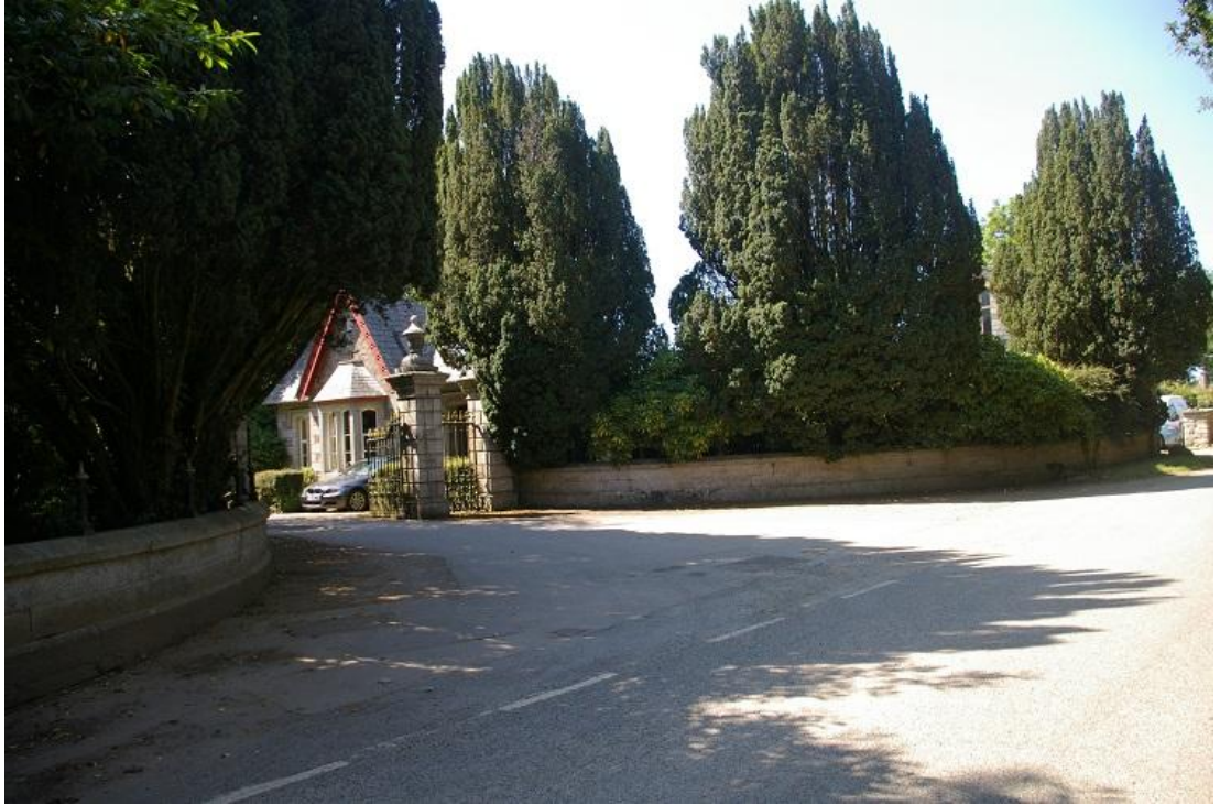
View of gatepiers, walls and lodge to Michaelstow Manor, showing blocking from specimen trees, planted in the grounds; from the east.
