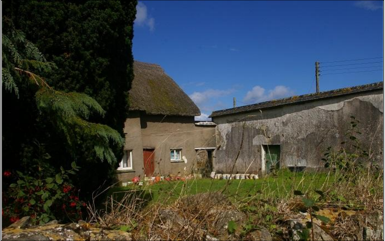
Pixton Farm, with its gardens walls and adjacent buildings; viewed from the south-west.
