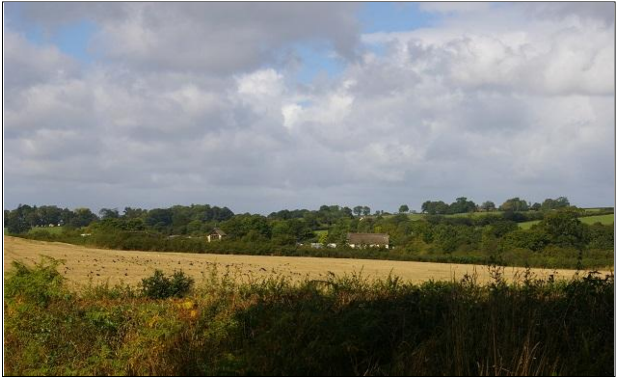
Burrow Farm, a Grade II* listed farmhouse outside Monkokehampton; viewed from the south-east.
