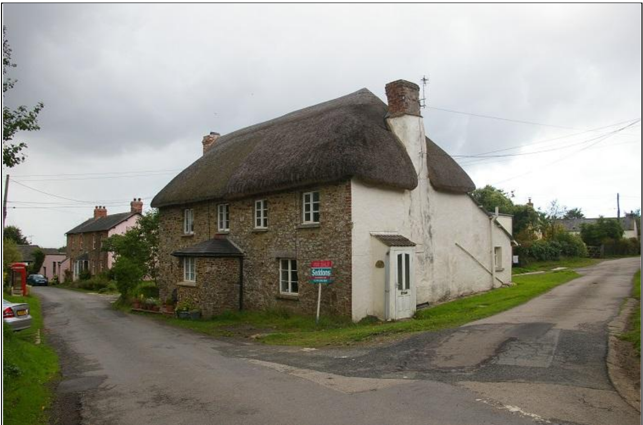
The listed cottages in Broadwoodkelly; viewed from the south-east.
