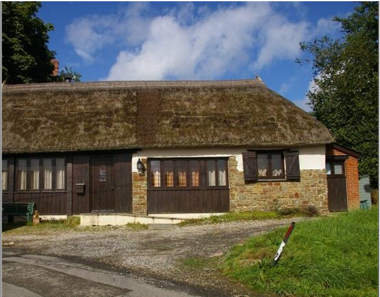
Listed outbuilding in Iddesleigh viewed from the south.
