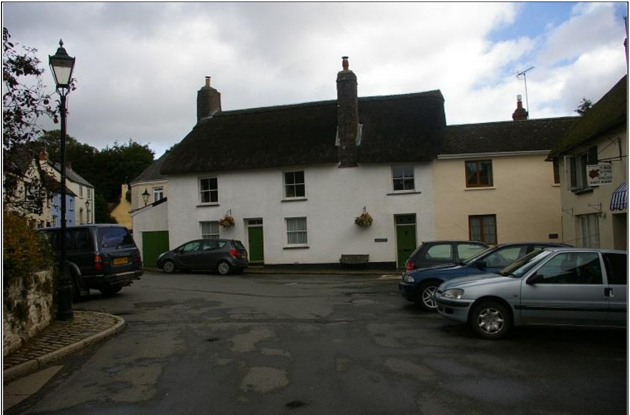
Bank House, in Winkleigh and the butcher's shop to the right hand side; viewed from the west.
