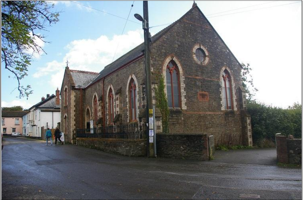
Methodist Chapel in Winkleigh; viewed from the south-west.
