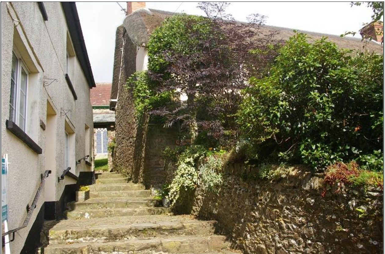
The church steps and Church House; viewed from the south.
