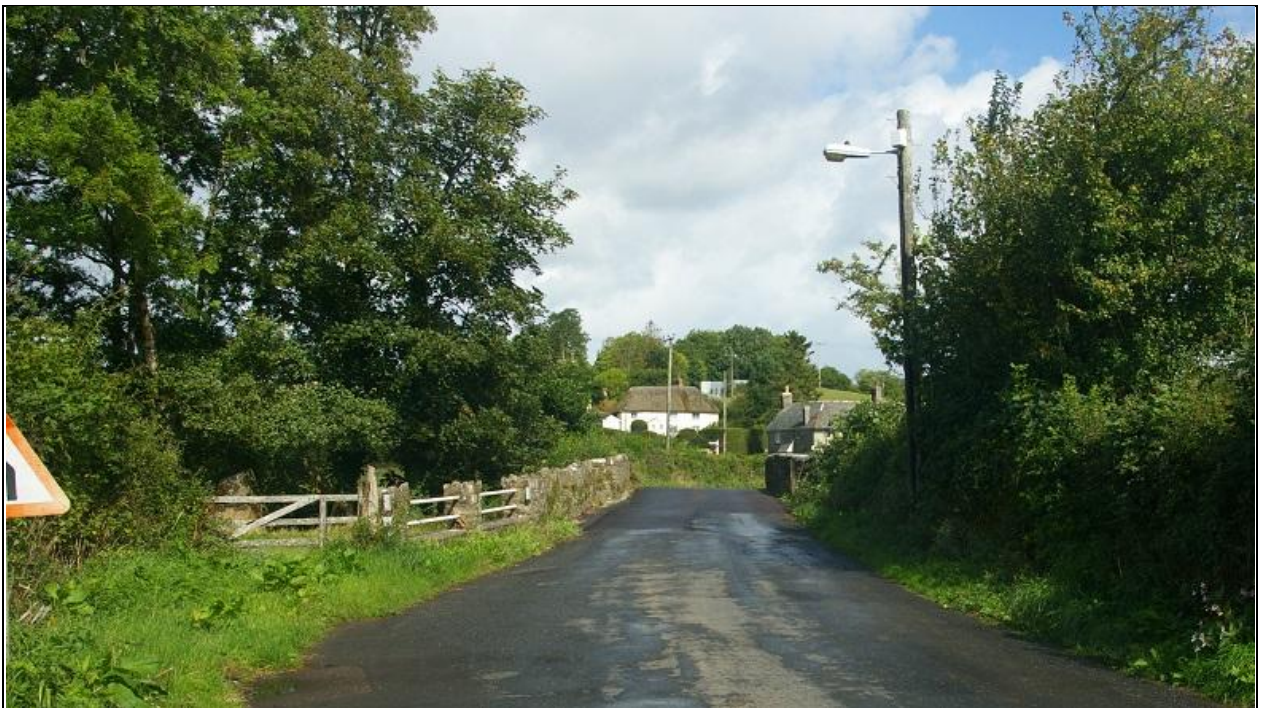
Shilley Bridge, north of Monkokehampton; viewed from the south.
