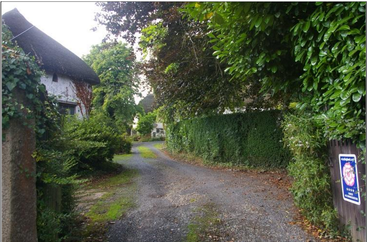
Parsonage Court and associated thatched outbuildings; viewed from the east.
