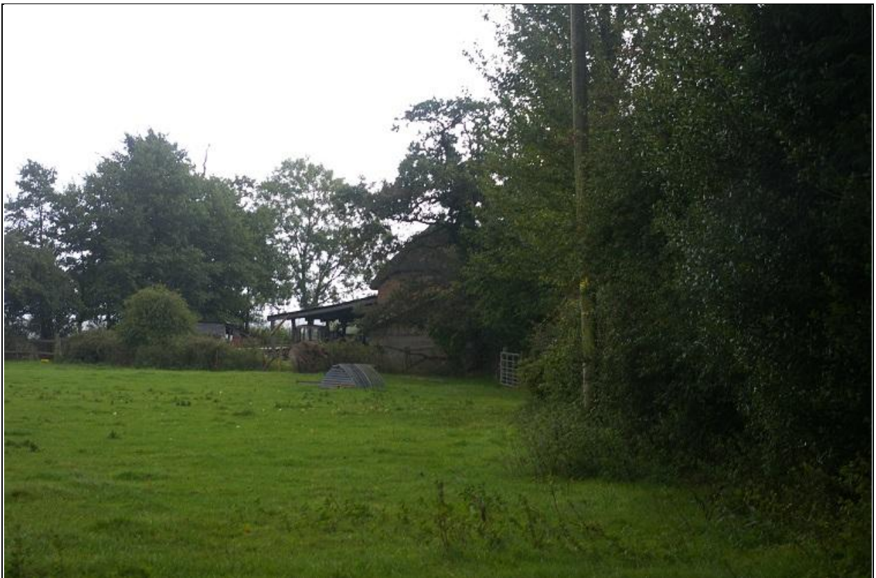
The outbuilding at BullHead Farm, with thatched roof; viewed from the north.
