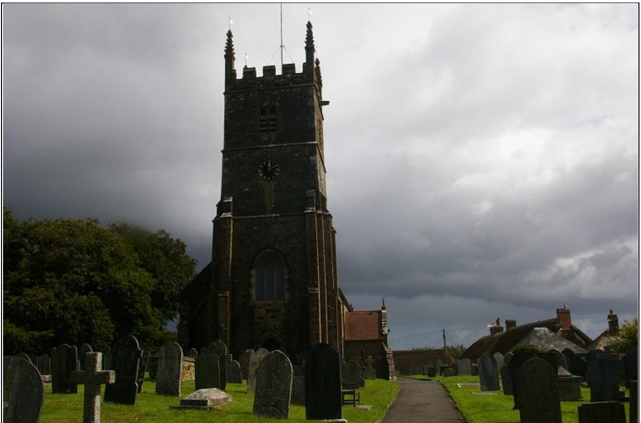
The church in Winkleigh, Church of All Saints; viewed from the west.
