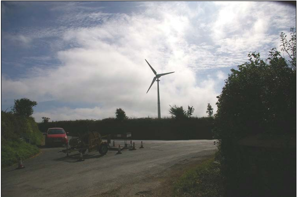
View of the wind turbine which stands just outside St Maybn, facing the track which leads down to Tregarden, a Grade II* listed farm; form the south-west.
