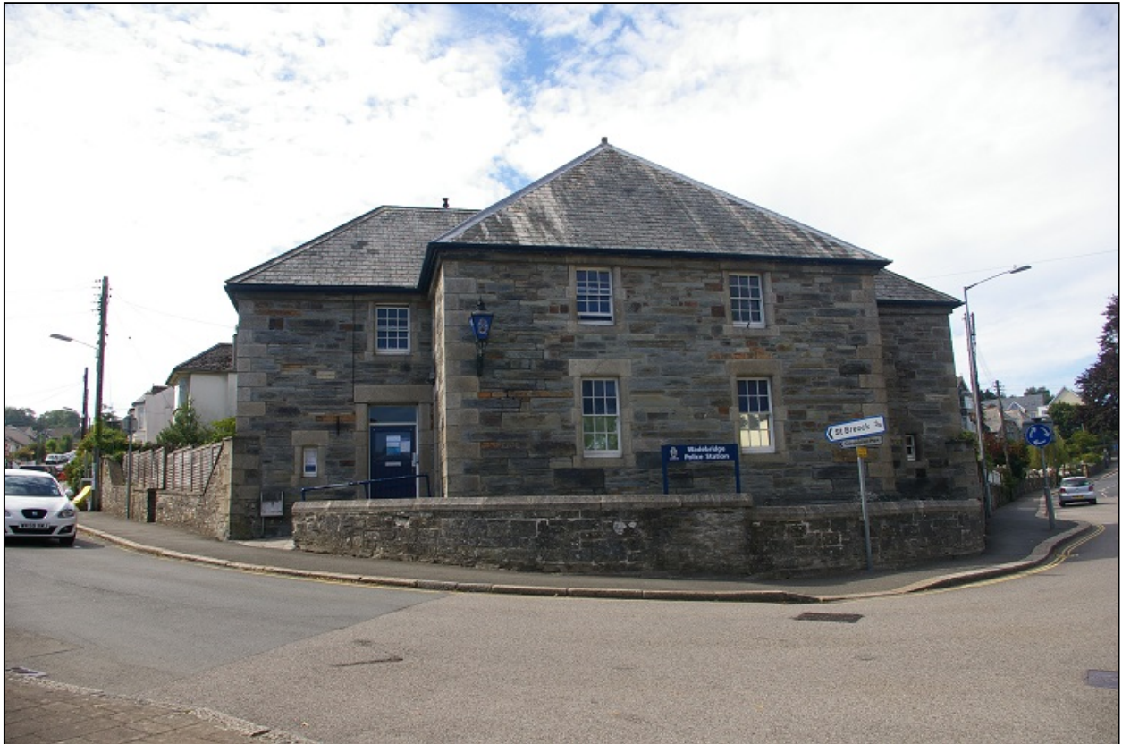
View of Wadebridge Police Station, a Grade II listed building; from the north
