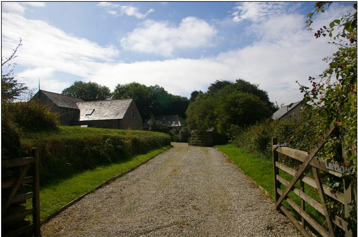
View to Pengelly Farm, set in a wooded enclosure beyond its historic stone farm buildings; from the south.
