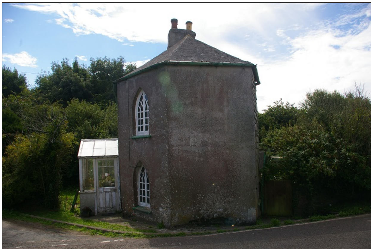
The small toll house, formerly on the old coach route over the high downs; from the north-west.
