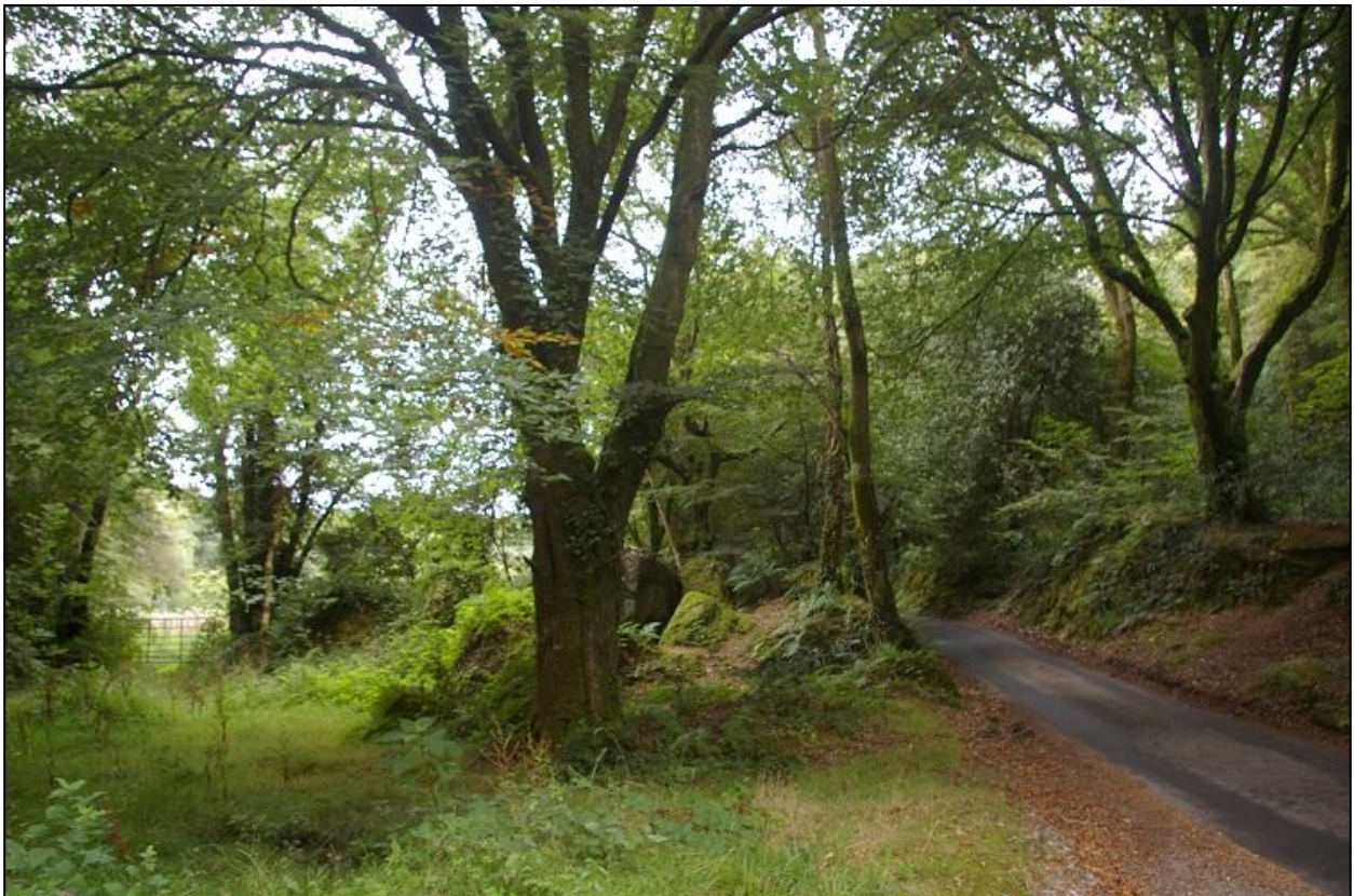
Views within the Luxulyan valley, a protected mining landscape, showing the thick tree coverage; from the south.
