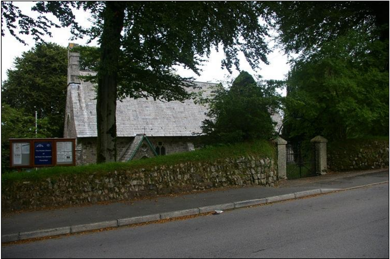
The small 19 th century church of St Peter, showing it surrounded by trees; with no views out to the surrounding countryside; from the south.
