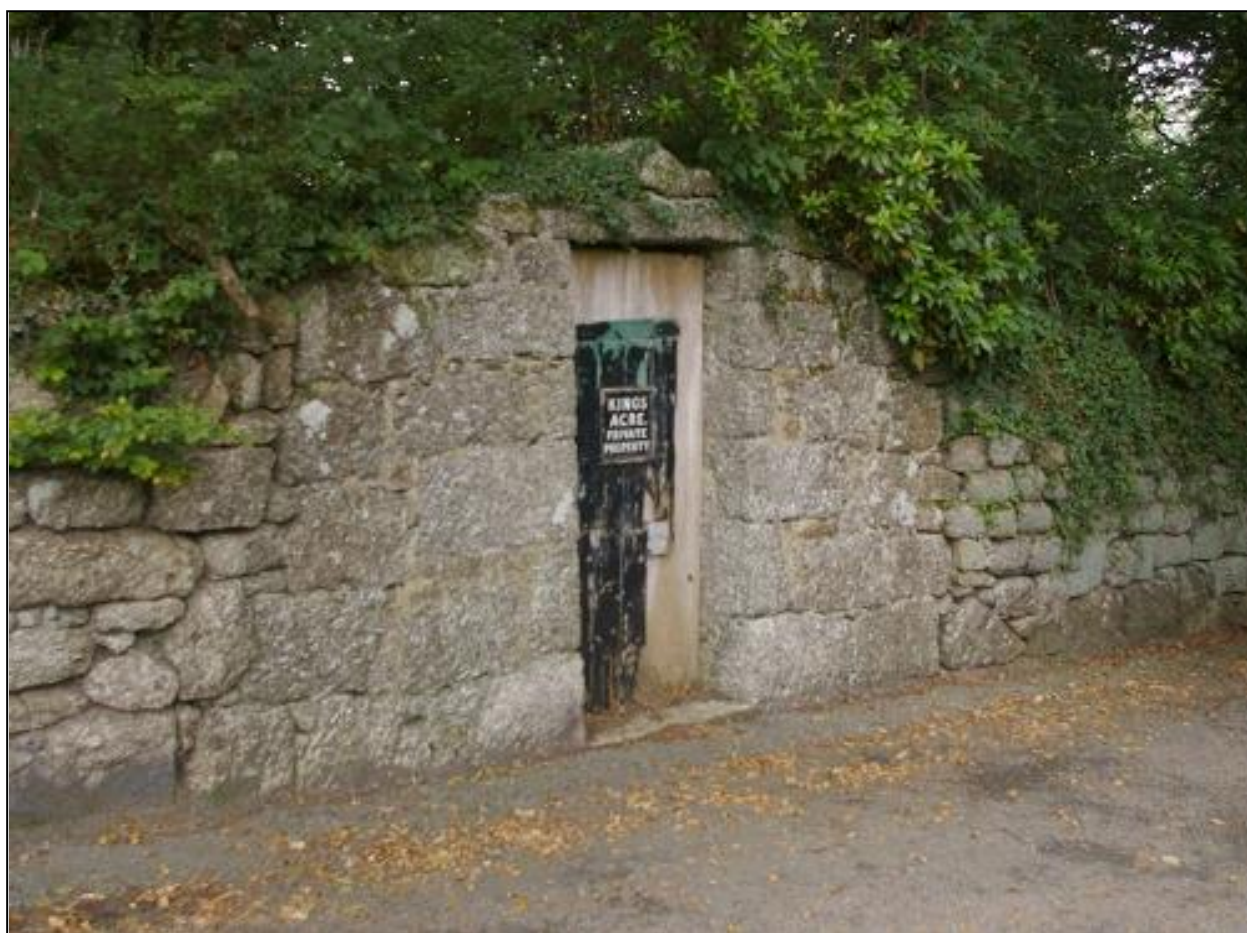
The Listed gateway into Kings Acre, opposite the church; from the south-west.
