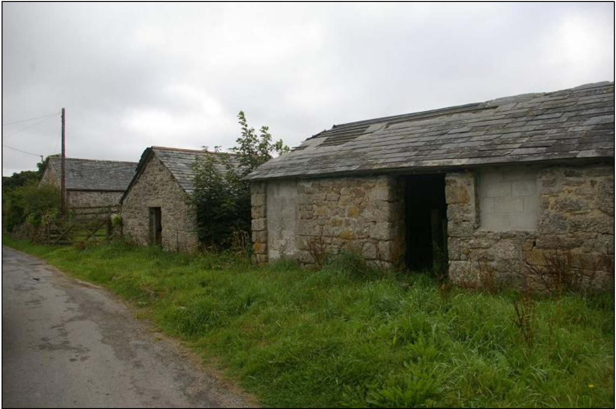
The barns and stables of the Old Farmhouse, in Bodwen, all Grade II listed buildings; from the north-east.
