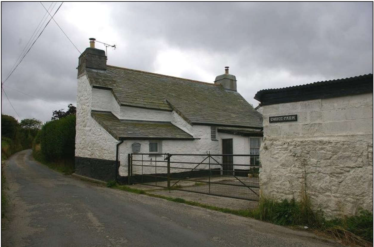
Conce Farmhouse, on the side of the road, showing its low roof height and the tall hedges to its garden at the front; from the north-east.
