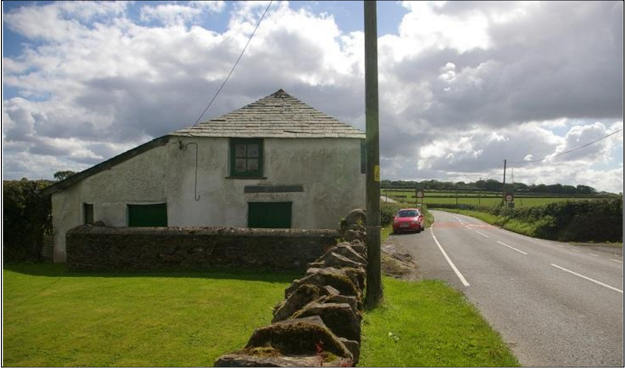
The Bible Christian Chapel and its views across the road to the south-west, towards the proposed turbine; from the north.
